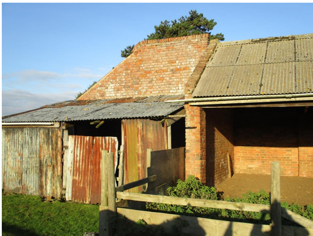
Photo 5: Corrugated-iron lean-to at south-western corner of the building.
