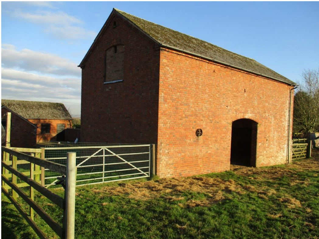
Photo 22: Brick-built barn to south-east of cow house.
