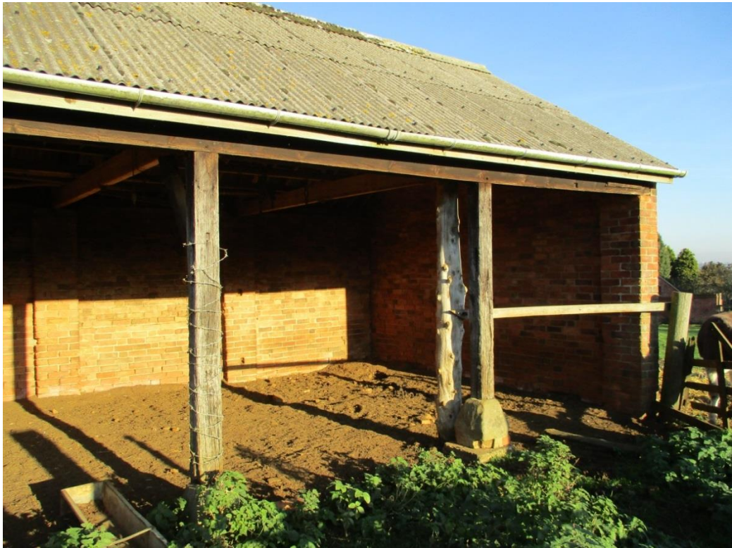
Photo 6: Room 2, cow shelter. Later asbestos roofing.
