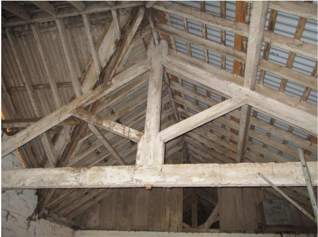
Photo 21: Roof-structure over room 6.
