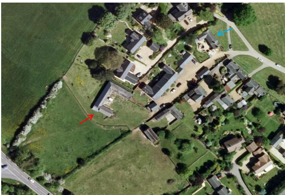
Aerial photo 1: Aerial view with the building at left (red arrow), and College Farm farmhouse (blue arrow). Comparison with the 1885 OS map (Fig. 3) confirms the extent of later infilling between the two. The paddock to the building's south-west is also part of the earlier farm.
