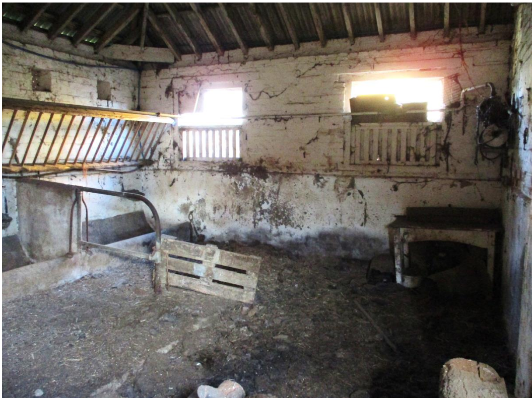
Photo 18: Room 6, the milking parlour.
