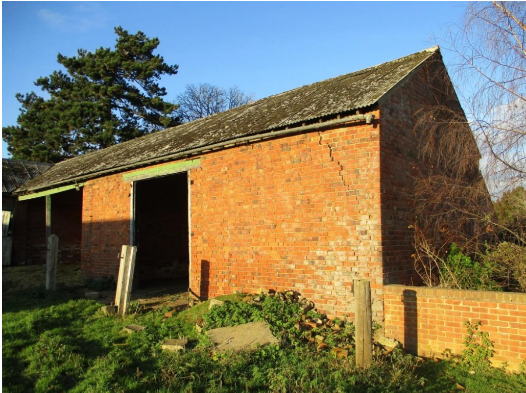
Photo 13: Cow shelter (room 7), and room 8 (right). Asbestos roof.
