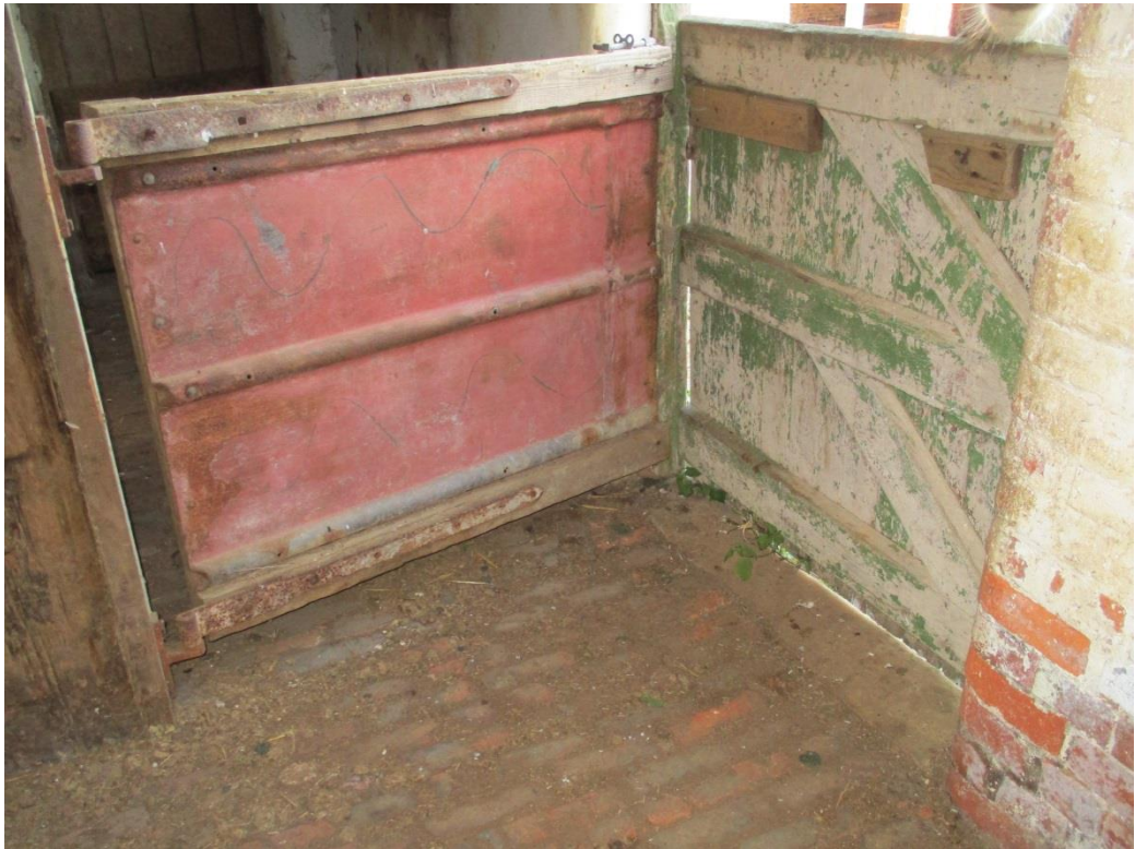
Photo 11: Stable doors in central range, and brick-flooring. Note the rounded edge to the brick-walling at right.
