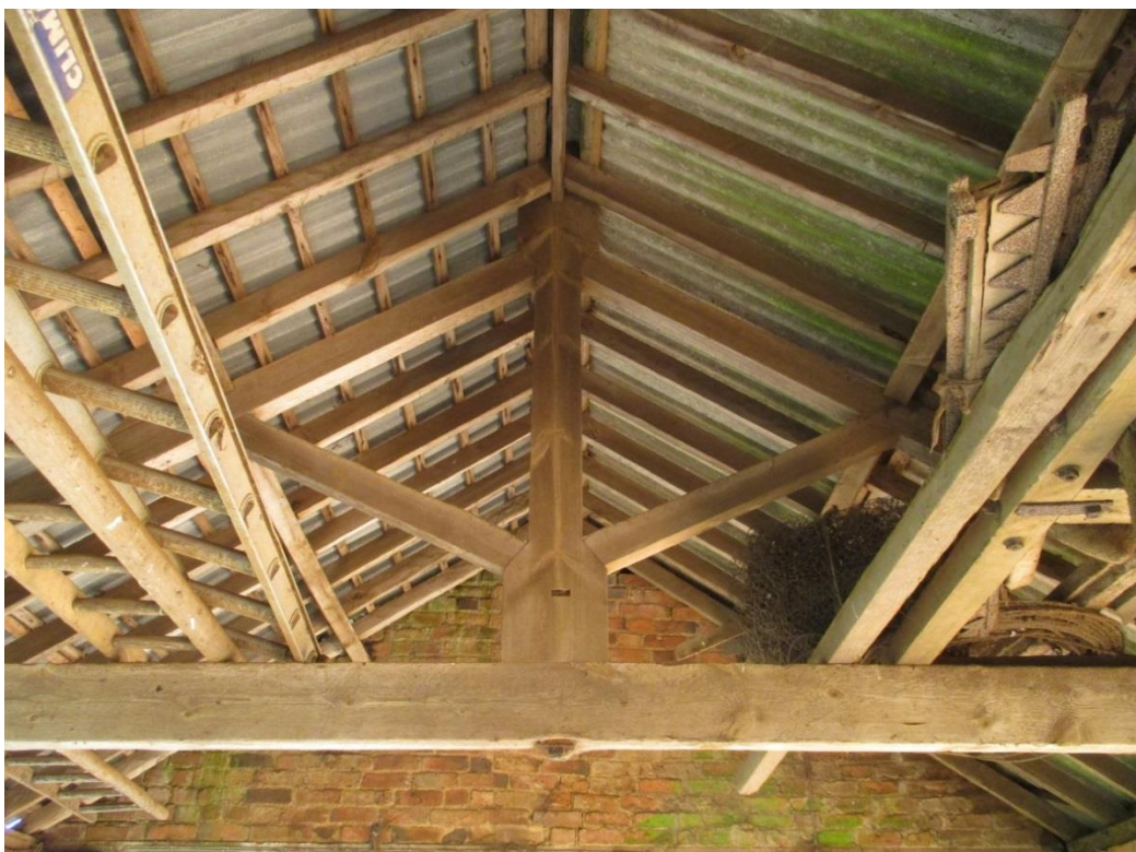
Photo 7: Roof structure to room 2. This appears more recent in date.
