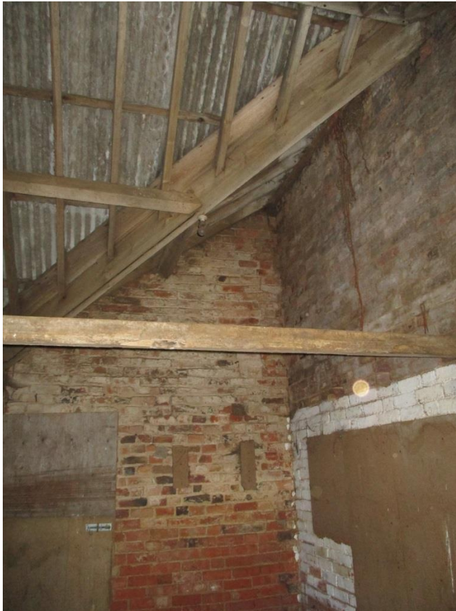
Photo 9: Roof intersection in room 2.
