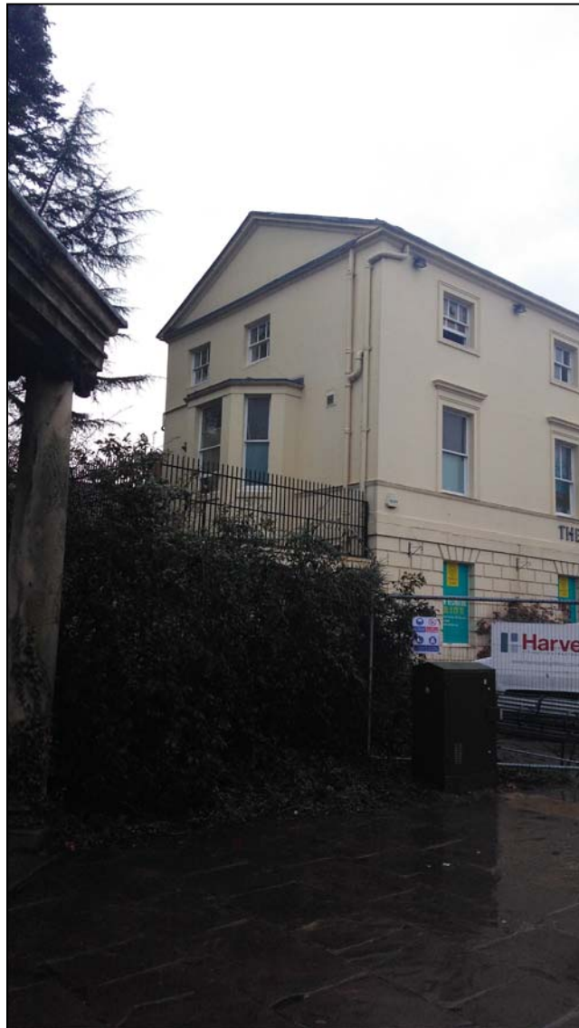
The south-west end of the building, from Friary
