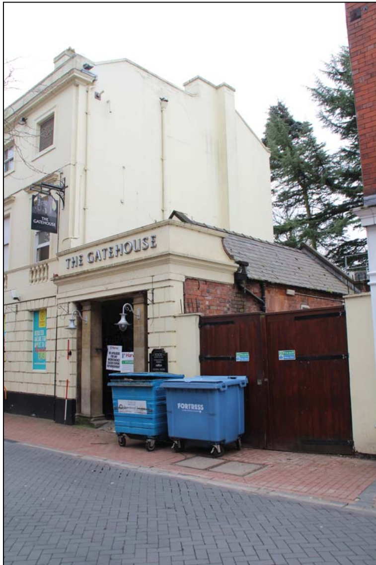
The north-west end of the building from Bird Street (scale 2m)
