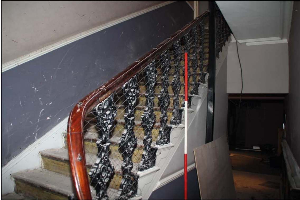
The ground floor flight of the stair ST1 (scale 2m)
