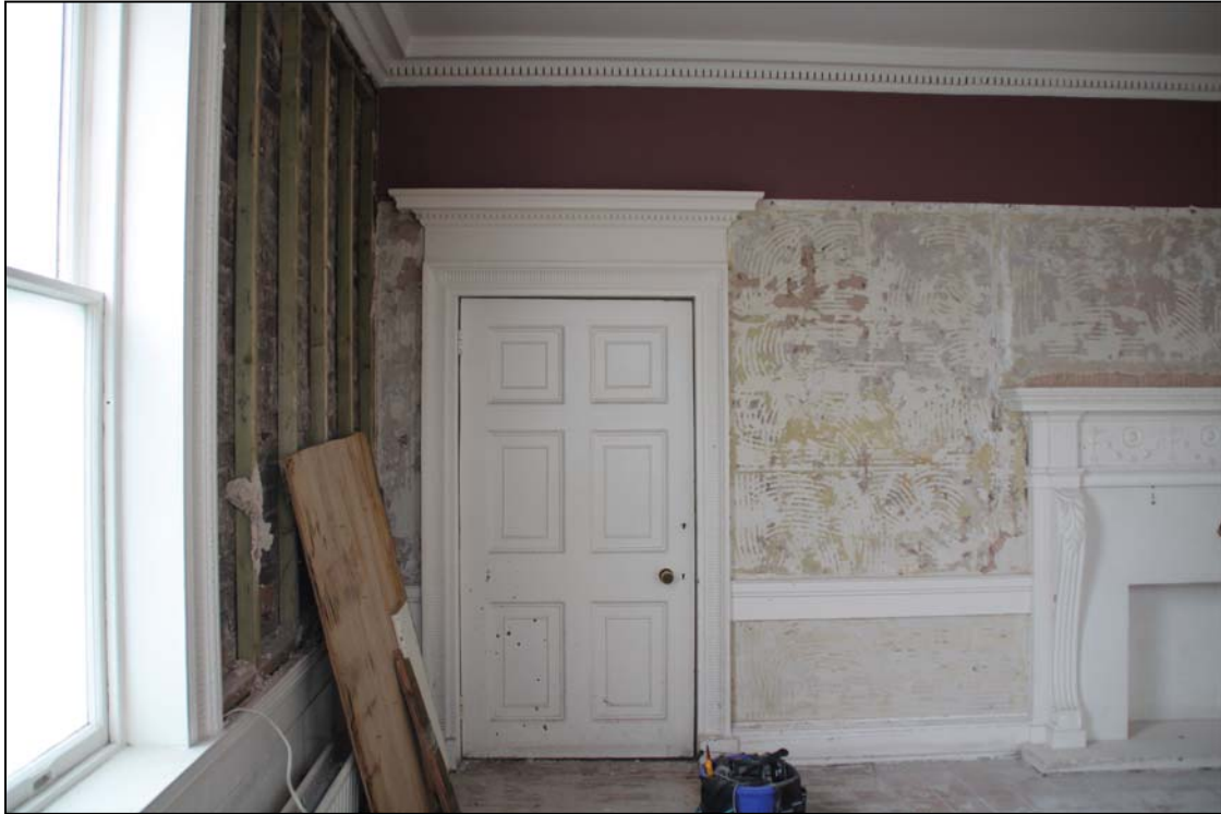
The door into the cupboard at the south-east end of the south-west wall of room 1.1 and the recent studding on the left (no scale)
