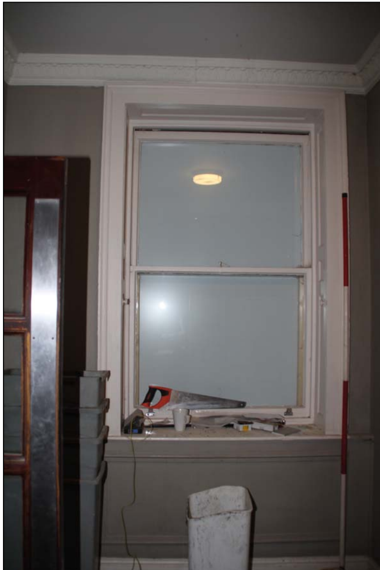
Typical window joinery in the Friary range here in G1 (scale 2m)
