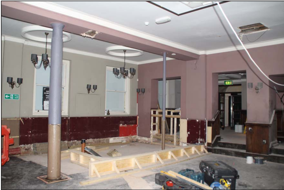
Room G11 looking south (scale 2m)
