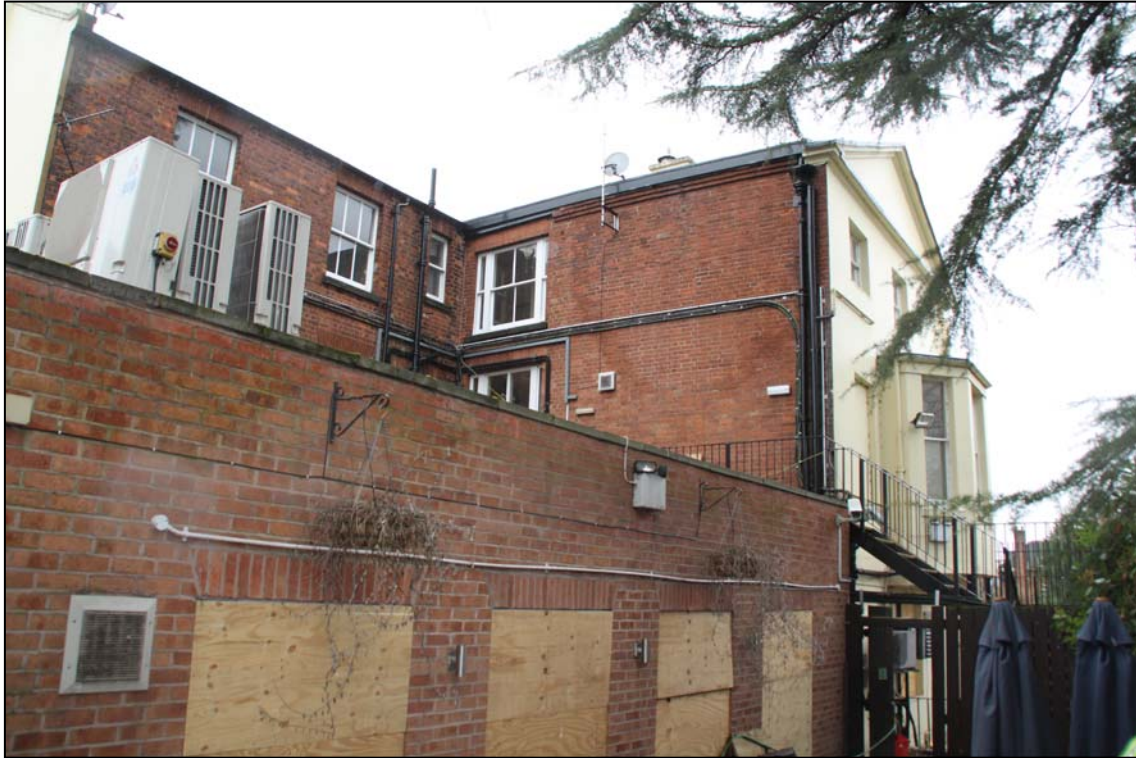
The rear, north-west elevation of the Friary range, looking east
