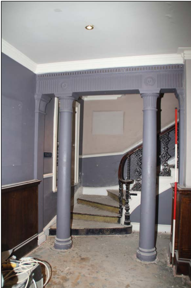
The columnar screen at the foot of the stair ST1, looking south-west (scale 2m)
