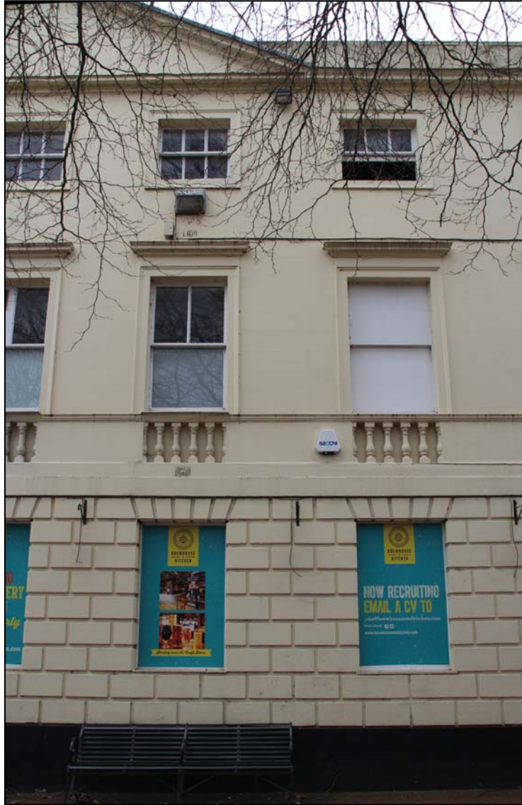
The windows and architectural treatment in the Bird Street elevation
