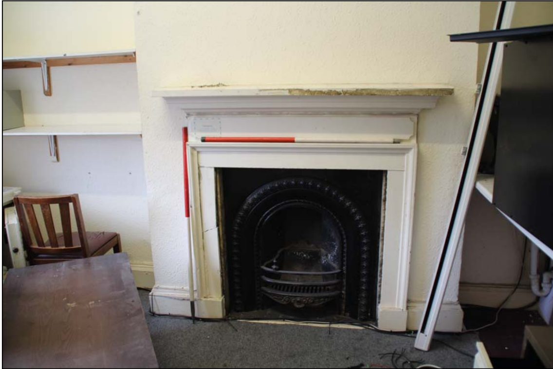
The fireplace in room 1.5 (scales 1m)
