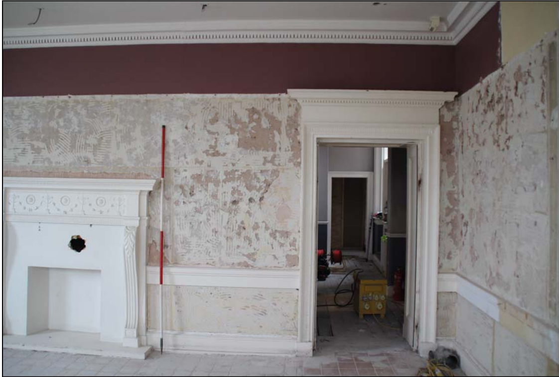
The north-east end of the south-west wall of 1.1 (scale 2m)
