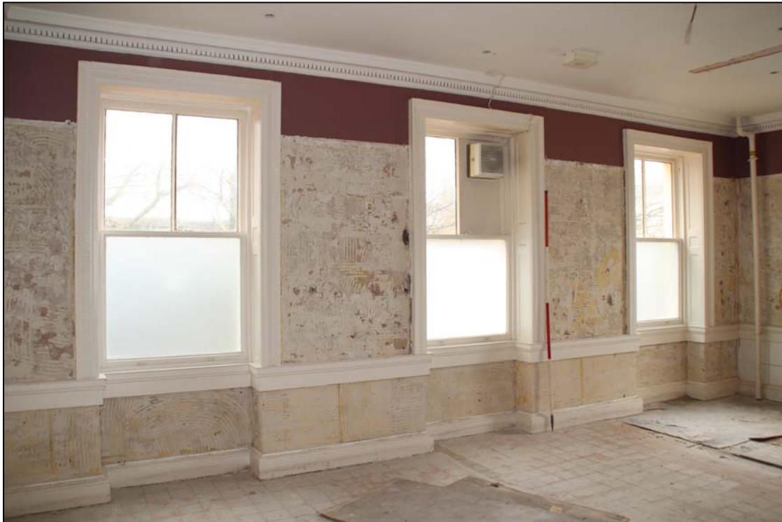
The windows in the Bird Street side of room 1.1 (scale 2m)
