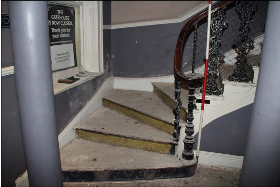
The foot of the stair ST1 (scale 2m)
