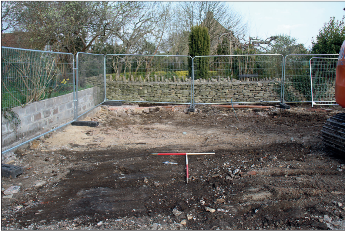
Layer 103, following removal of concrete slab 102, looking east (1m scales)
