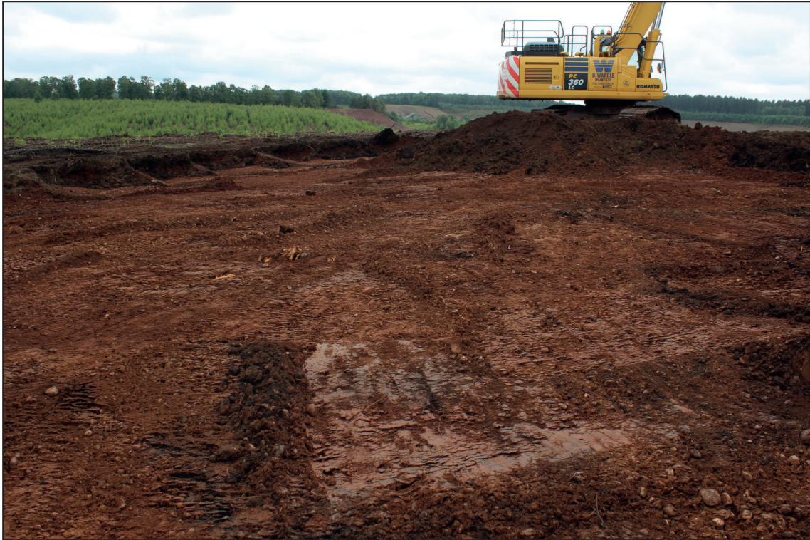
Soil stripping of watching brief area, looking south-west
