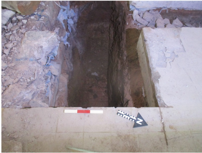
SW facing view of test pit 8 showing natural
