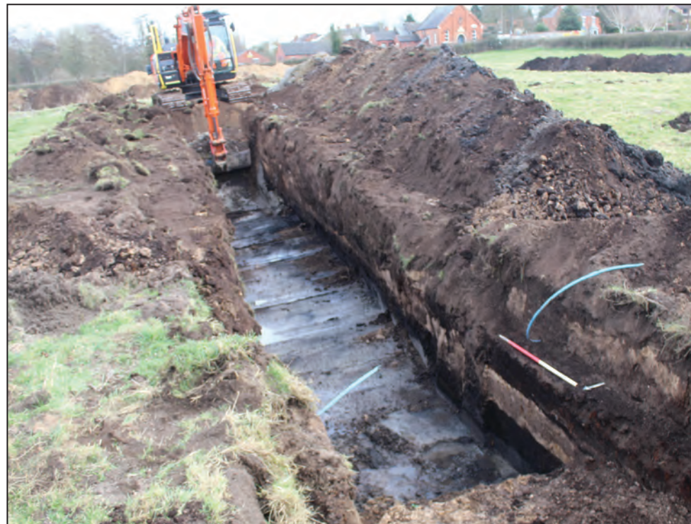
Trench 3, during excavation of palaeochannel 309, looking south-east (scale 1m)
