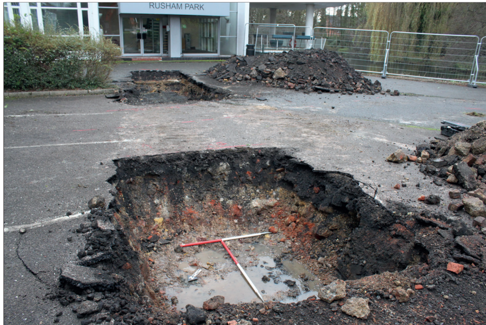
Trench 11, looking south-east (1m scales)
