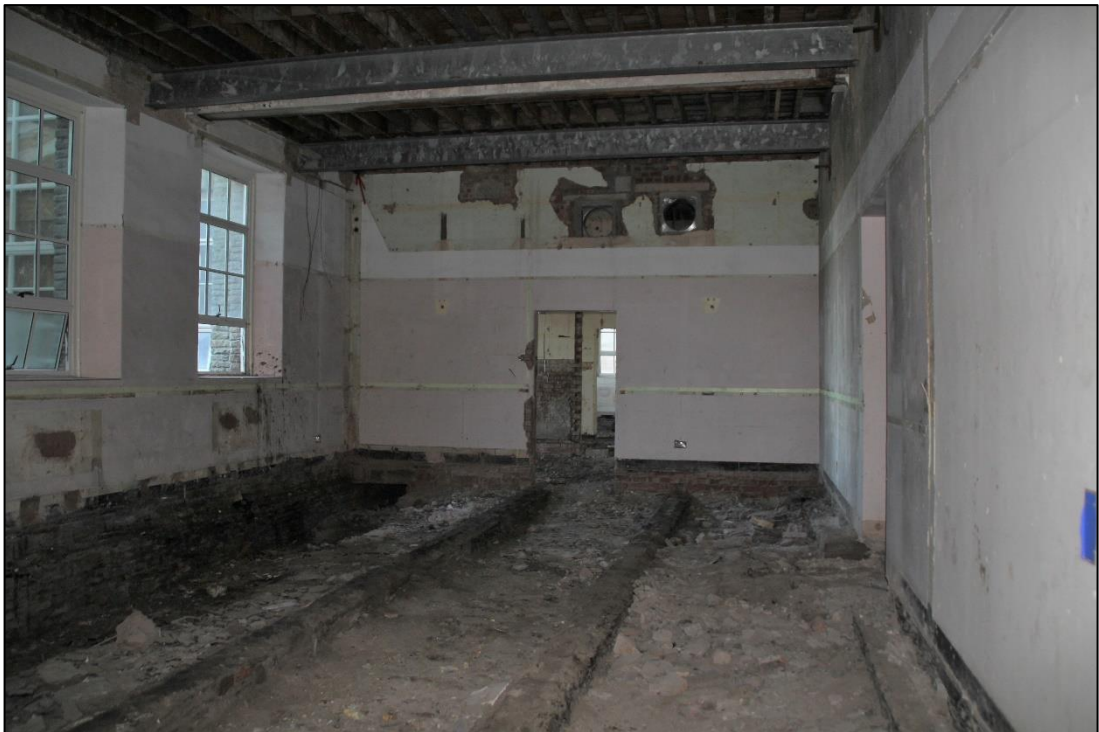
Photo 15 Room G1 looking east
