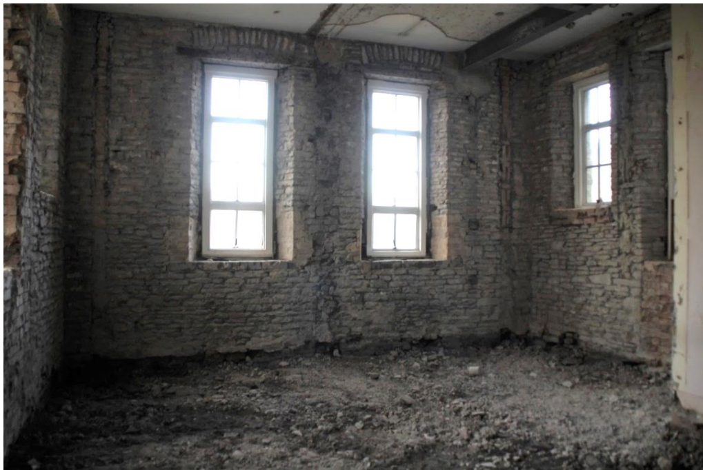
Photo 20 Room G3 looking north
