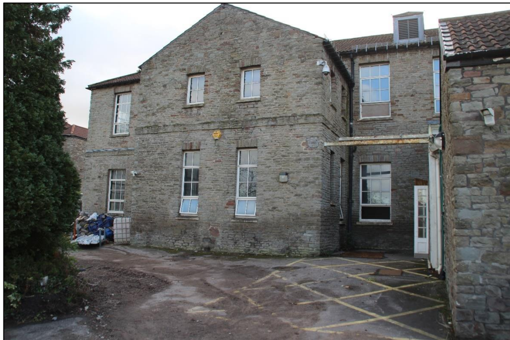
Photo 8 The rear eastern section of the Building
