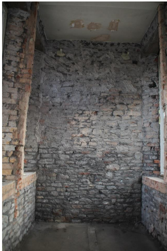
Photo 30 Looking east in Room F2
