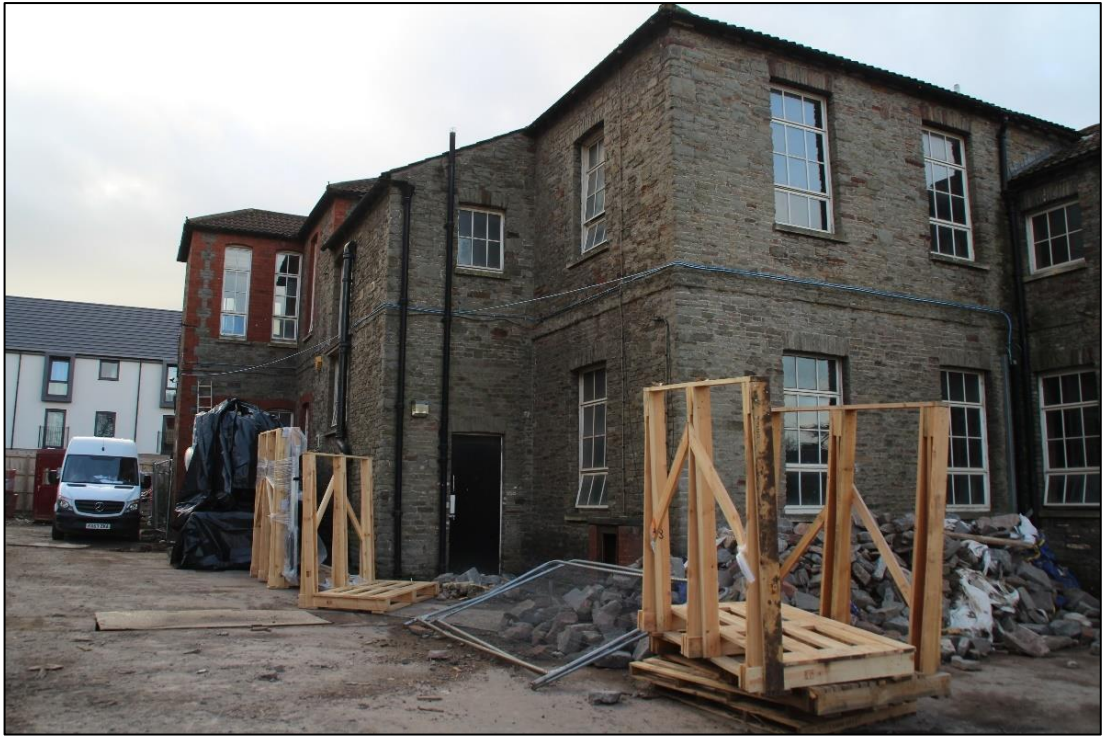
Photo 10 The western elevations of the Building
