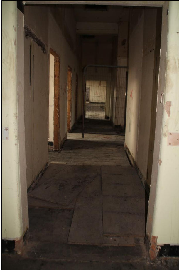
Photo 31 Looking west through subdivided central area
