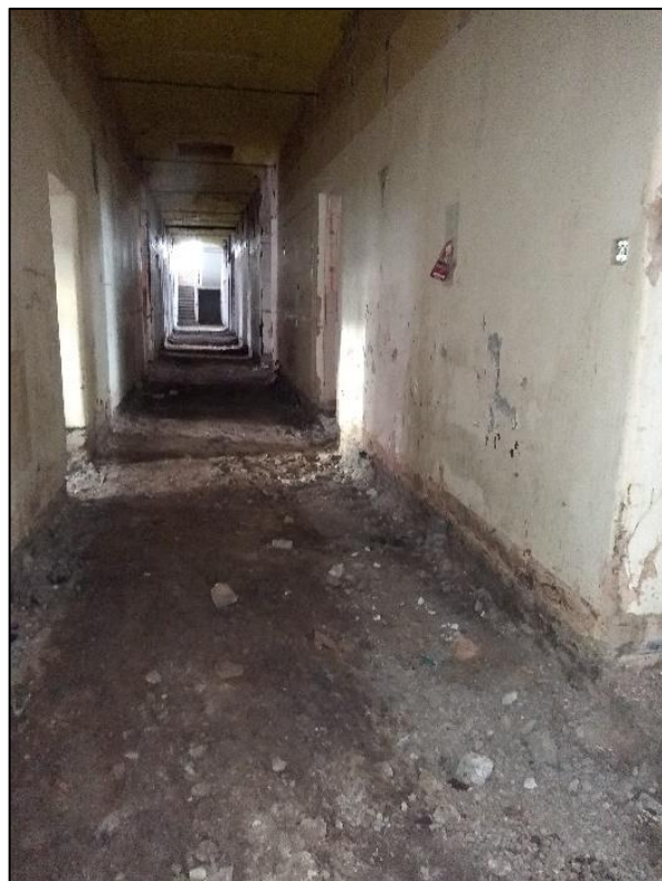
Photo 14 View looking west along the ground floor corridor
