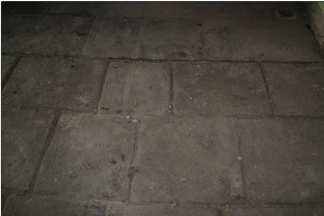
Photo 27 Detail of flagstones, upper corridor
