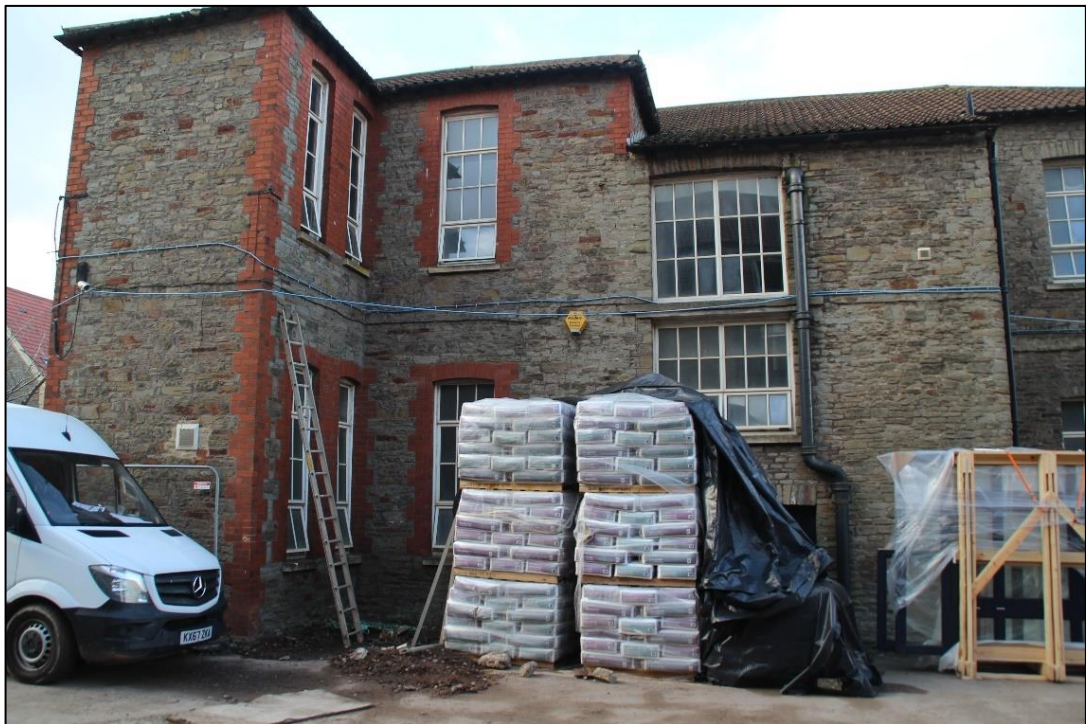
Photo 11 Detail of the western elevation of the Building
