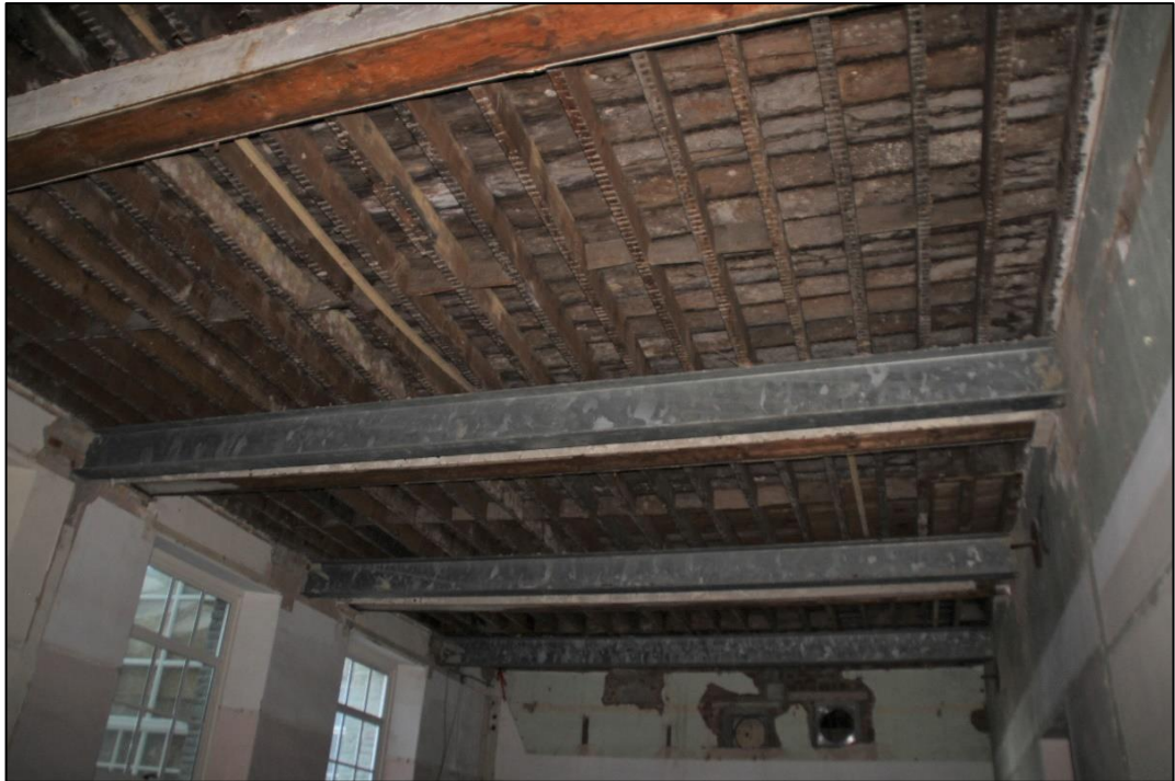
Photo 16 Room G1 looking up
