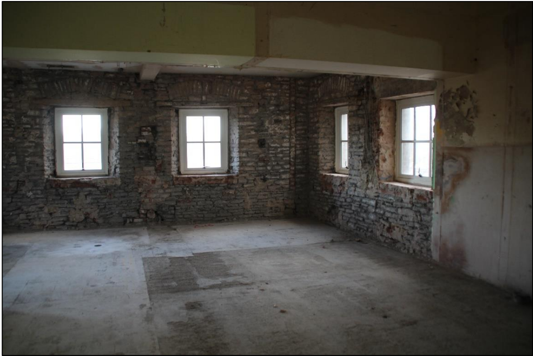
Photo 32 Looking north in Room F3
