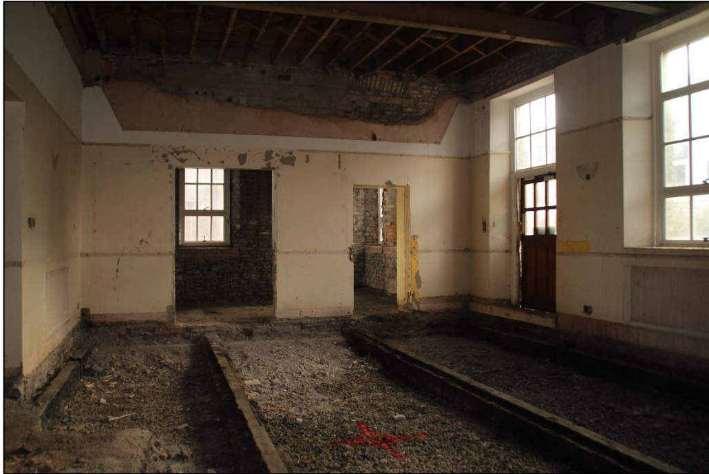
Photo 21 Room G4 looking east
