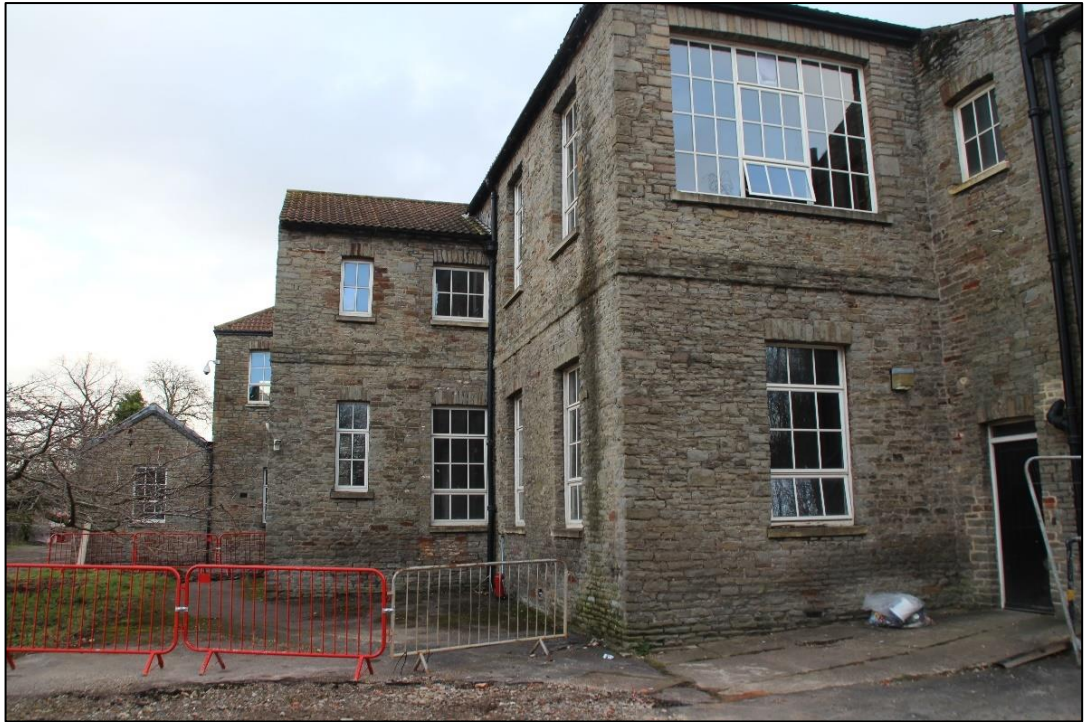
Photo 6 The rear western section the Building
