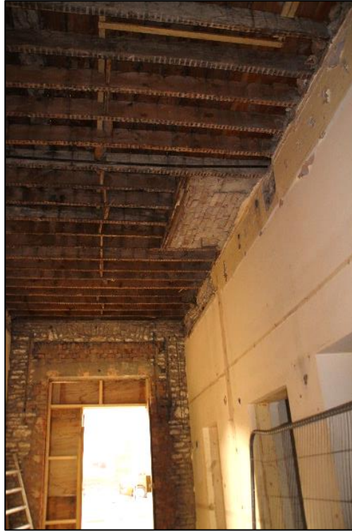
Photo 24 The front entrance hall with possible brick hearth above, looking south
