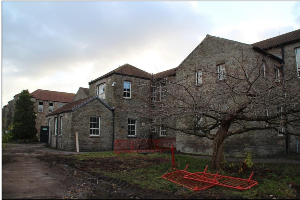
Photo 7 The rear of the Building taken looking east
