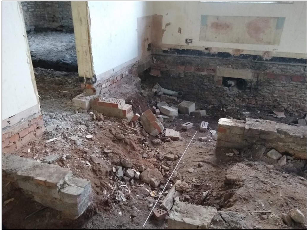
Photo 19 Room G2 looking down and to the north-west
