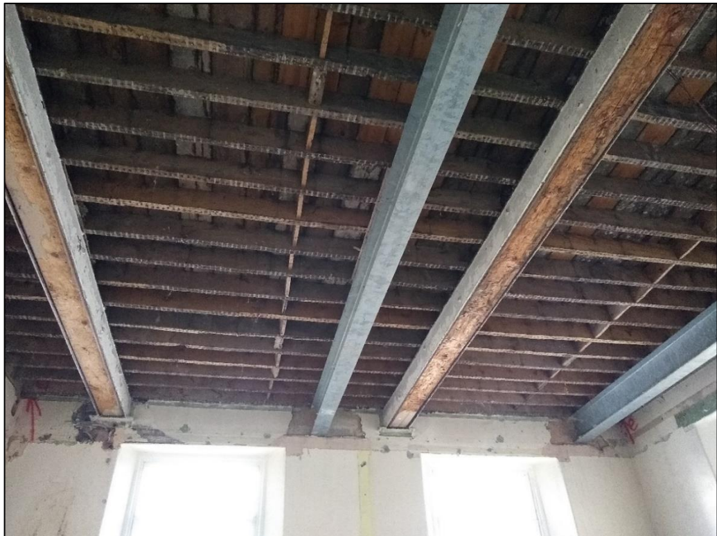
Photo 18 Room G2 looking up
