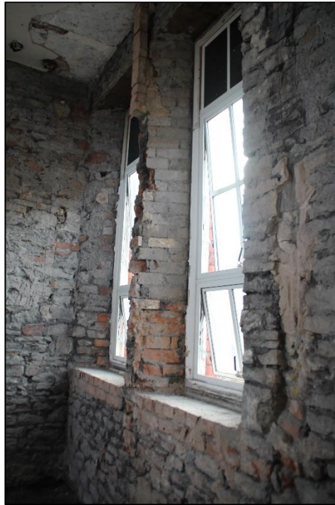
Photo 22 Room east off G4, looking south-east
