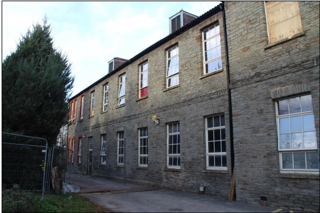
Photo 3 The front (southern) eastern section of the Building
