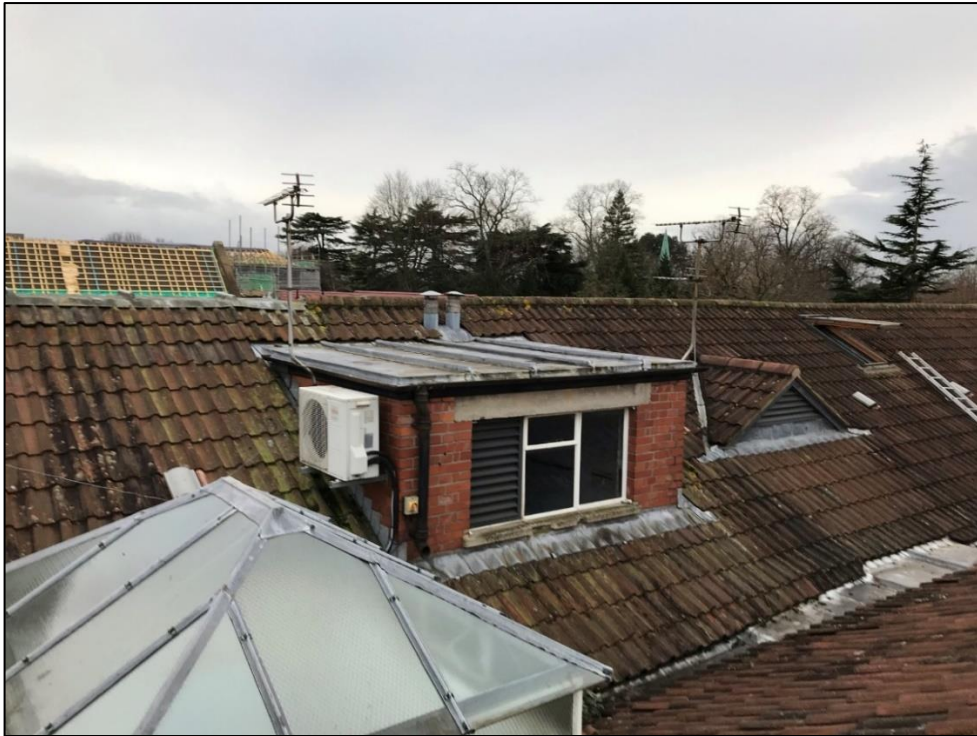
Photo 39 Detail of dormer on roofscape
