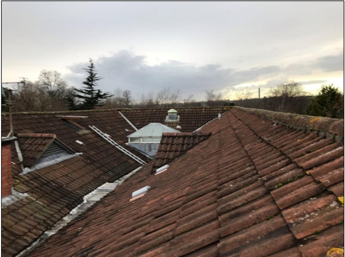
Photo 38 Roofscape looking west
