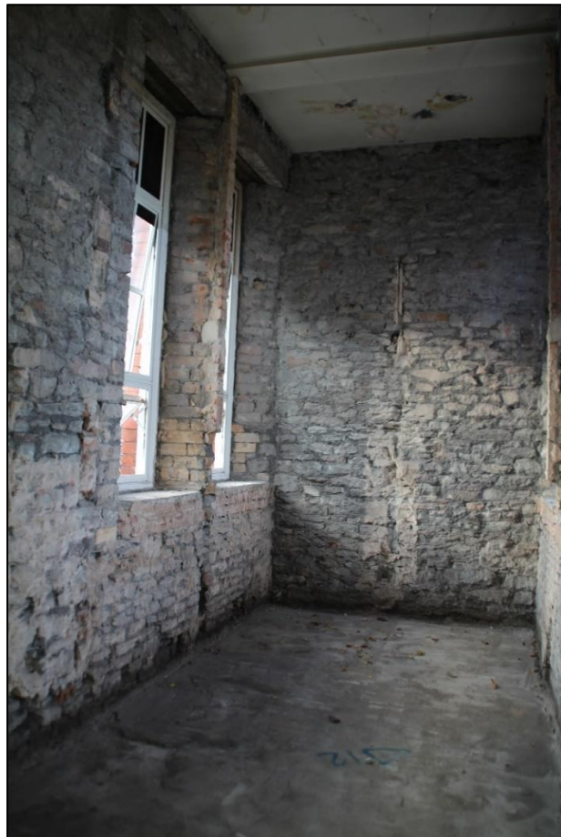
Photo 35 Looking west in the wing to Room F4
