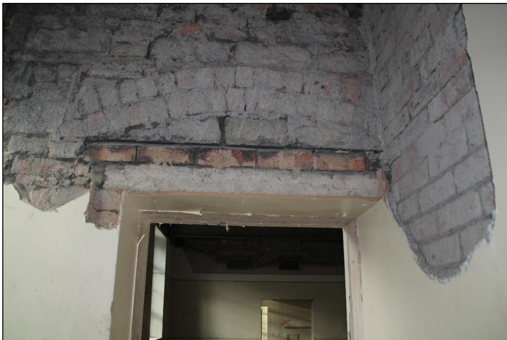
Photo 23 Detail of doorway going into Room G4 from the east
