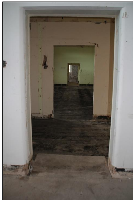
Photo 37 Detail of chamfered doorcases
