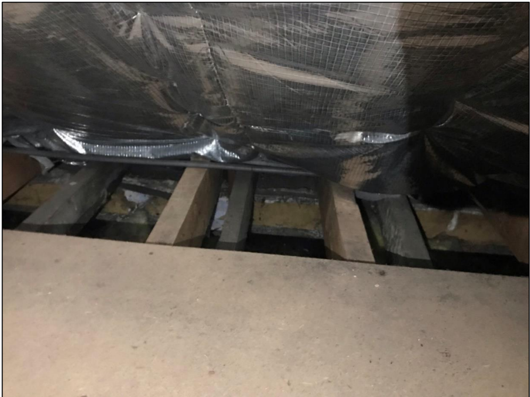
Photo 41 Detail of new and old timbers
