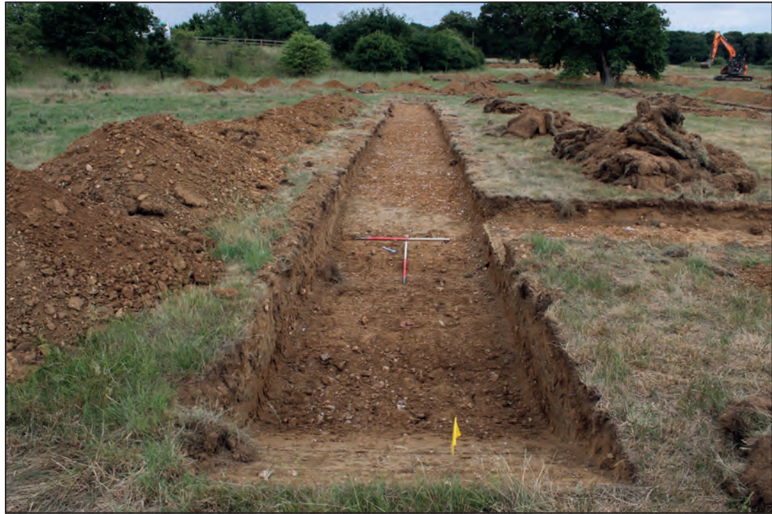
General view of Trench 1, looking south-west (1m scales)
