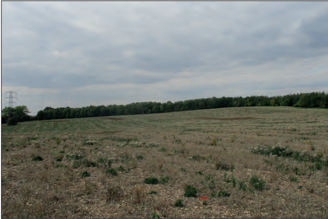
General view of the backfilling looking, looking north-west
