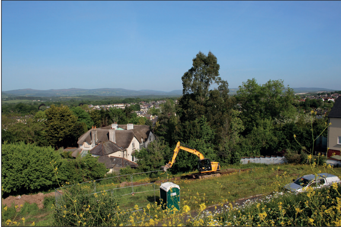
Site overview, looking west
