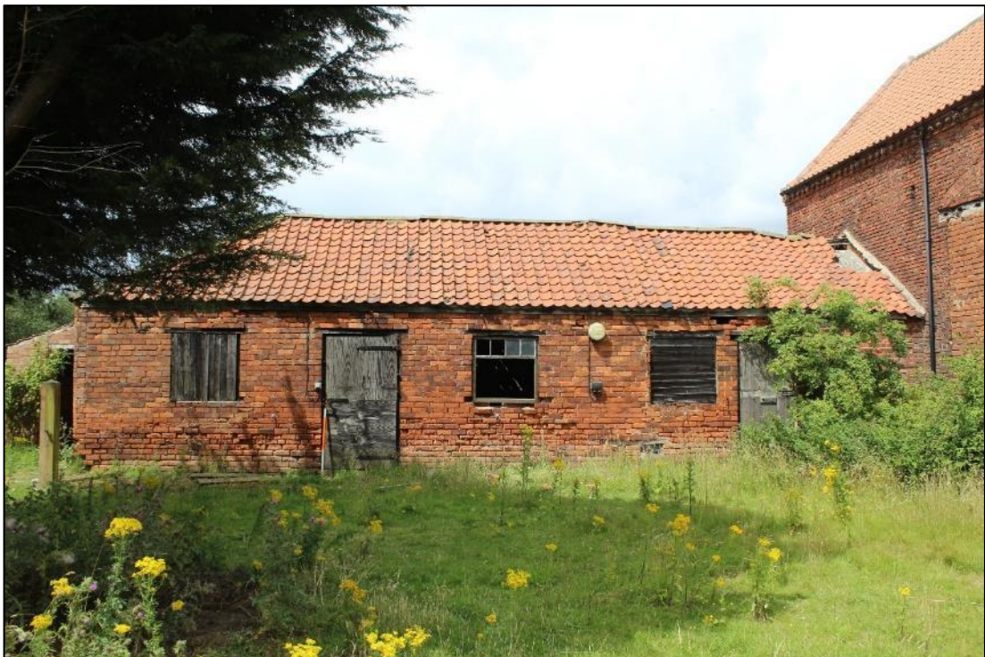
Photo 31: Building C, eastern elevation
