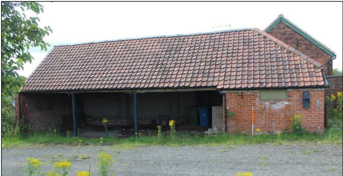
Photo 41: Building E, northern elevation
