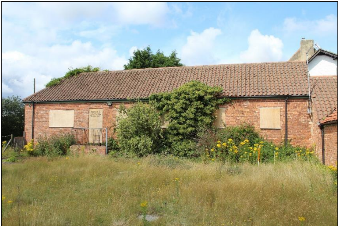
Photo 52: Building F, eastern elevation
