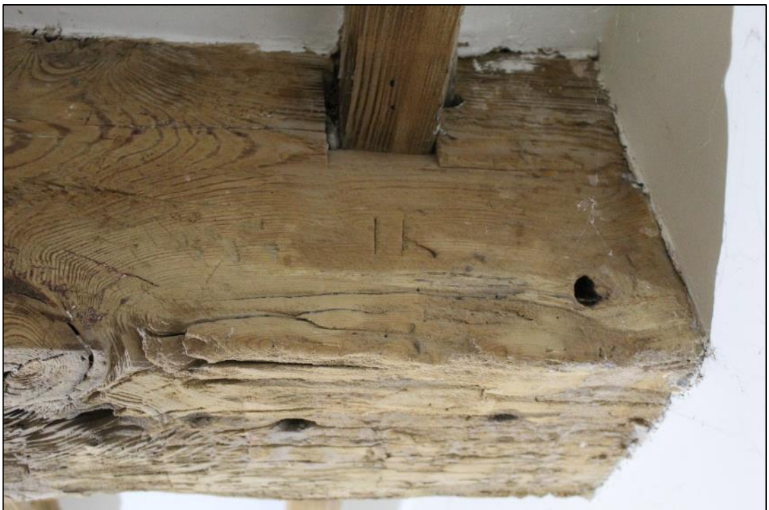
Photo 27: Detail of carpenter's mark at western end of bridging beam
