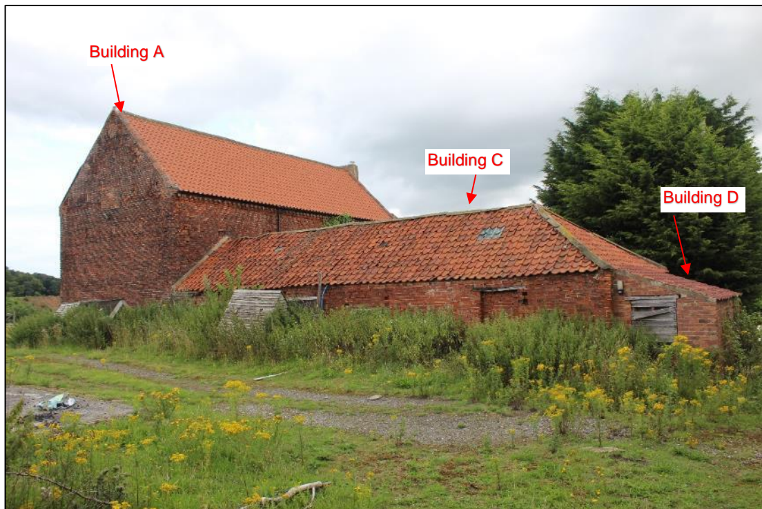
Photo 1: Overview of Farm building, looking north-east
