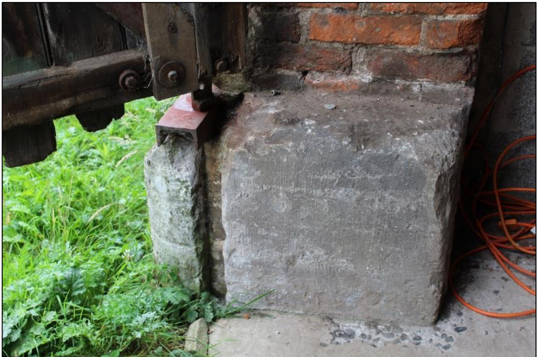
Photo 6: Plank groove within stone base, northern threshing doors of Building A
