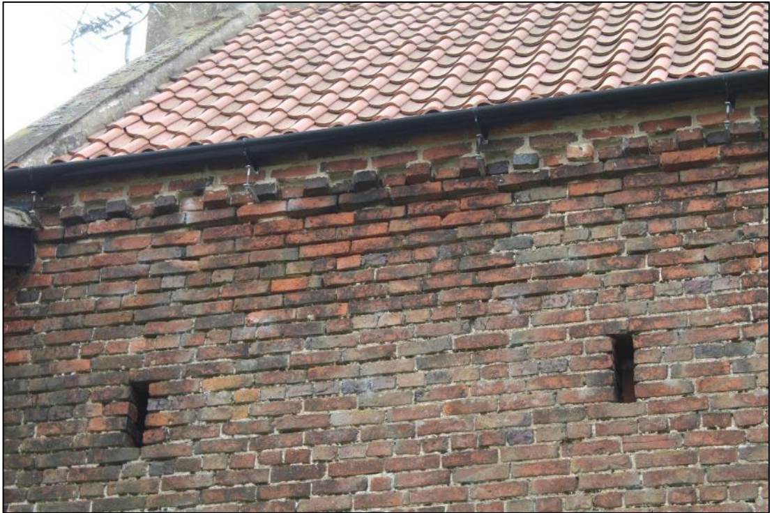
Photo 4: Dentils beneath roof eaves, Building A, northern elevation
