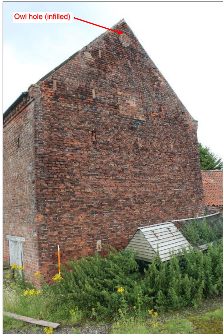
Photo 8: Building A, western elevation
