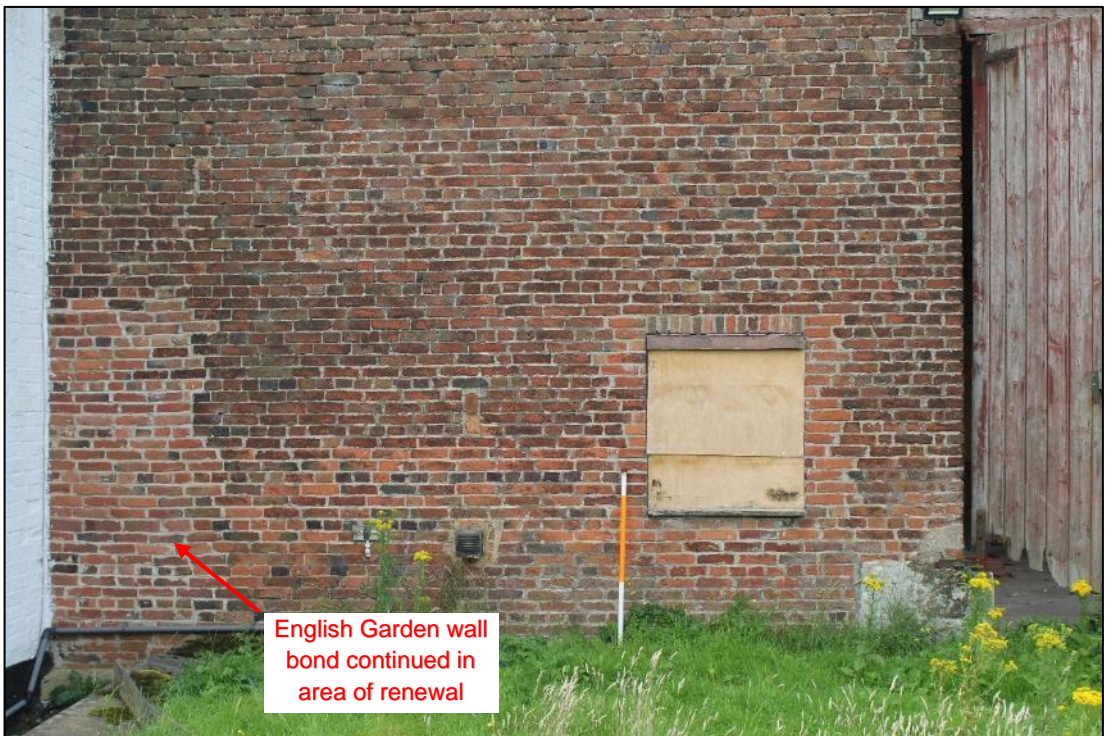
Photo 3: Detail of brickwork, Building A, northern elevation
