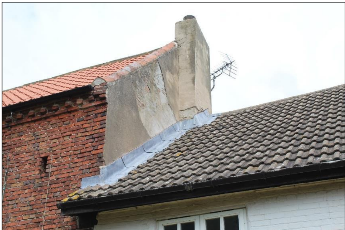
Photo 21: Detail of chimney between Buildings A and B
