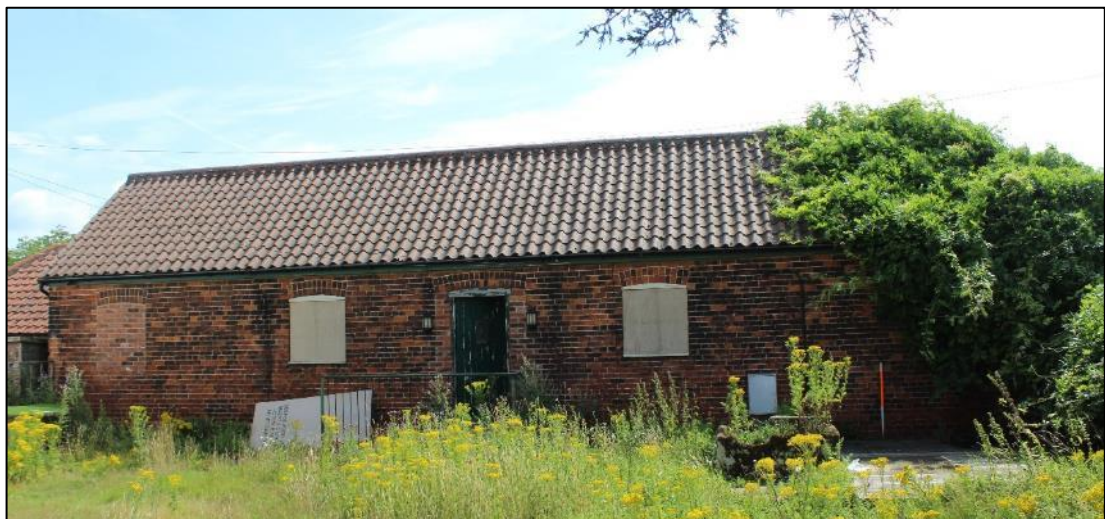
Photo 49: Building F, western elevation
