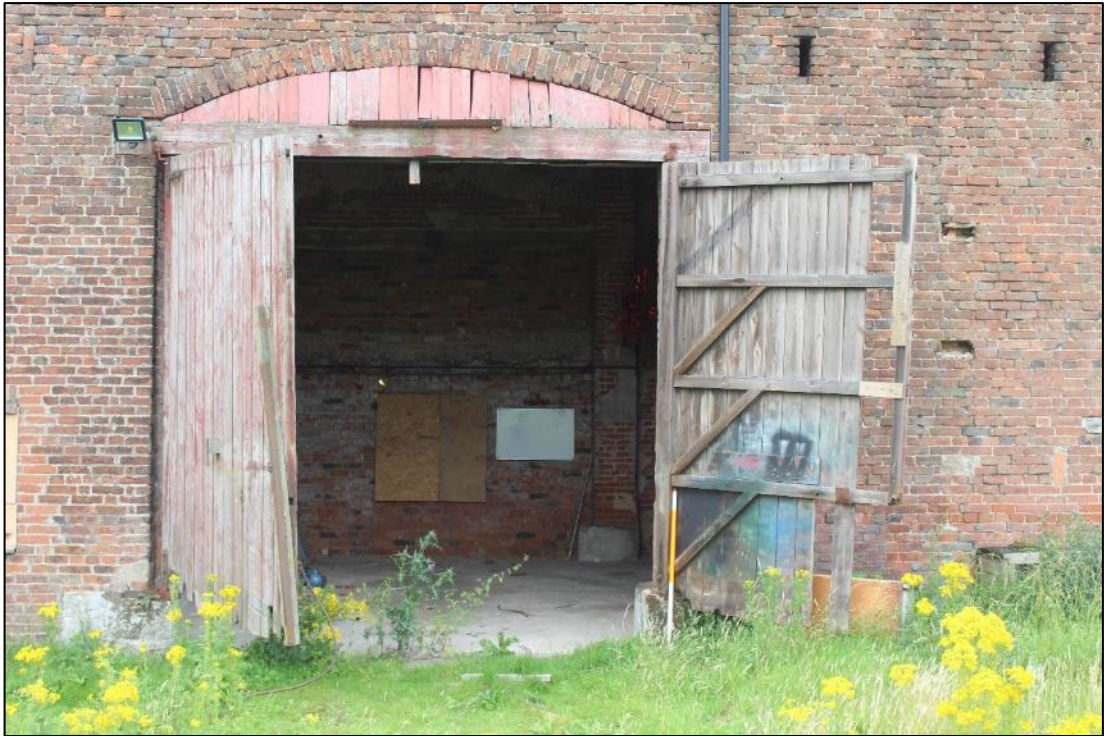
Photo 5: Threshing doors within northern elevation of Building A
