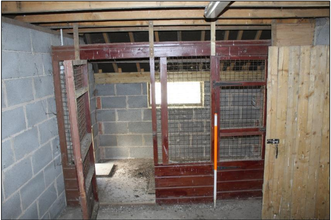
Photo 48: Room E2, looking north
