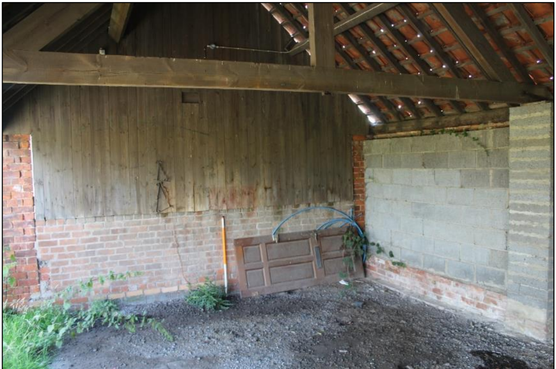
Photo 47: Overview of Room E1, looking south-east
