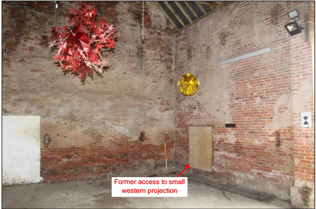
Photo 11: Overview of western extent of Building A interior
