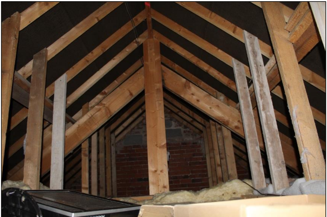
Photo 56: Detail of roof structure within Building F
