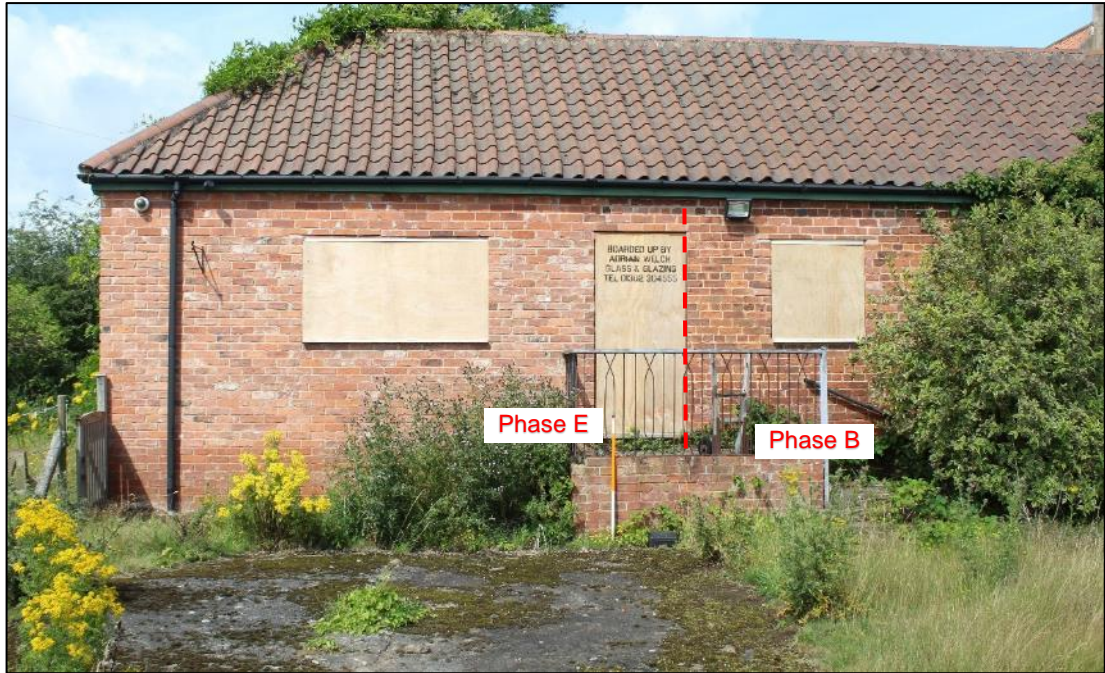
Photo 53: Building F, southern extent of eastern elevation
