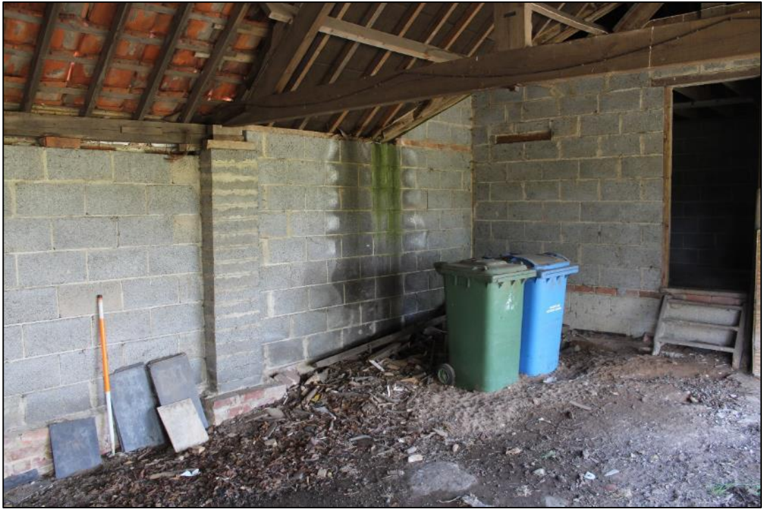
Photo 46: Overview of Room E1, looking south-west
