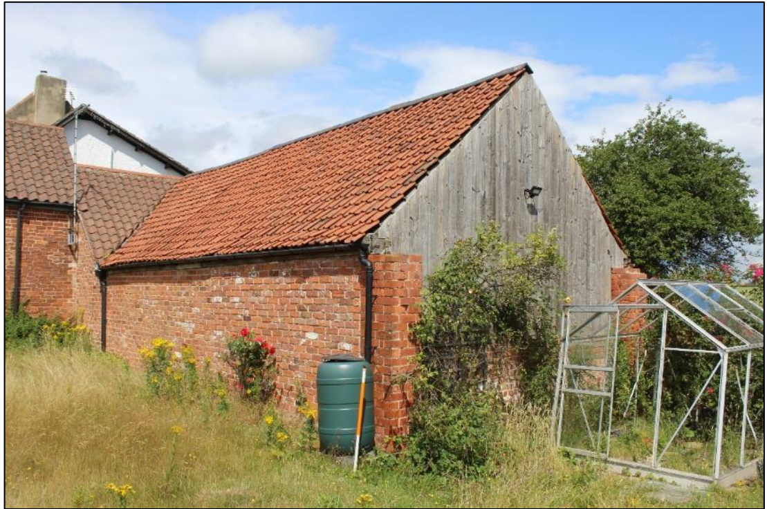
Photo 43: Building E, eastern and southern elevations
