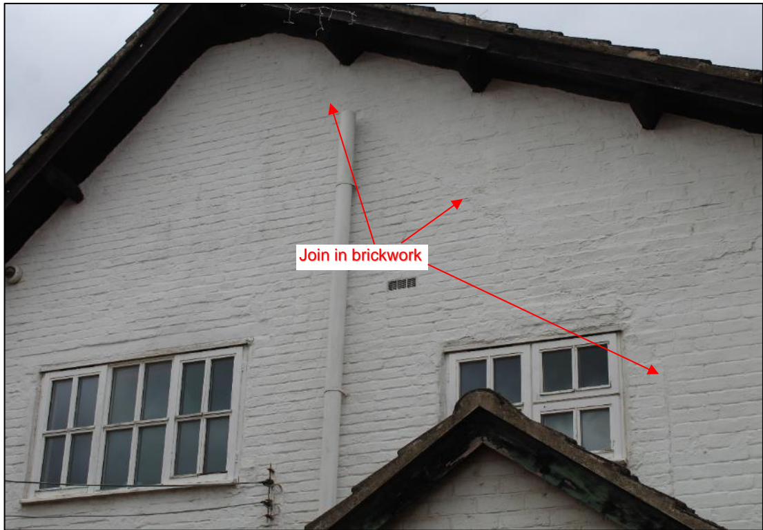
Photo 23: Detail of phased brickwork on eastern elevation
