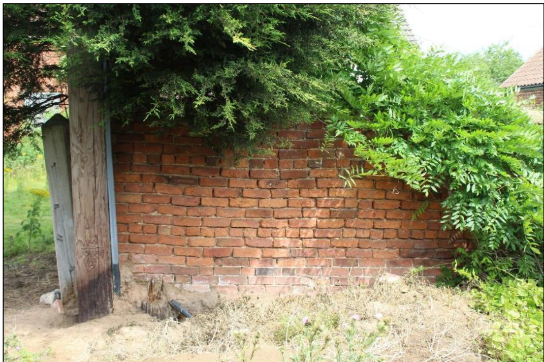
Photo 57: Detail of southern boundary wall, looking north
