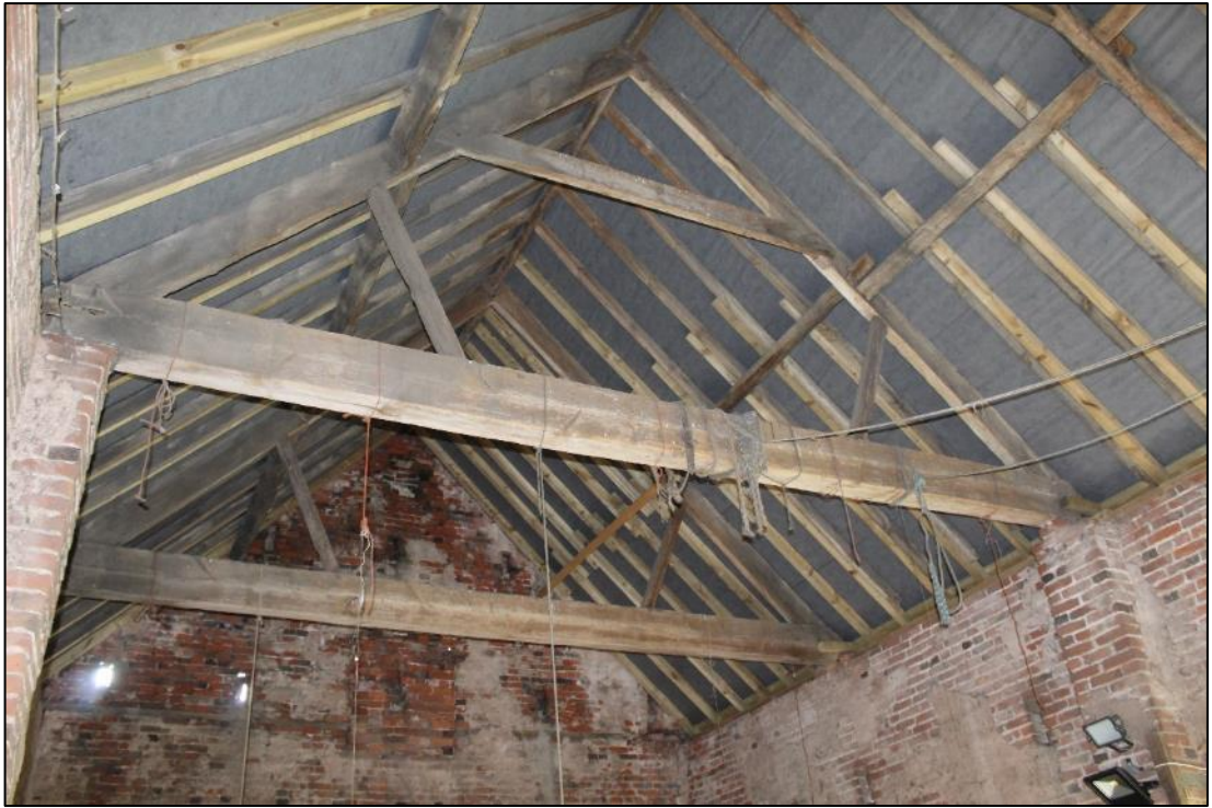
Photo 15: Overview of roof structure, Building A
