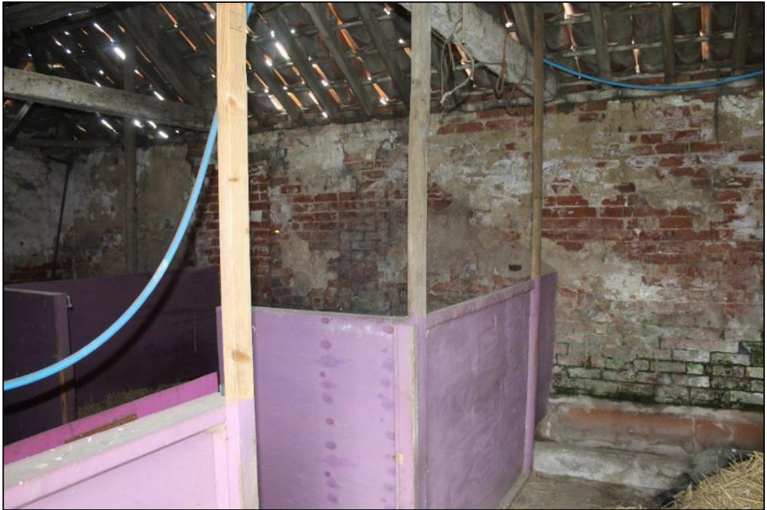
Photo 35: Overview of Room C1, looking west
