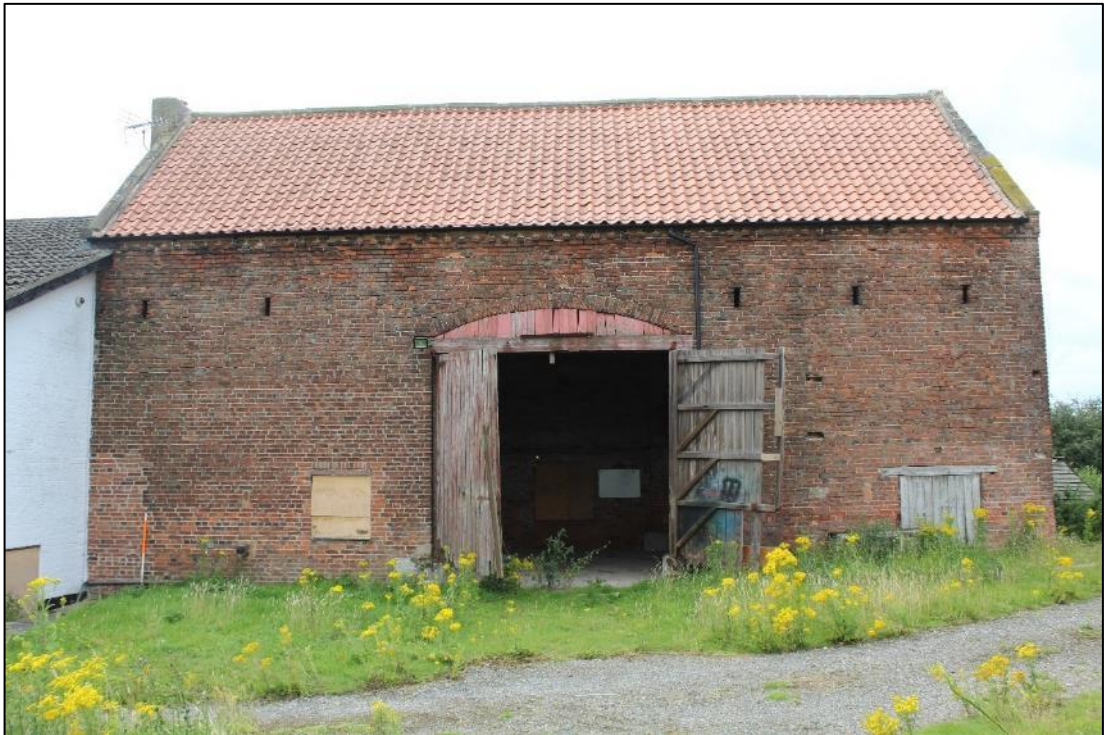
Photo 2: Building A, northern elevation
