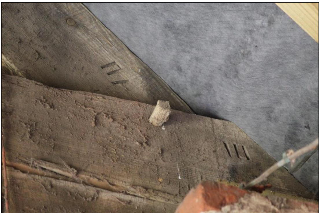
Photo 18: Detail of carpenter marks 'III' on truss III
