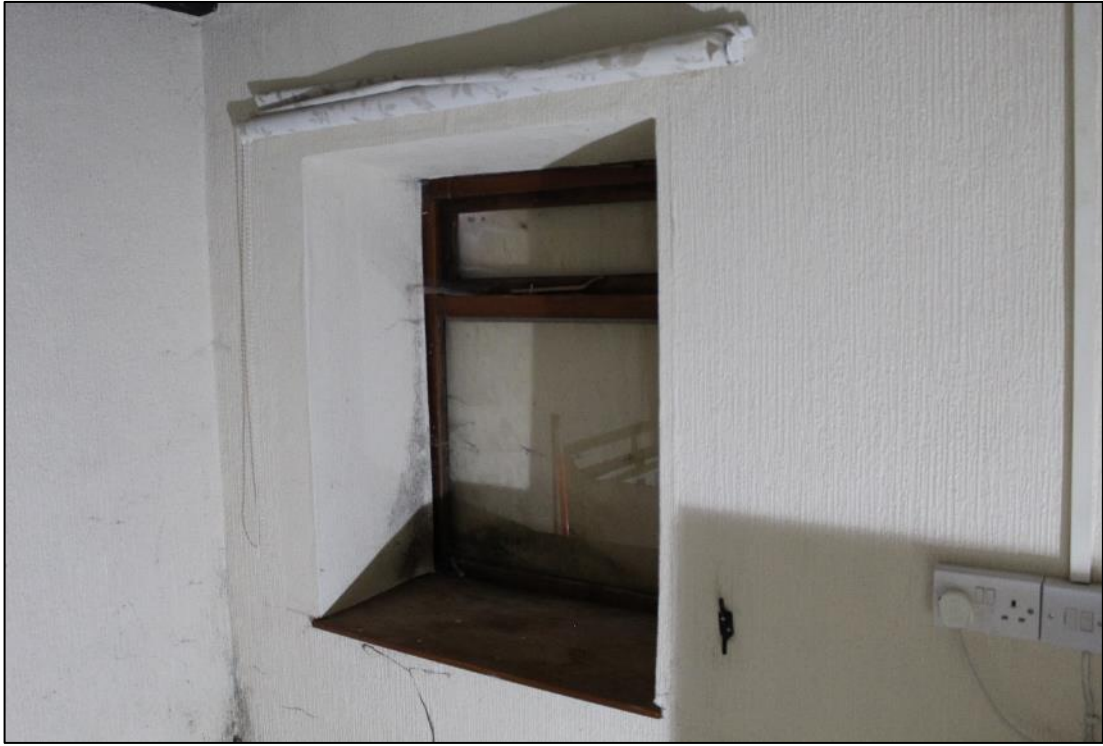
Photo 29: Window within northern wall of Room B7
