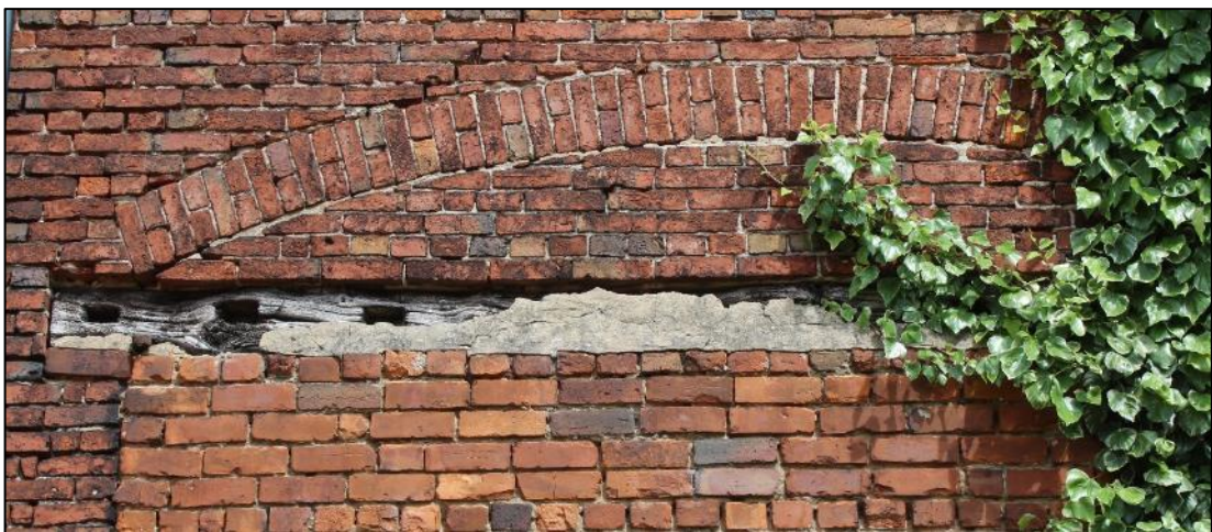
Photo 10: Detail of timber lintel above southern threshing door infill
