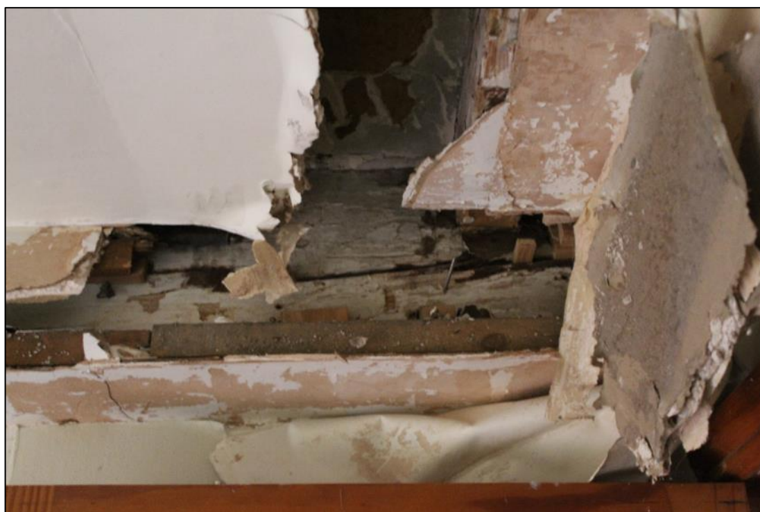
Photo 25: Detail of timber beam within ceiling of Room B2
