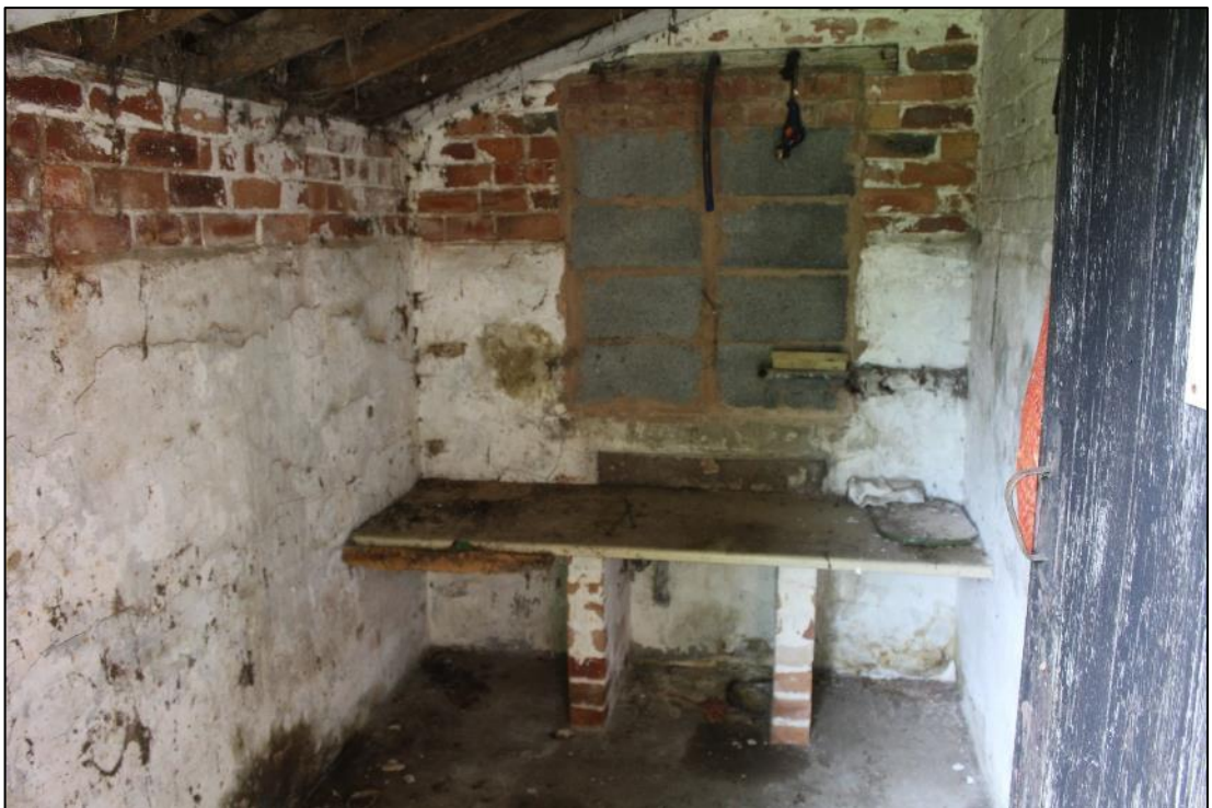
Photo 40: Interior of Building D, looking west
