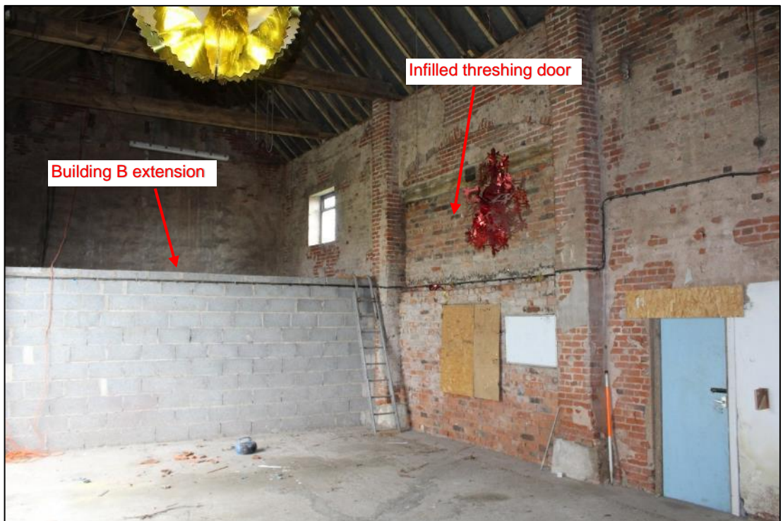
Photo 12: Overview of eastern extent of Building A interior
