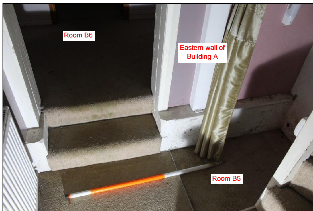
Photo 28: Detail of threshold between Rooms B5 and B6
