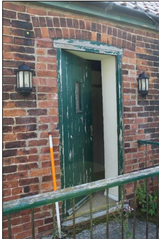
Photo 50: Detail of doorway alterations
