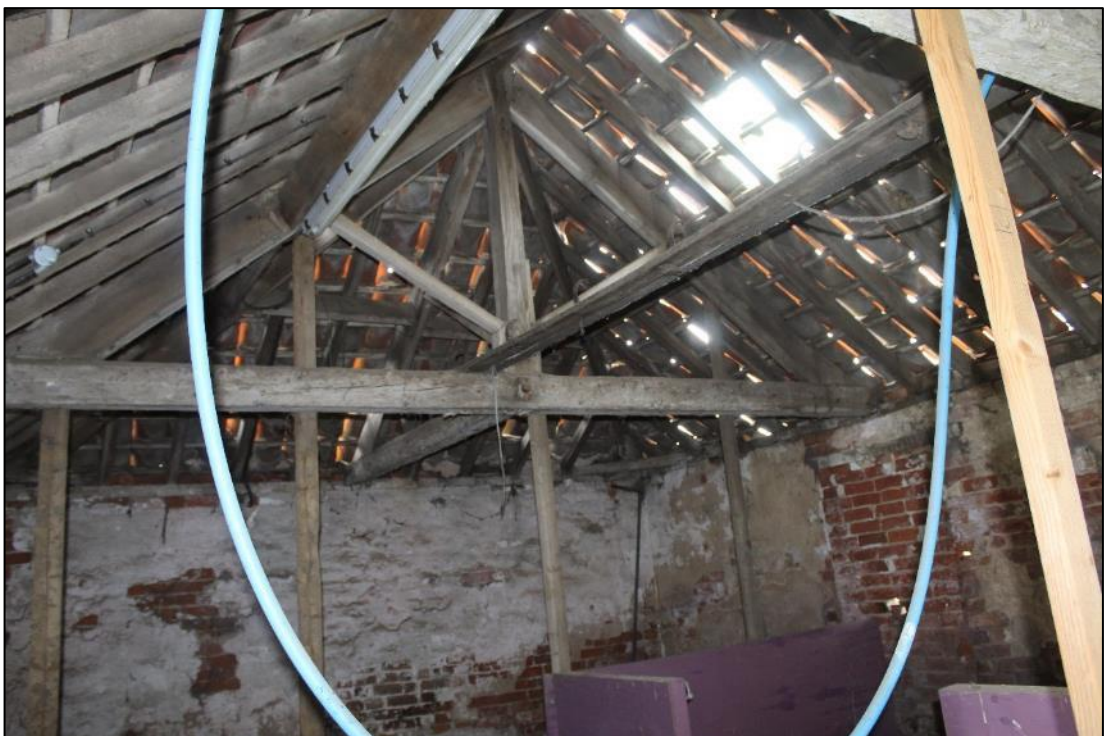
Photo 36: Overview of roof structure within Room C1, looking south
