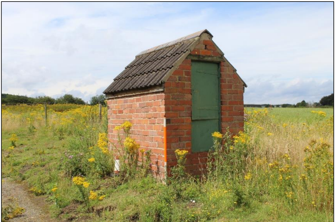
Photo 59: Propane store, looking north-west
