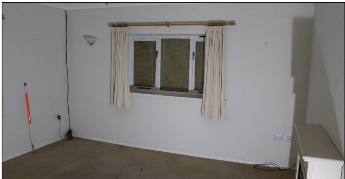
Photo 54: Room F1, looking south-east
