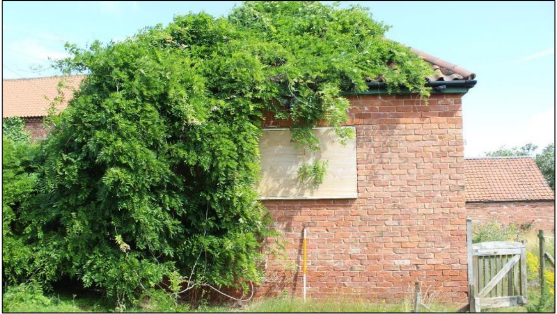
Photo 51: Building F, southern elevation
