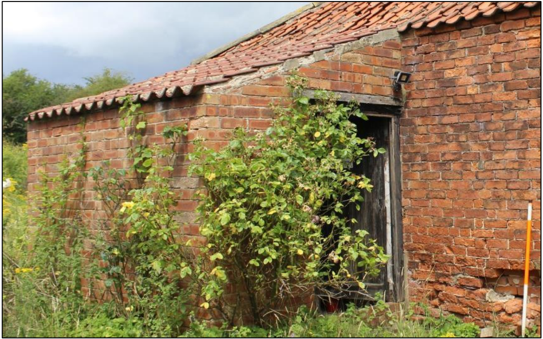
Photo 39: Building D, looking north-west
