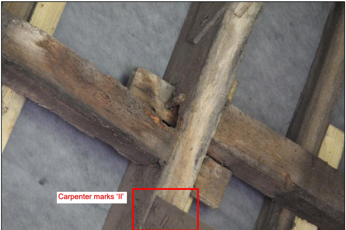
Photo 16: Threaded purlins on southern principal rafter of truss II
