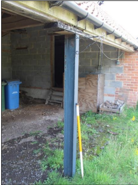
Photo 42: I-beam post, Building E
