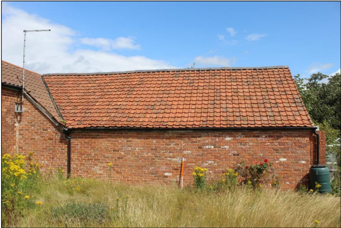
Photo 45: Building E, southern elevation
