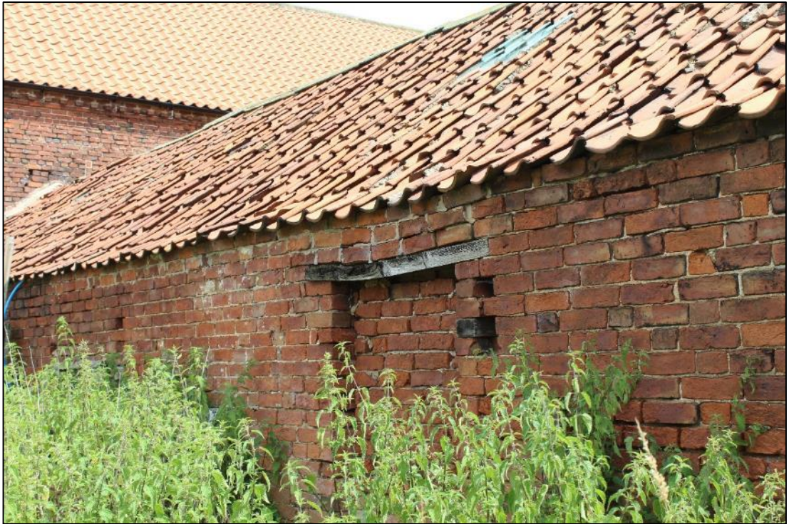
Photo 34: Detail of brickwork within western elevation of Building C
