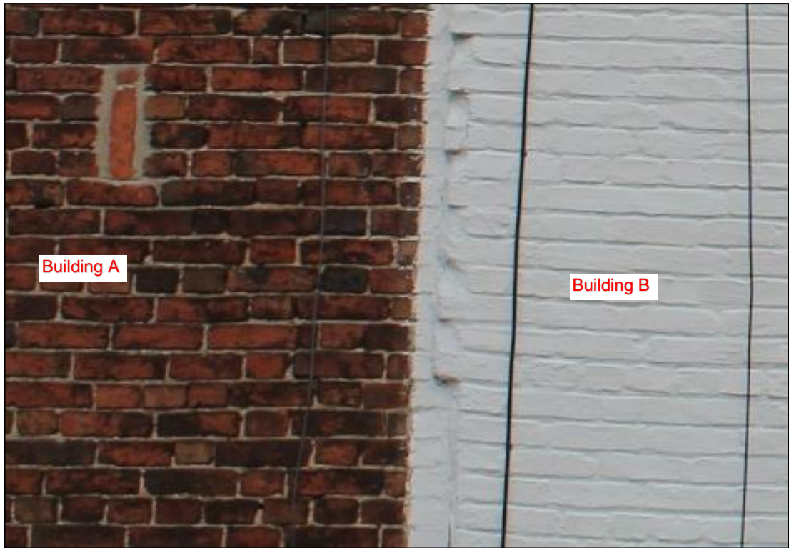
Photo 20: Detail of brickwork joint between Buildings A and B
