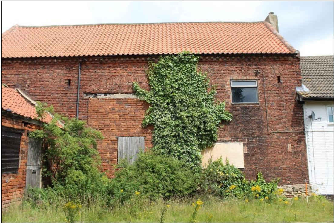
Photo 9: Building A, southern elevation
