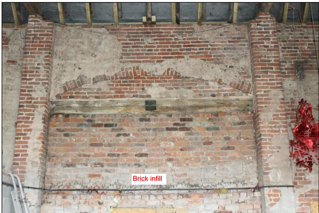
Photo 14: Detail of infilled southern threshing door, upper portion
