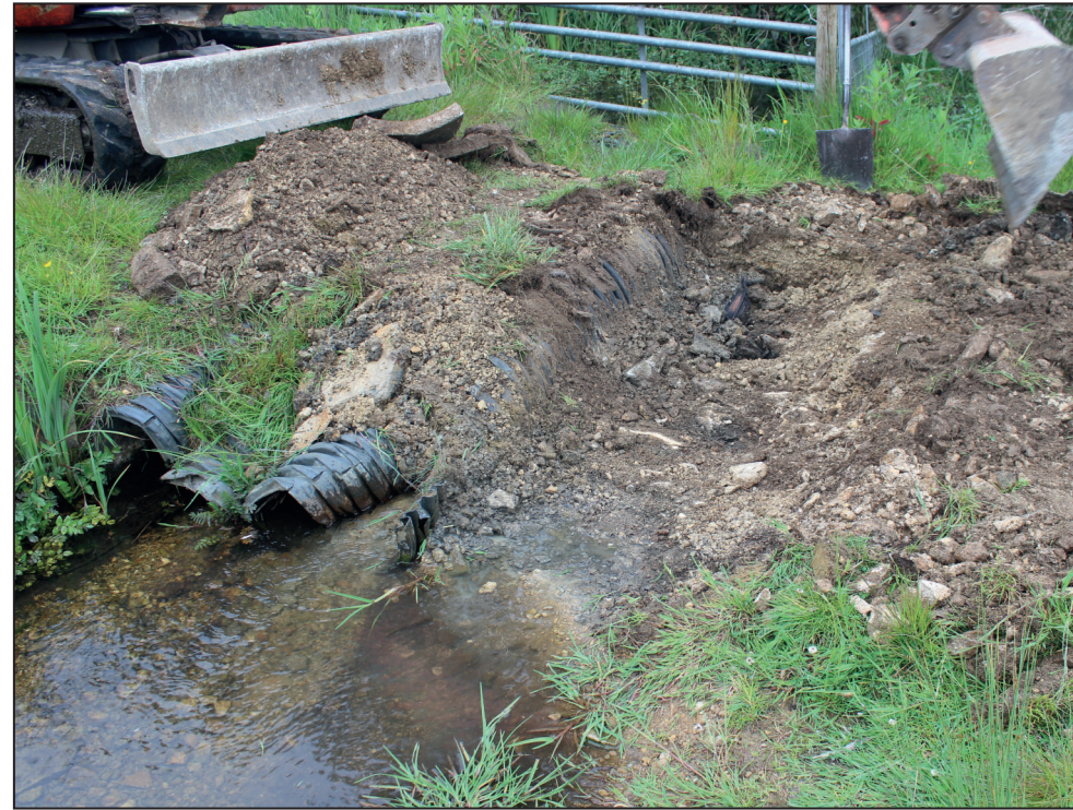
Trench 22, during excavation, showing depth of made ground 2201, looking north-west
