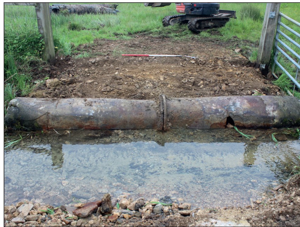
Trench 22, post-excavation, looking west (1m scale)
