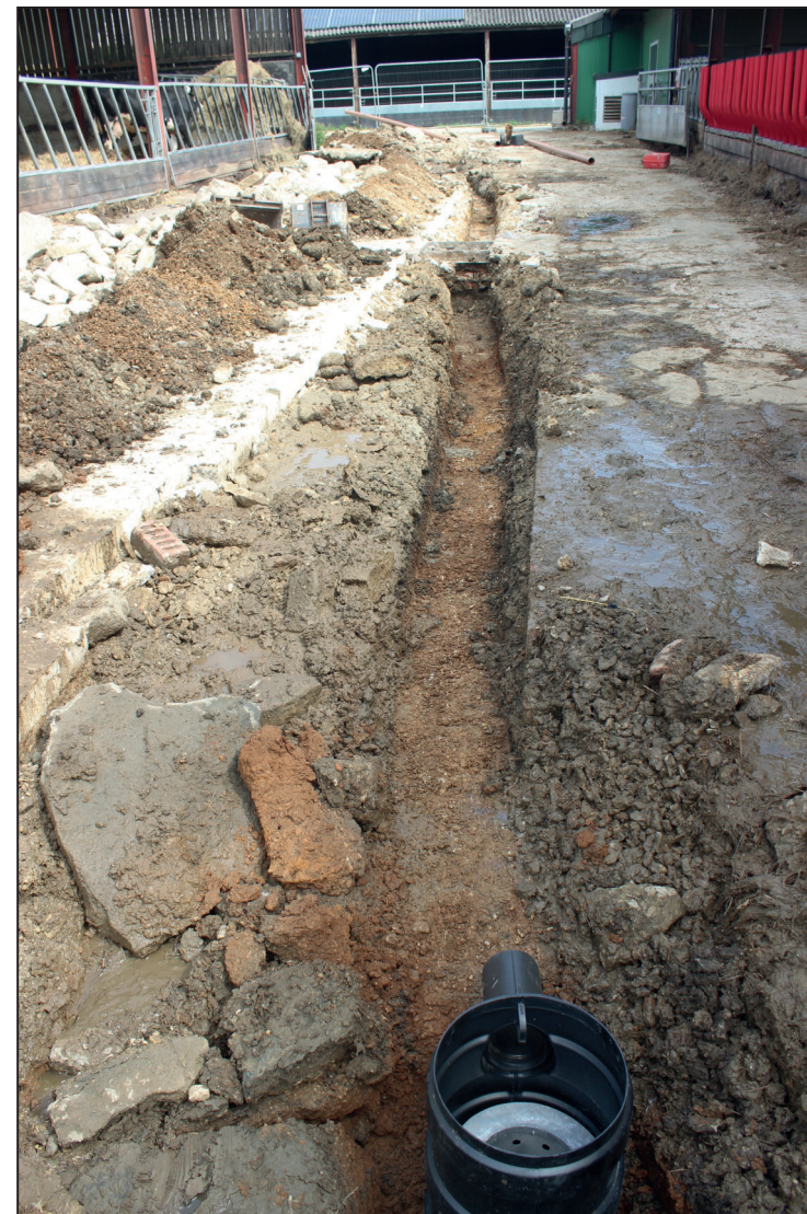
Trench 16, southern section post-excitation, looking north
