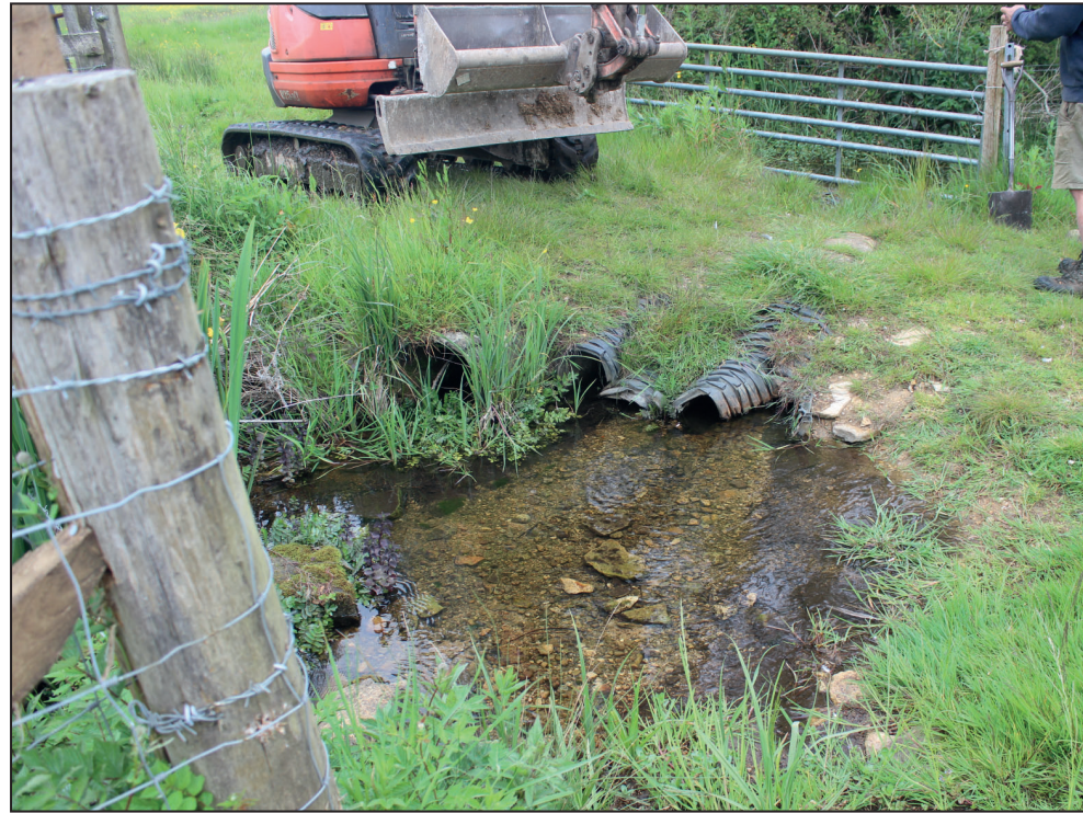
Trench 22, pre-excavation, looking south-east
