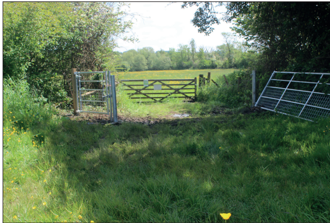
General view of gates in Trench 21, after installation, looking east
