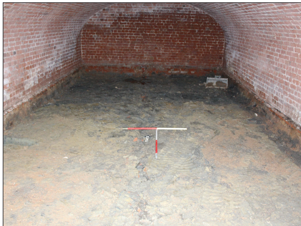
Trench 6 showing brick vaulted sub-basement and reduced ground levels
