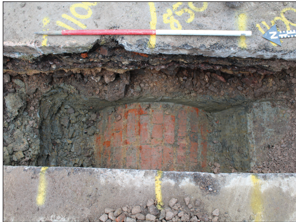
Culvert 105, looking east (scale 1m)
