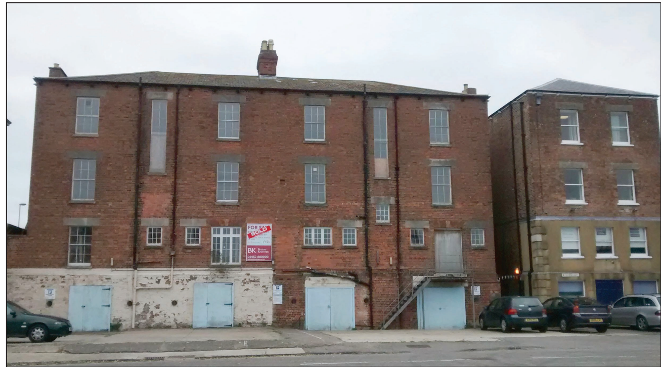
Rear (dockside) elevation of 27-29 (left) and 23-25 (right) Commercial Road
