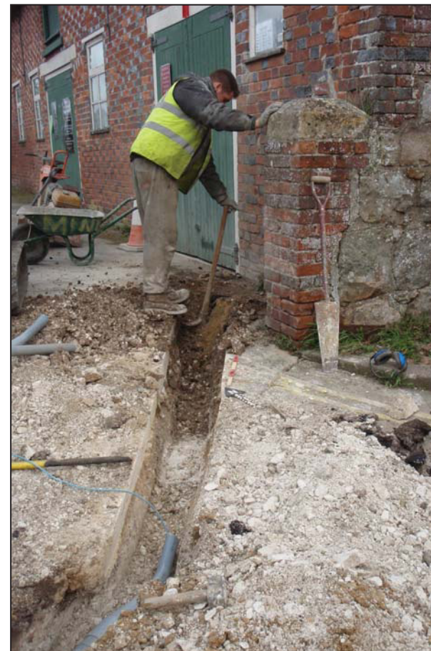
Fig. 6 Telecommunications trench after excavation, looking north east
