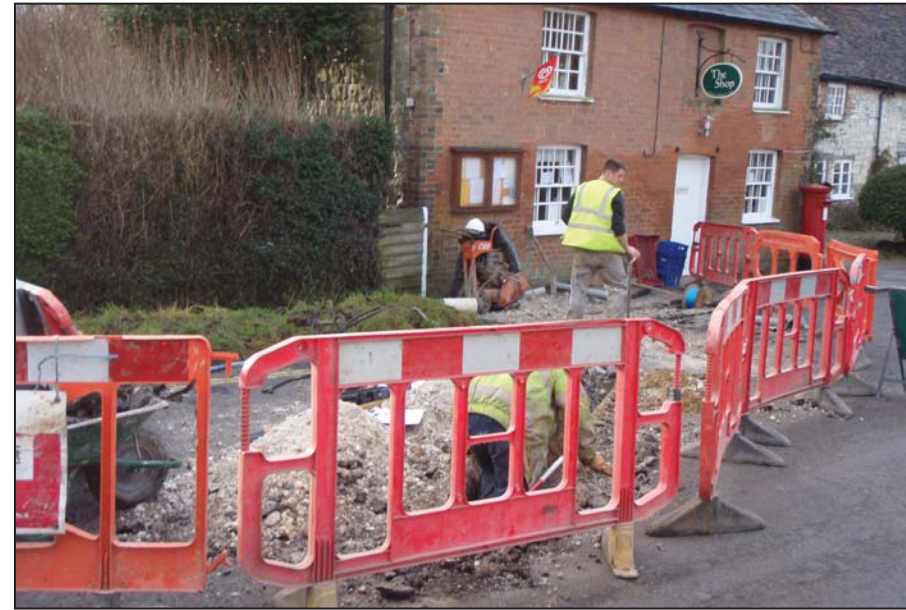
Fig. 4 Excavation of telecommunications trench, looking south west
