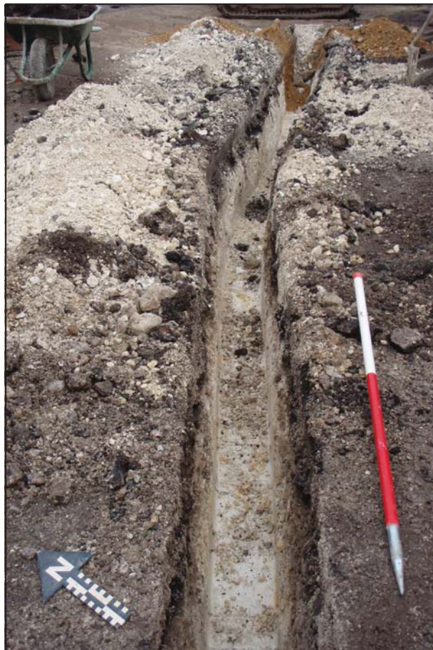
Fig. 5 Telecommunications trench after excavation, looking north east
