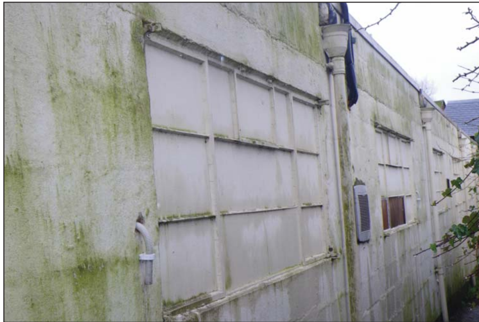
6 Crittall-type windows in the north-east wall of Block 1, looking north
