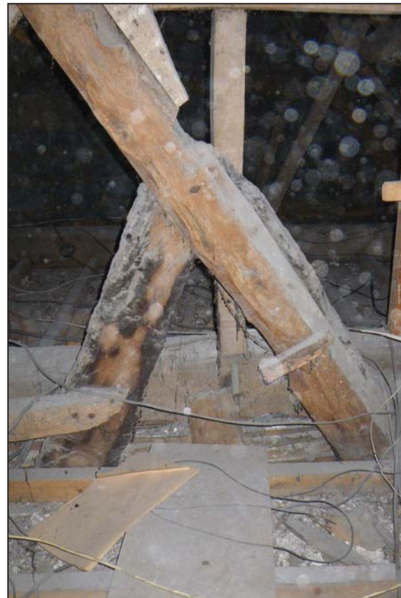
13 The charred phase 1 truss apex, looking north-west partly obscured by phase 2 timbers
