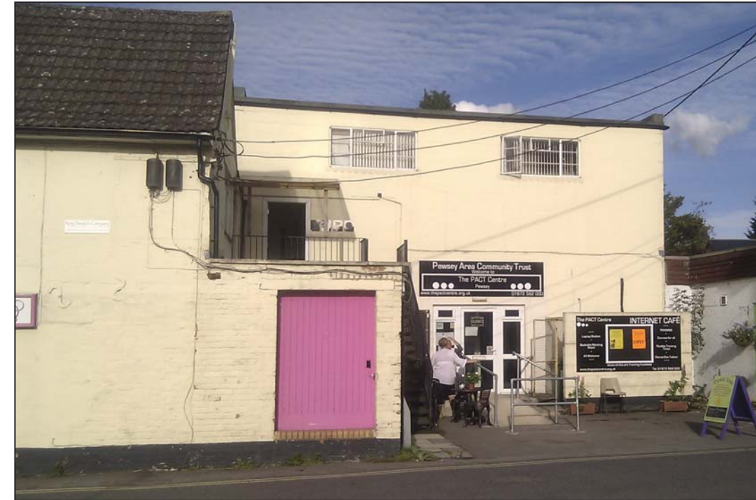
5 The south-west elevation of Block 2, looking north-east, Block 1 to right
