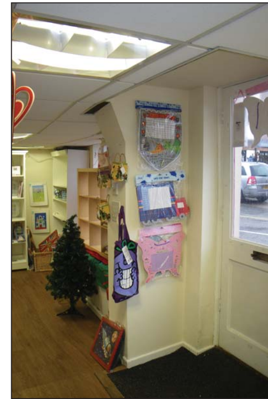
8 The enclosure of a probable structural timber in the shop looking south
