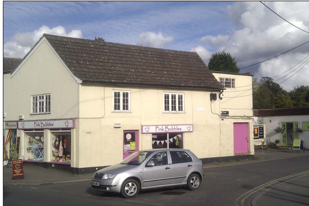
3 General view to east, Block 3 in foreground on Old Ford Lane
