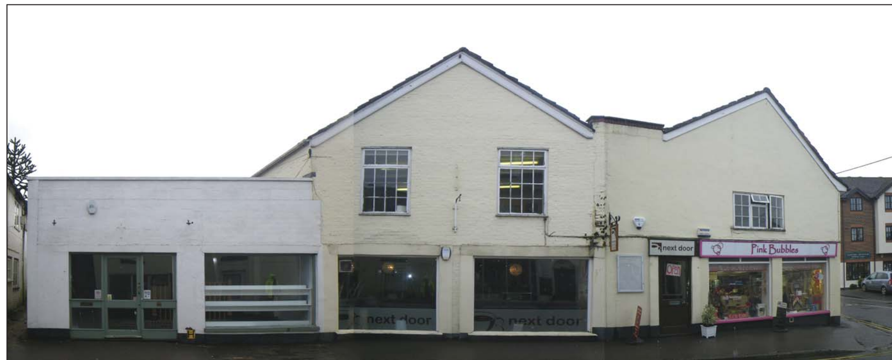
4 Composite view of north-west elevation of Blocks 2 and 3 on Pewsey High Street
