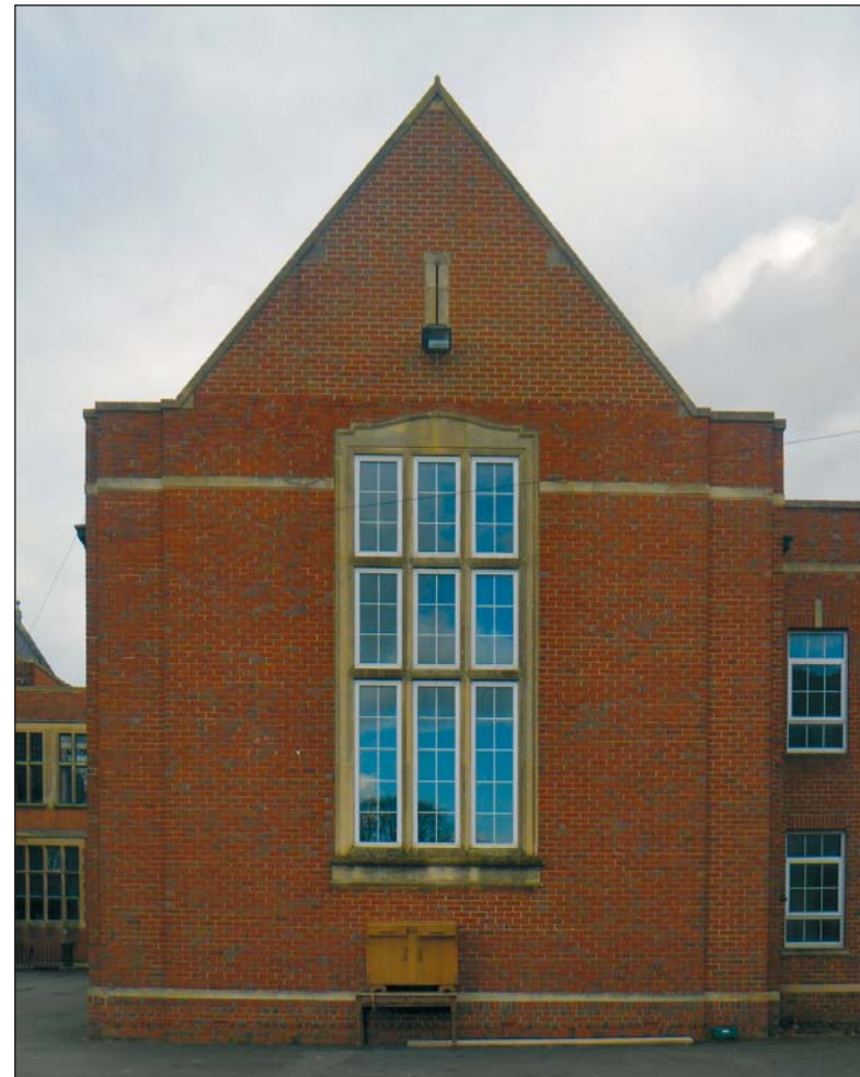
18 The south end of the Period 3 hall, looking north
