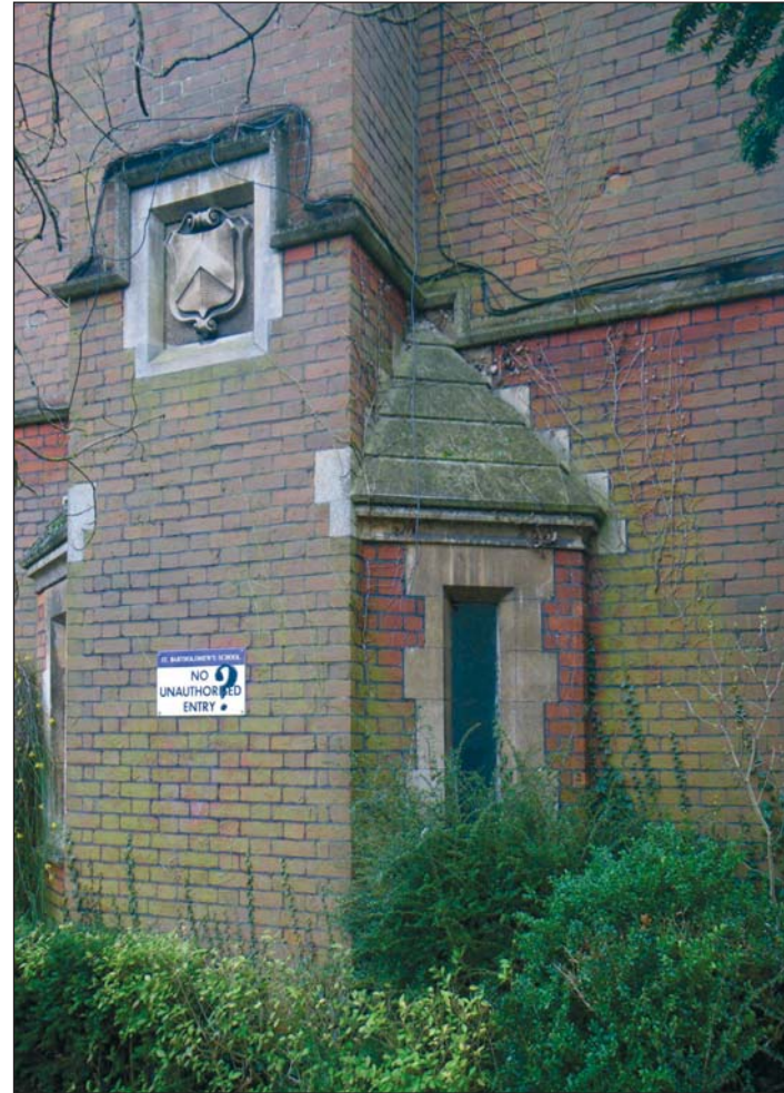
8 The exterior of the chimney stack in Fig. 6, at ground level, looking south-east
