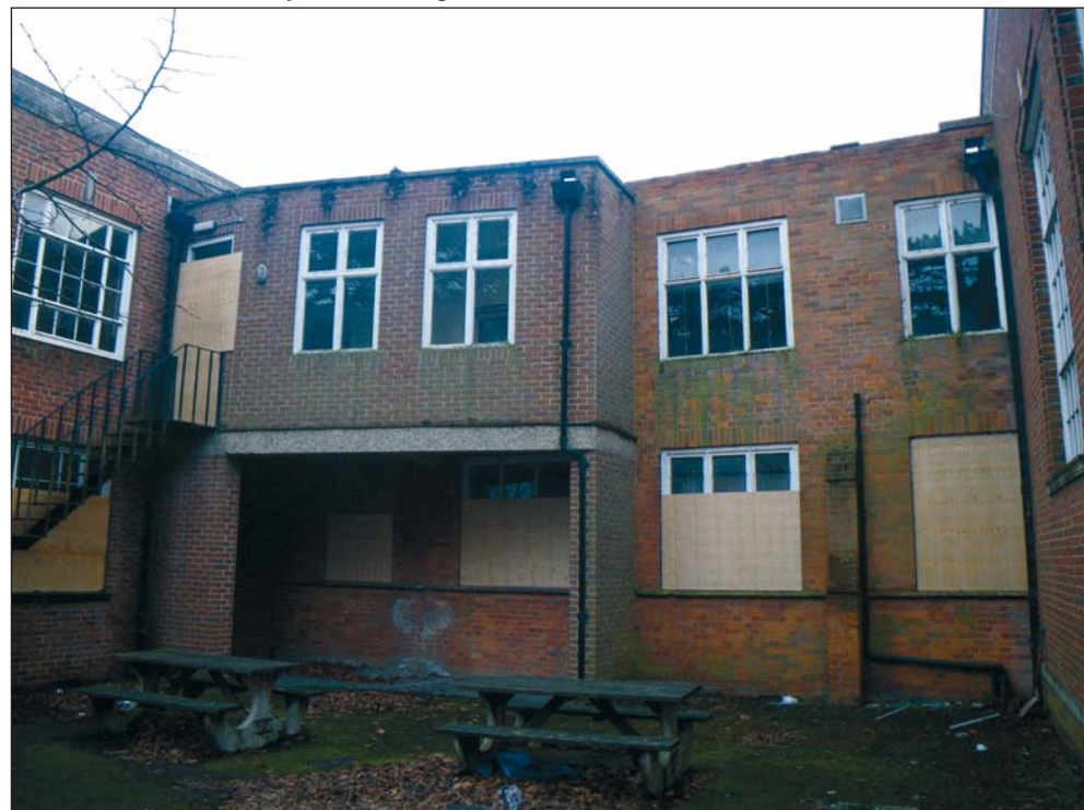
12 The eastern courtyard, looking south
