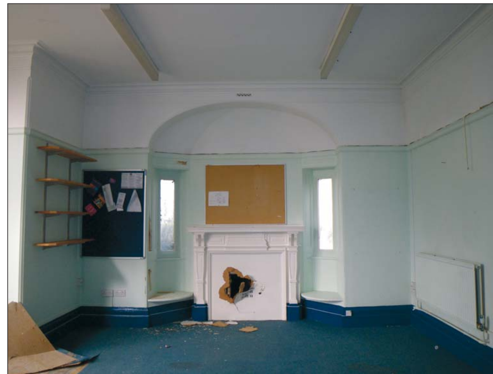
29 The Period 1 fireplace and chimney windows in room G10, looking north
