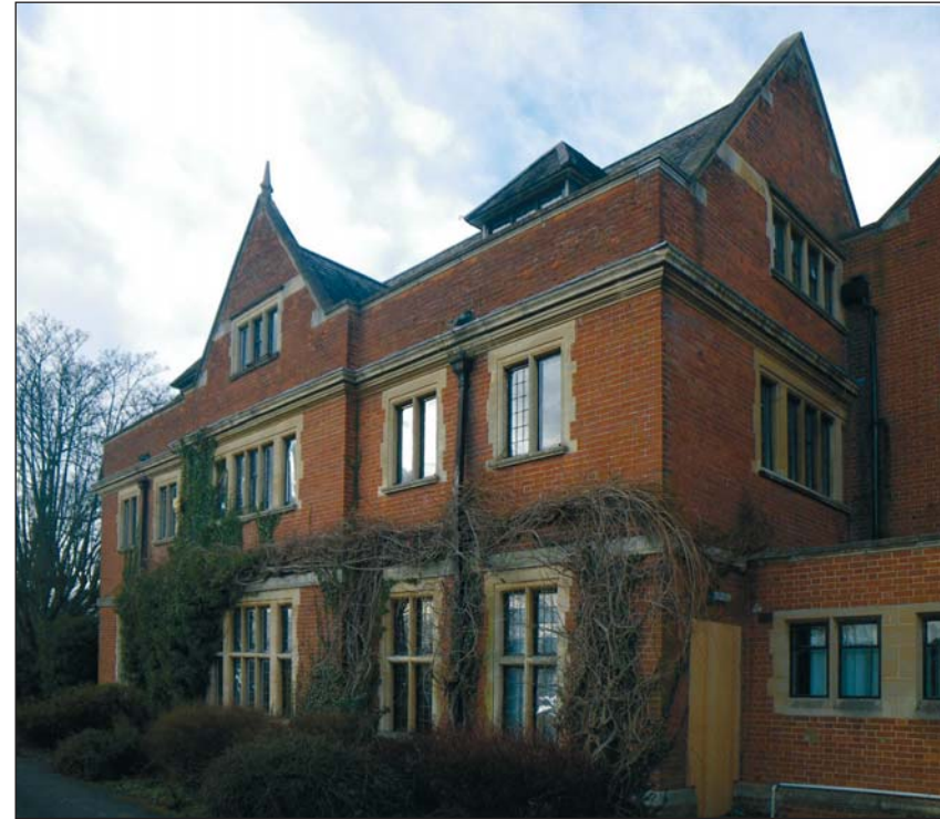
21 The south elevation of the Period 2 wing, looking north-west
