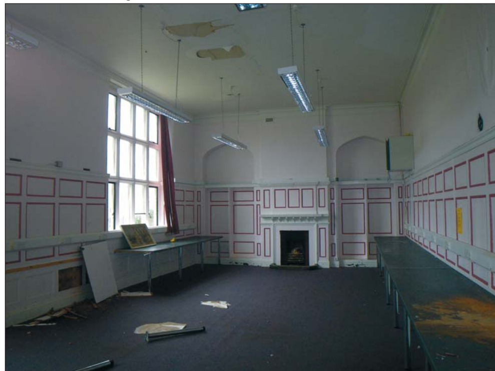
27 Room G8, looking east
