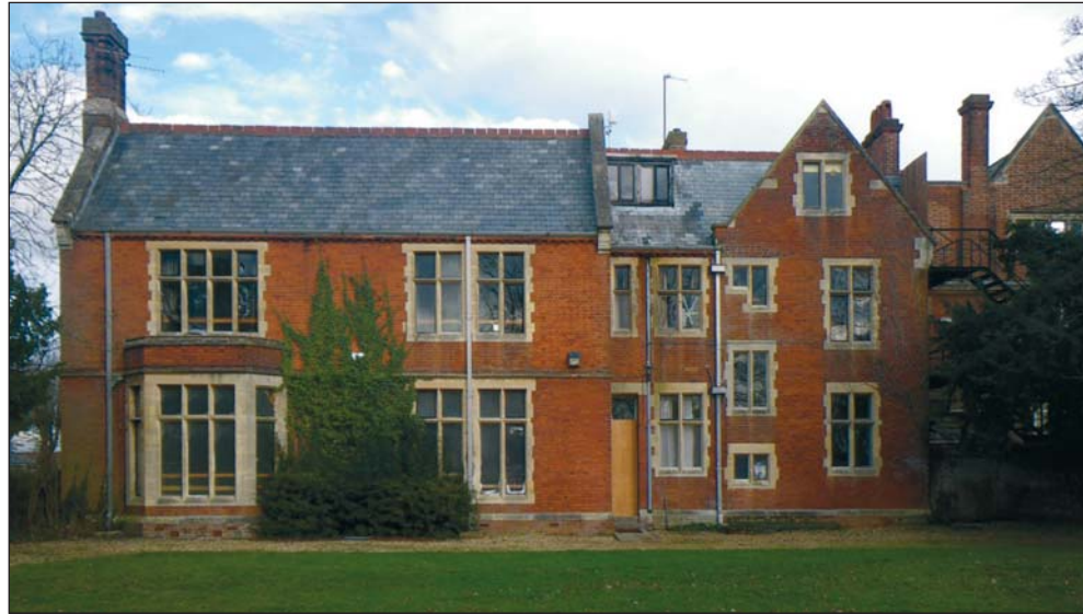
4 The west elevation, looking east
