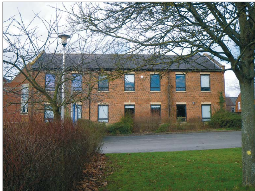
16 The Period 8 addition: the south elevation, looking north
