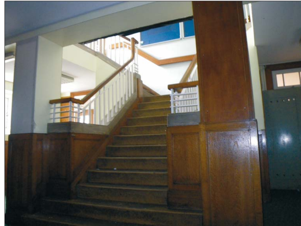
39 The Period 3 stairs ST1, looking south-east
