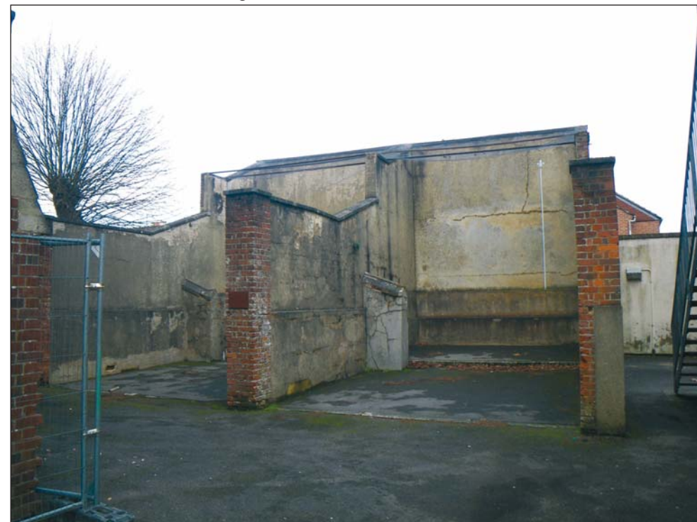
14 The Fives courts, looking east
