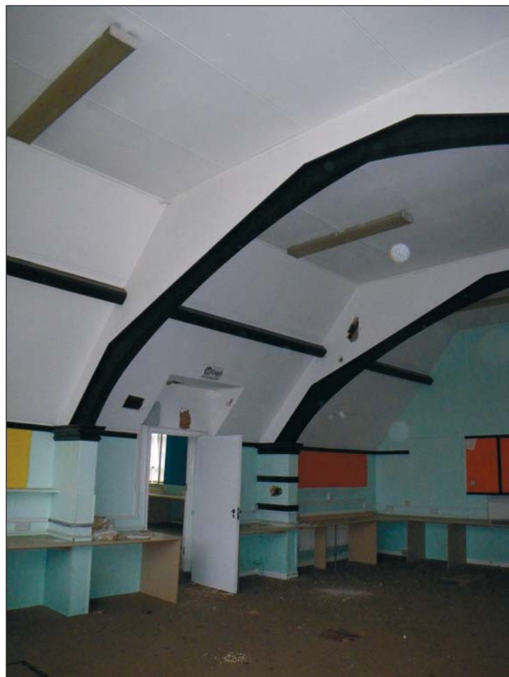
24 The upper part of the Period 1 hall in room F1, with Period 3 ceiling and inserted floor, looking south-east
