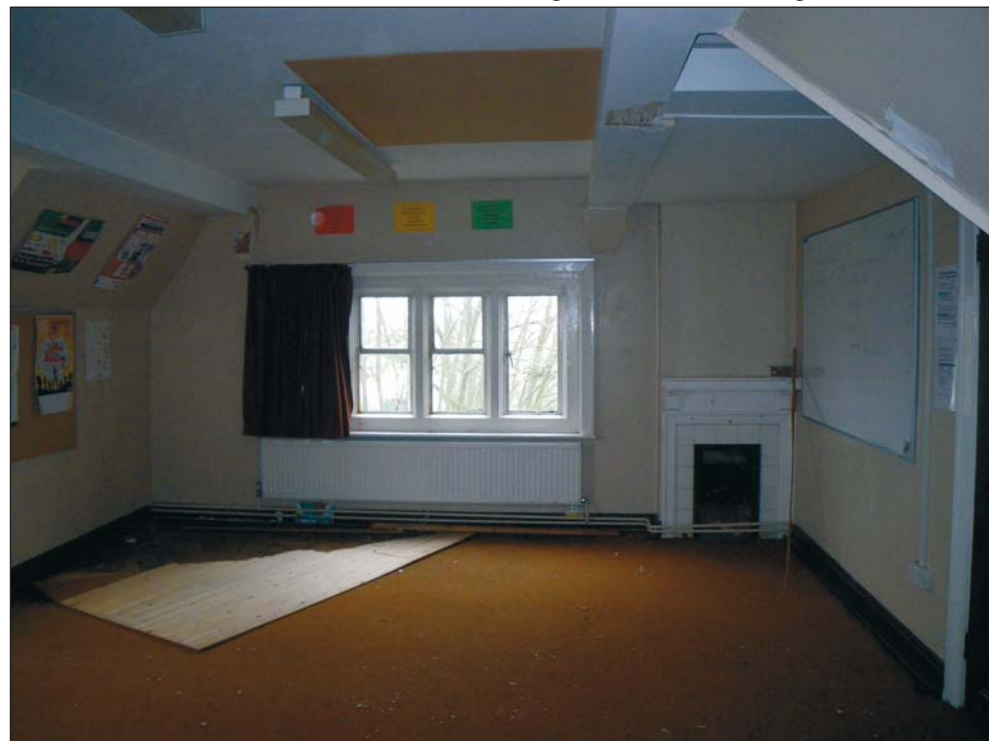
35 The second floor of the Period 2 south wing; room S17a, looking west
