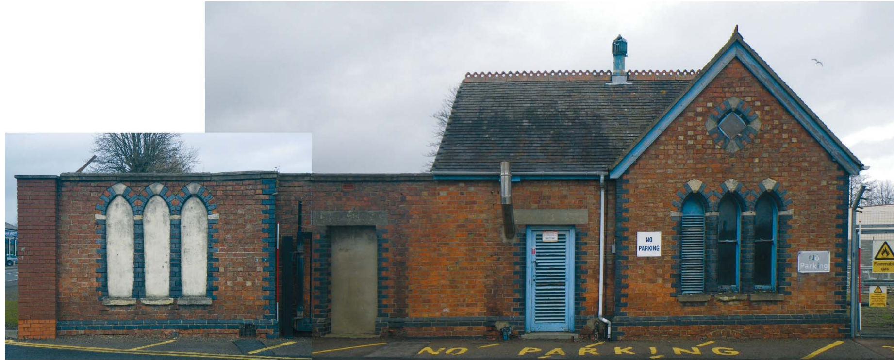
Fig. 8 The south elevation of the gate lodge BD1 (Scale 2m)
