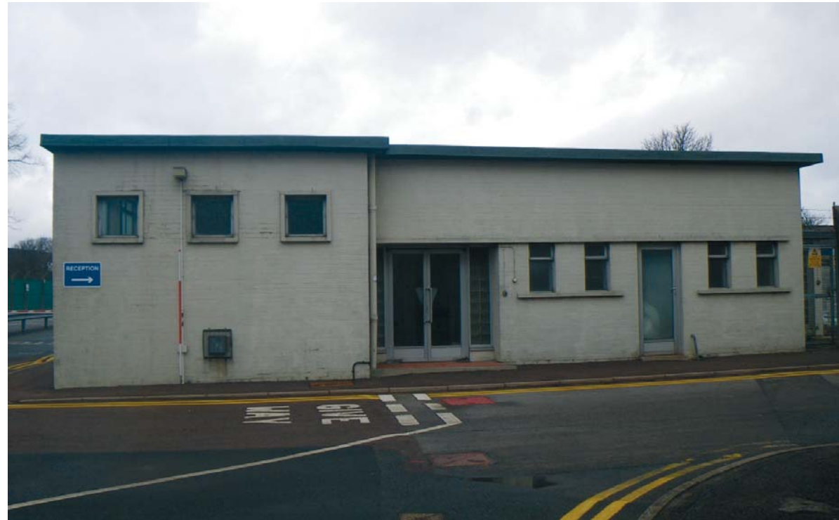
Fig. 12 The east elevation of BD2 (Scale 2m)
