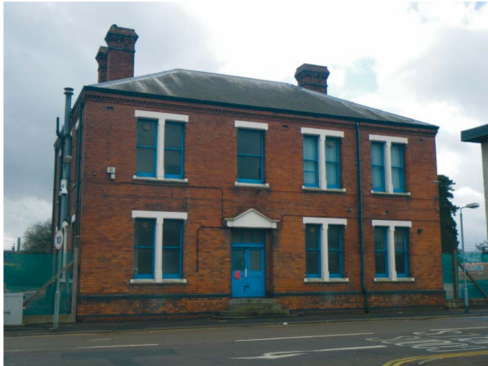
Fig. 22 The north elevation of BD3, looking south-west
