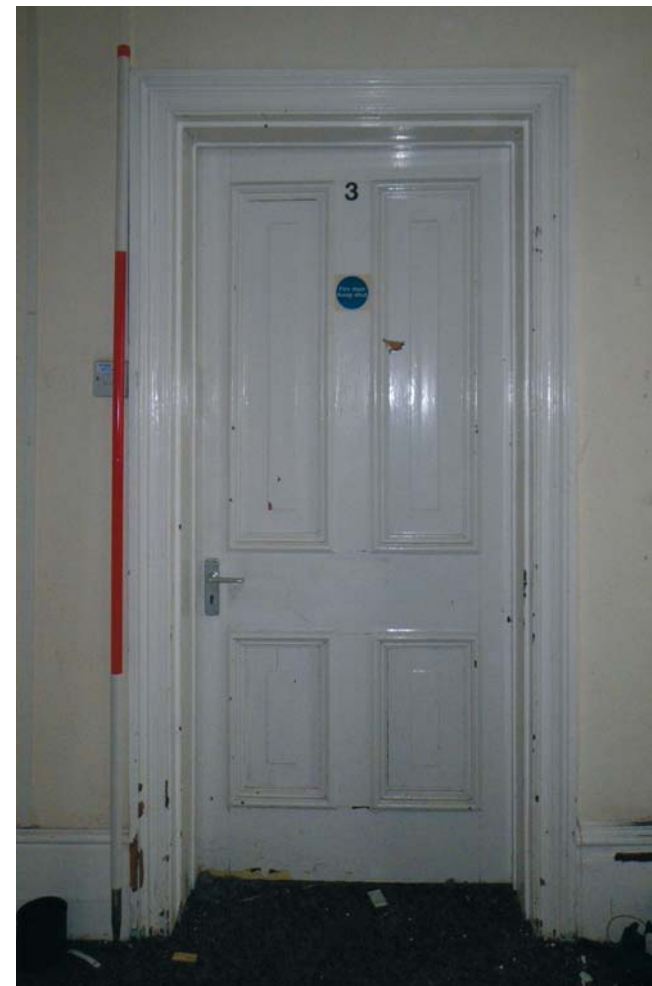
Fig. 21 A typical internal door and architrave on the ground floor of BD3 (Scale 2m)
