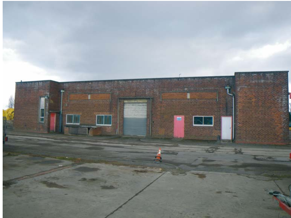
Fig. 32 The west elevation of BD5, looking north-east (Scale 2m)
