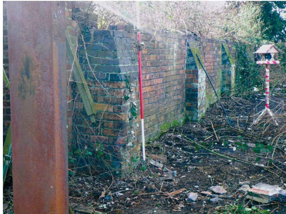
Fig. 28 The north wall and north-east corner of BD4.1 looking west, showing the buttresses (Scale 2m)
