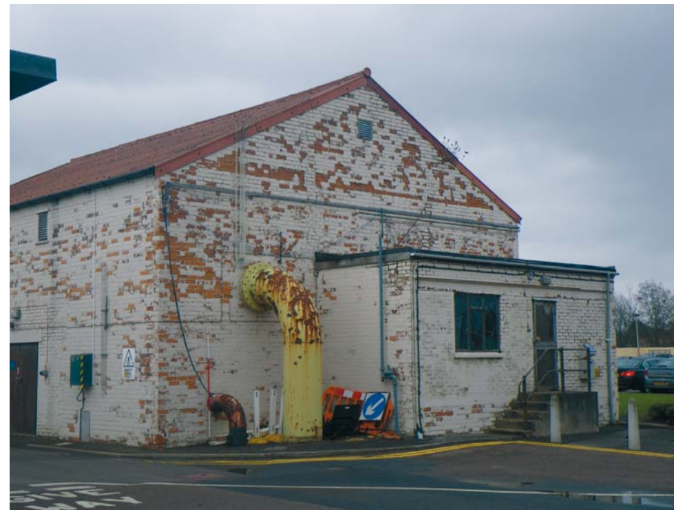
Fig. 46 BD6 looking north-east (Scale 2m)
