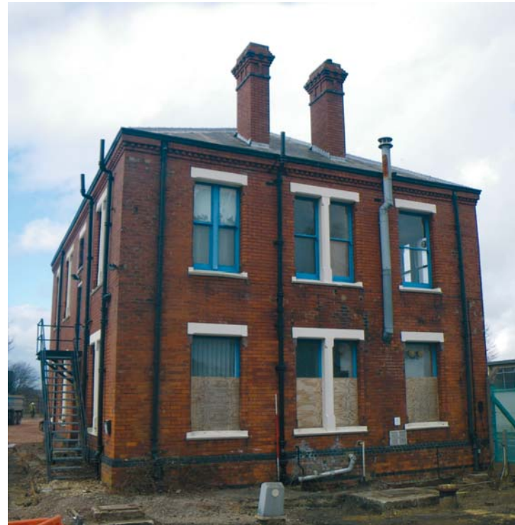
Fig. 23 The east elevation of BD3, the fenestration reflecting the smaller rooms and the WC on the ground floor (Scale 2m)
