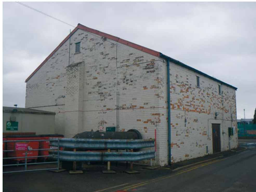
Fig. 45 BD6 looking south-east (Scale 2m)
