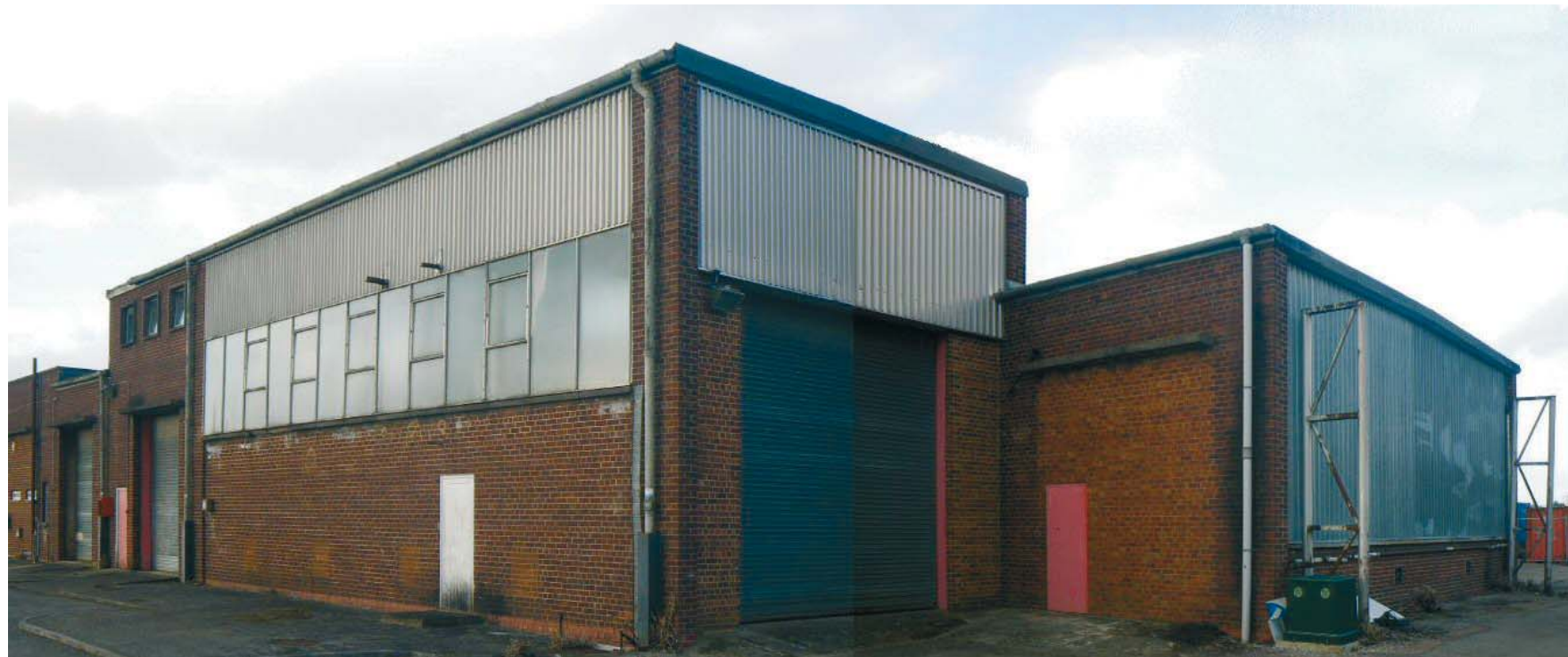
Fig. 34 The south and east elevations of BD5, looking north-west
