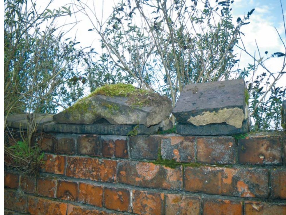
Fig. 27 The fired brick copings of most of the walls in BD4
