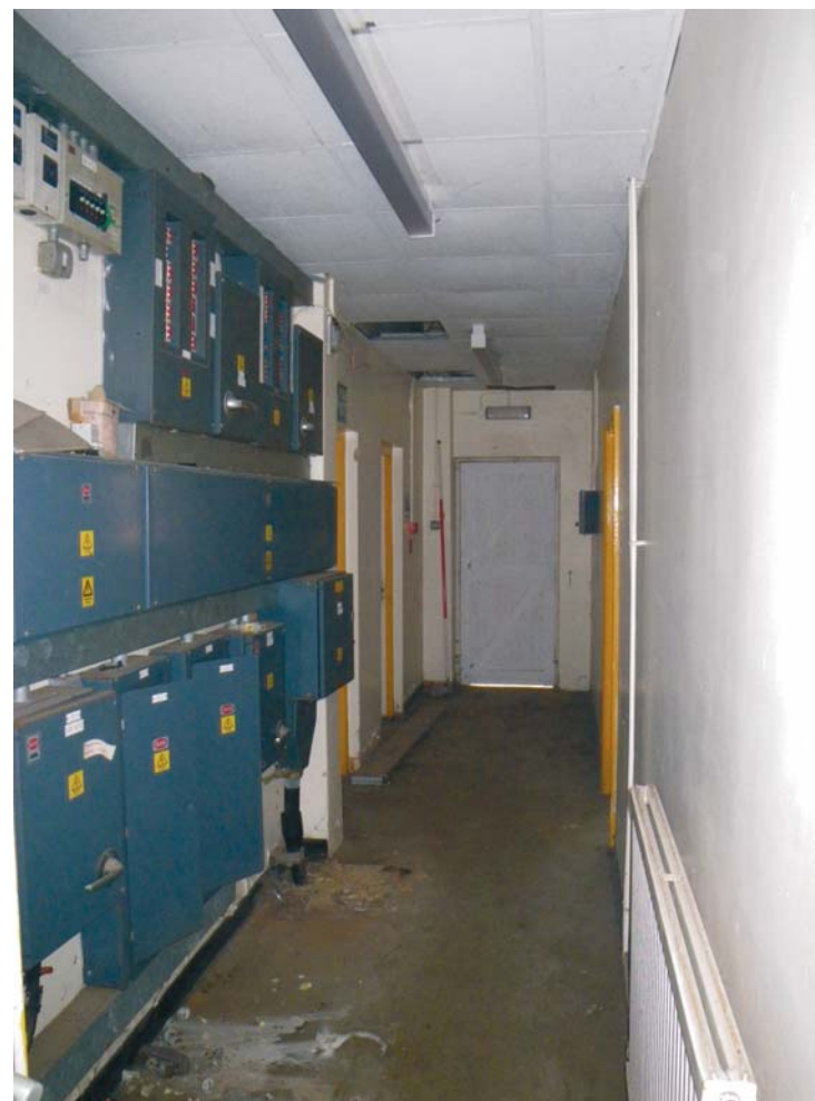
Fig. 36 The corridor in the south-west corner of BD5, looking west, showing the two original doors to the vehicle bays on the left, the inserted door, by the scale, and the added office wall on the right (Scale 2m)
