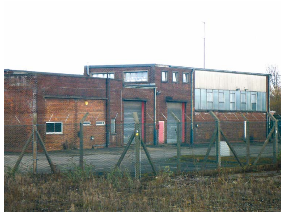
Fig. 33 The south elevation of BD5, looking north-east
