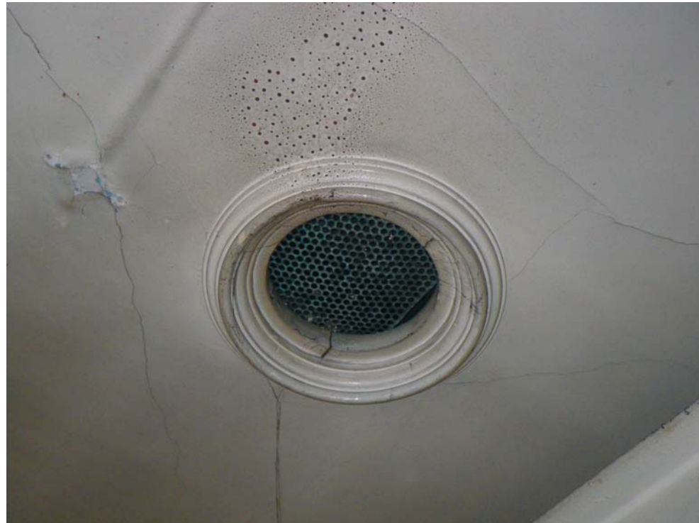
Fig. 9 The ceiling vent in the eastern room of BD1
