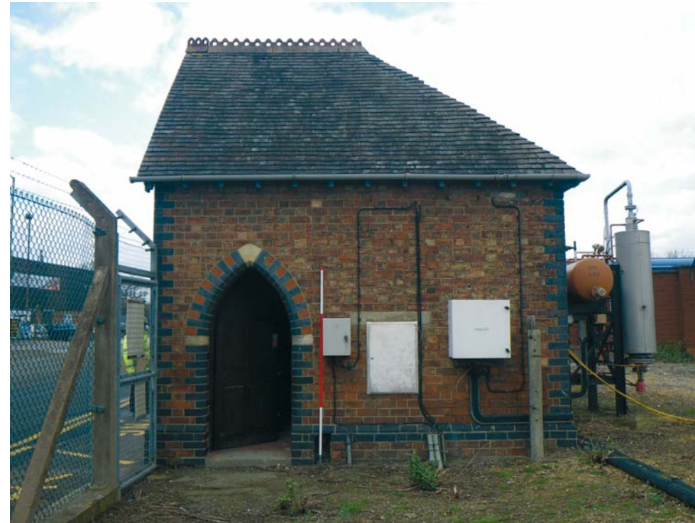
Fig. 10 The east elevation of BD1 (Scale 2m)
