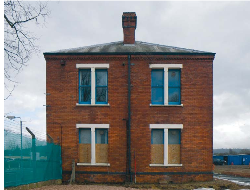
Fig. 25 The west elevation of BD3 (Scale 2m)
