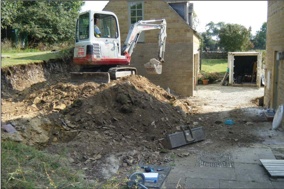
General working shot looking south towards garage
