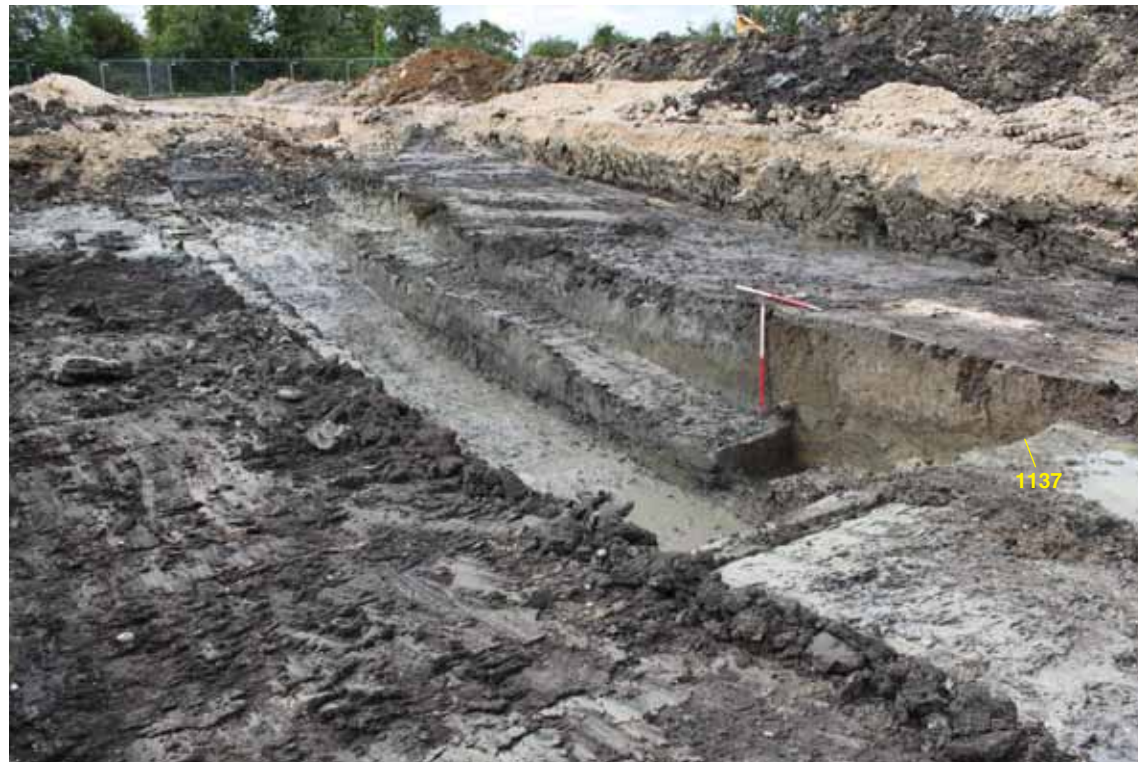
Full profile through moat ditch 1137 after removal of modern dump deposits looking north-west (2 x 1m scale)
