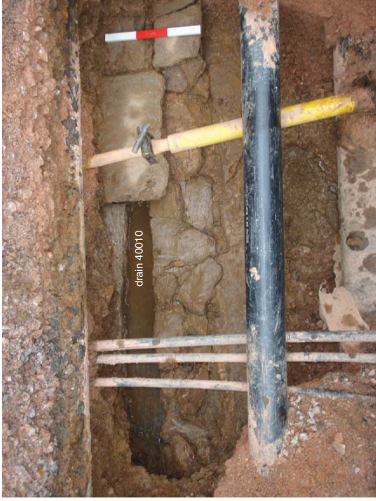
General view of drain 40010 looking north (0.3m scale)
