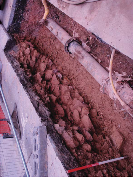
General view of wall 17002 looking north (1m Scale)
