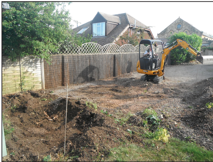
View of groundworks, looking north-east
