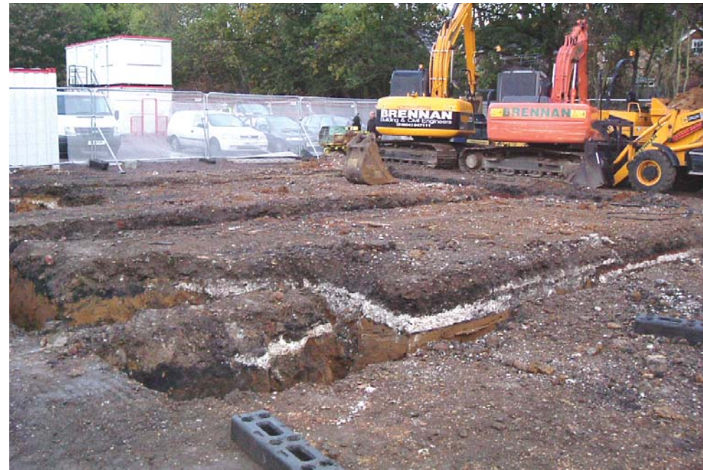
The foundation trench for House F2, looking north-west
