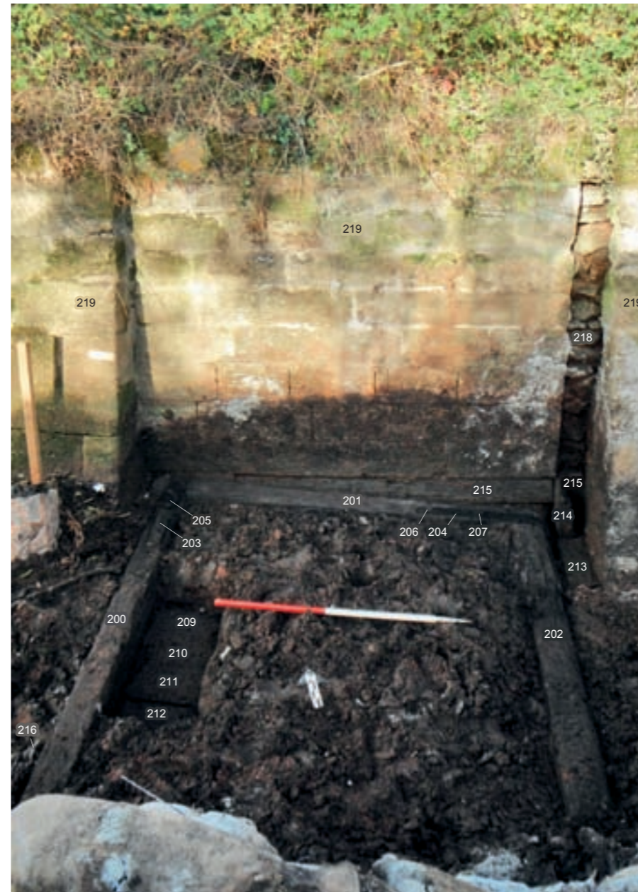
Stop gate remains, western side of swing bridge, looking north (1m scale)
