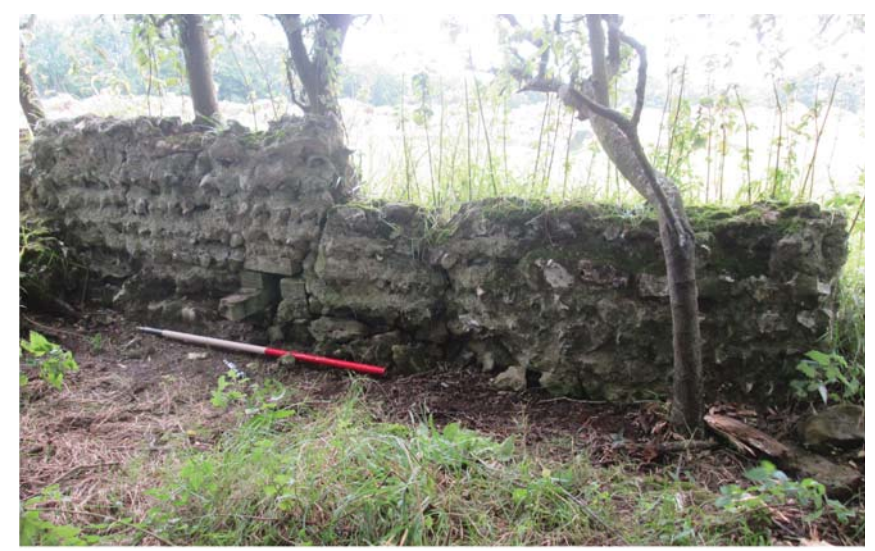
Flint wall adjacent to Trench 12, looking south-west (1m scale)
