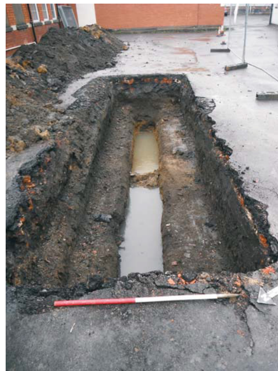
Trench 2, looking south-east (scale 1m)
