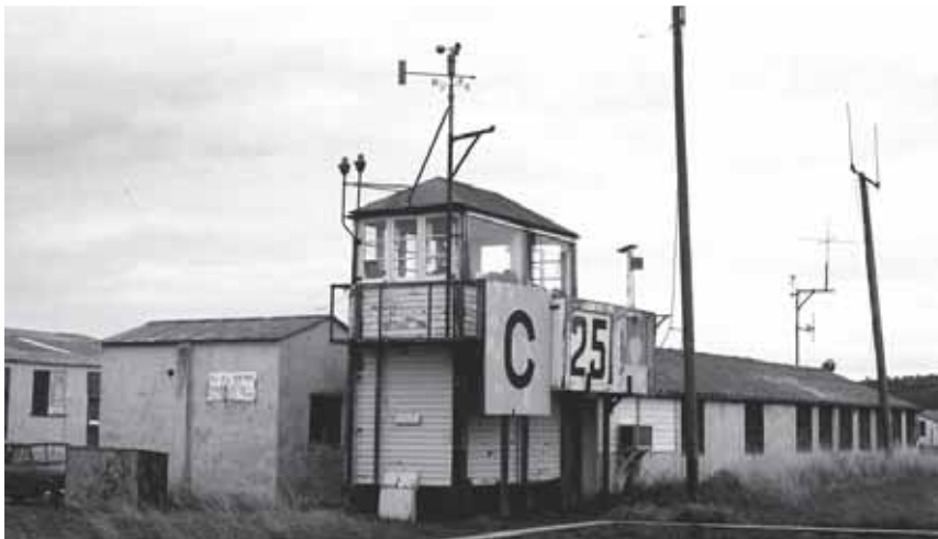
Plate 3: Control tower, (Bldg.53), as seen in September 1982
