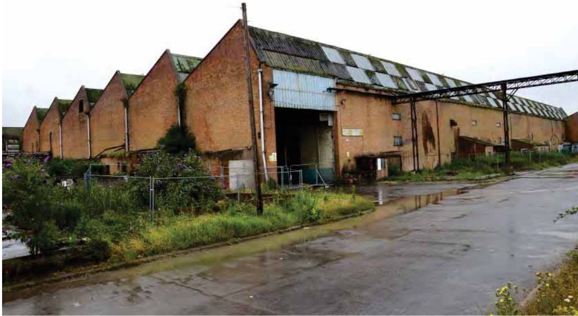
Plate 54: Shop 7 – view looking south-west showing the one internal loading bay
