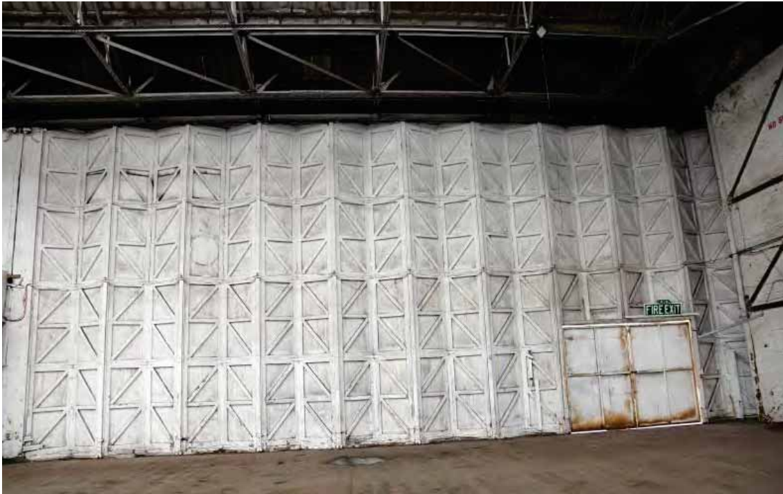
Plate 40: Dope Shop – interior view of the Esavian doors
