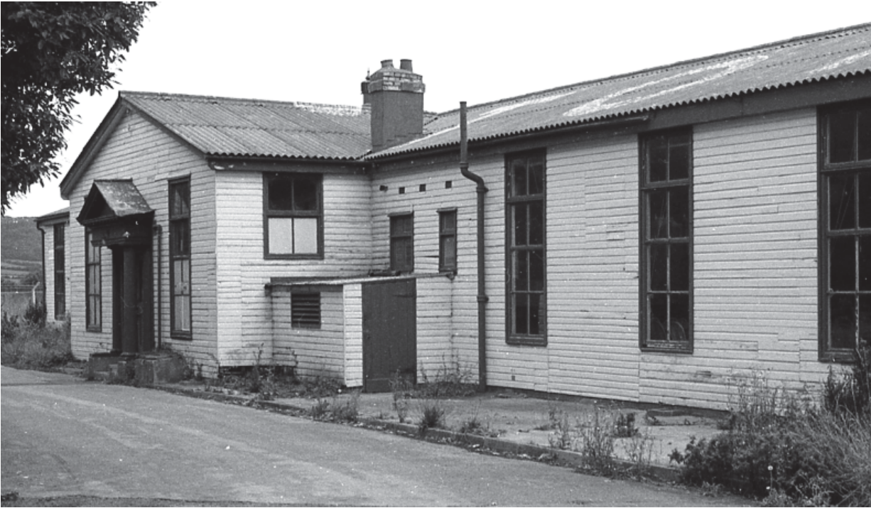
Plate 7: Station offices, canteen and officers' mess, (Bldg.5) – view of the entrance elevation, September 1982. This was formally the passenger terminal building.
