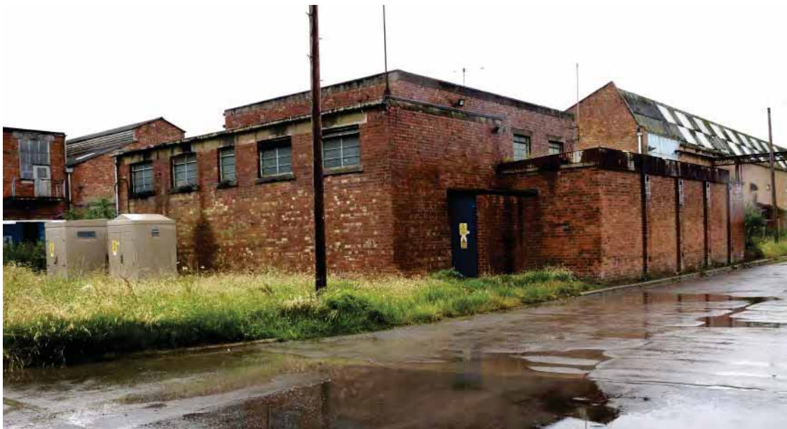
Plate 42: Power house – view from north
