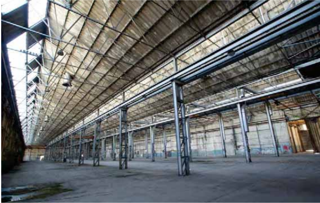
Plate 56: Shop 7 – clearly showing the uncluttered roof trusses
