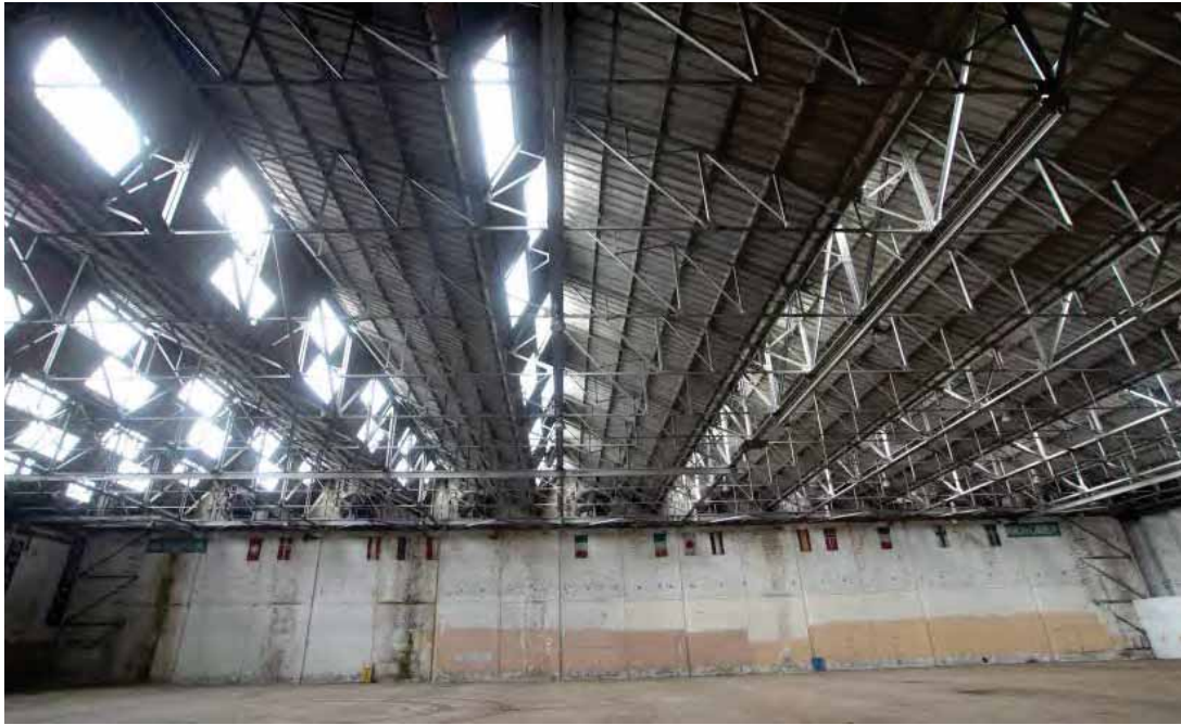
Plate 38: Dope Shop – interior view looking at the eastern side wall
