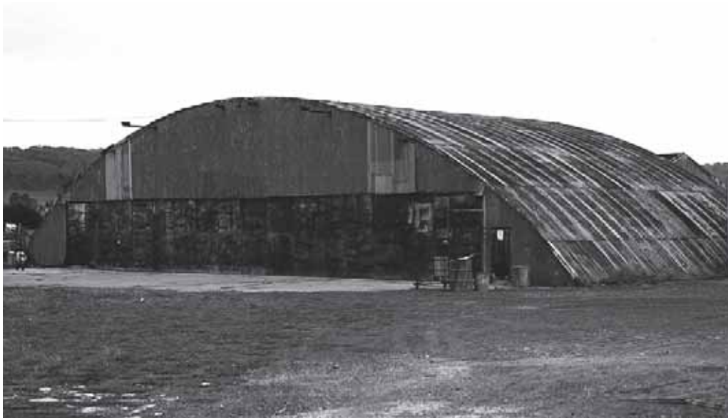
Plate 1:9 Blister Hangar, (Bldg.128), September 1982
