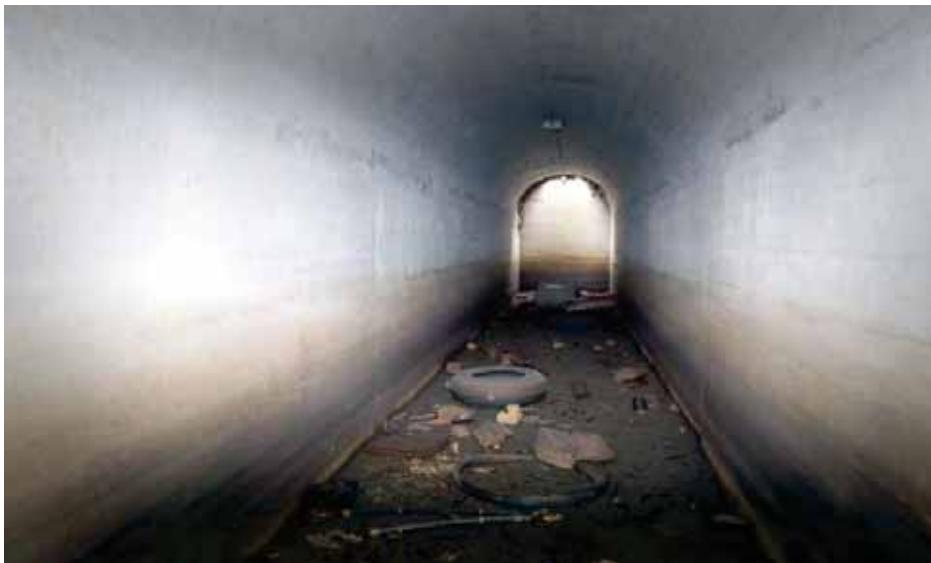
Plate 82: Air-Raid Shelter, (Bldg.142) – view looking towards the emergency exit
