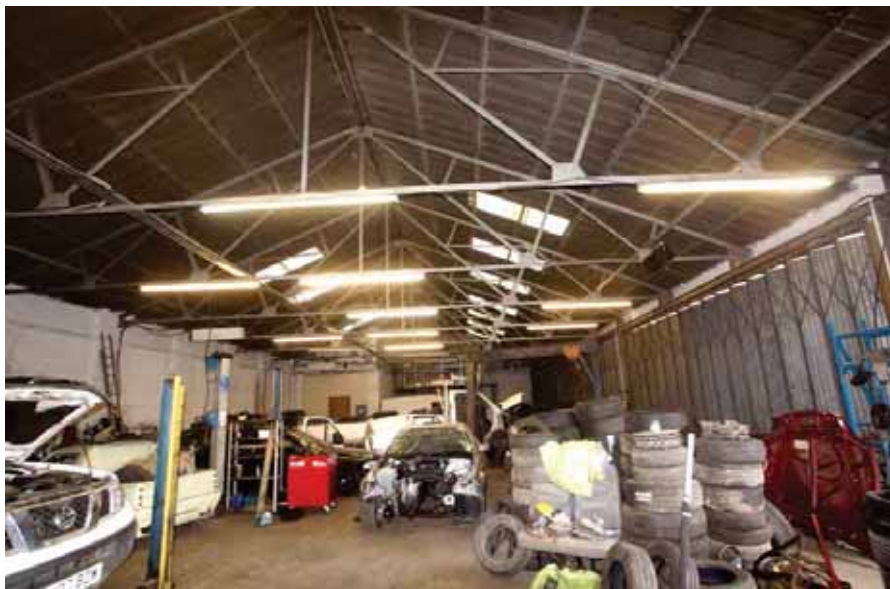
Plate 52: Interior of the garage
