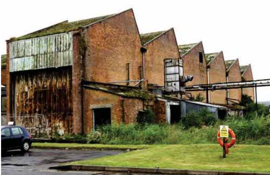
Plate 59: Shop 7 – view looking west at an external loading bay
