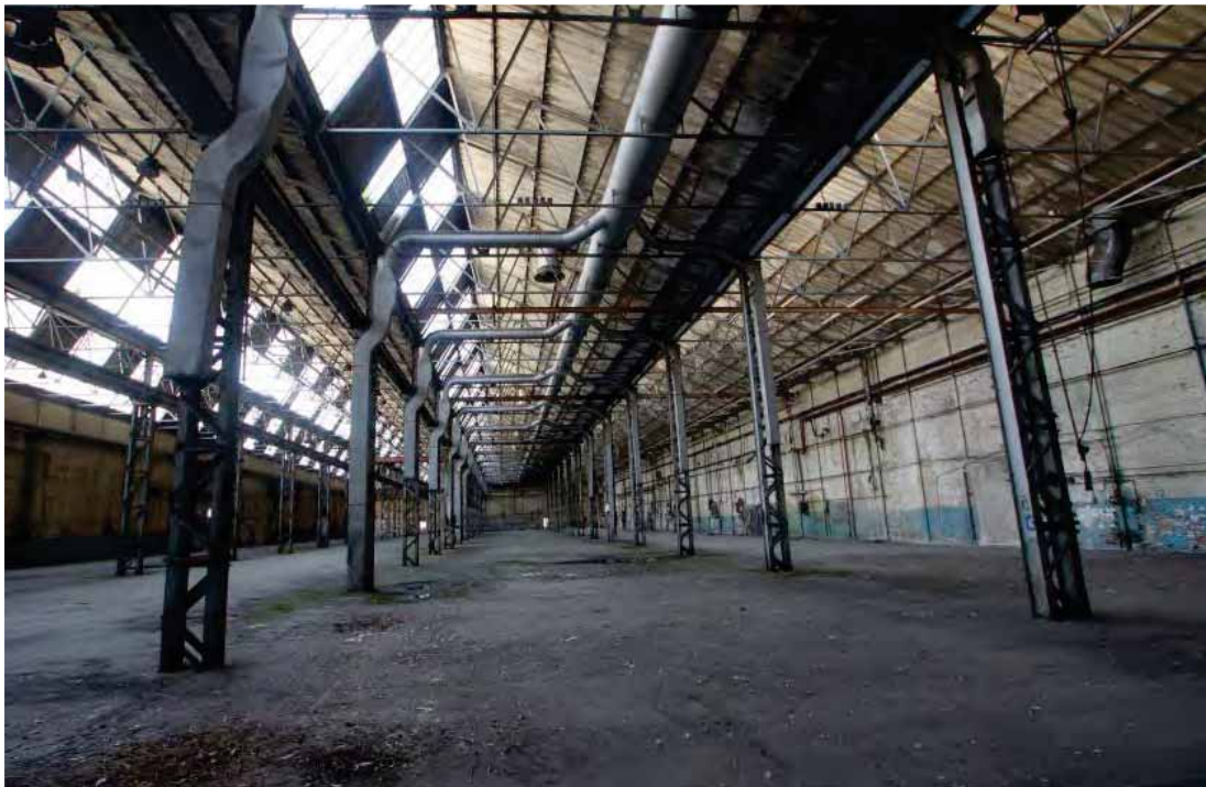
Plate 55: Shop 7 – view looking east inside the main area
