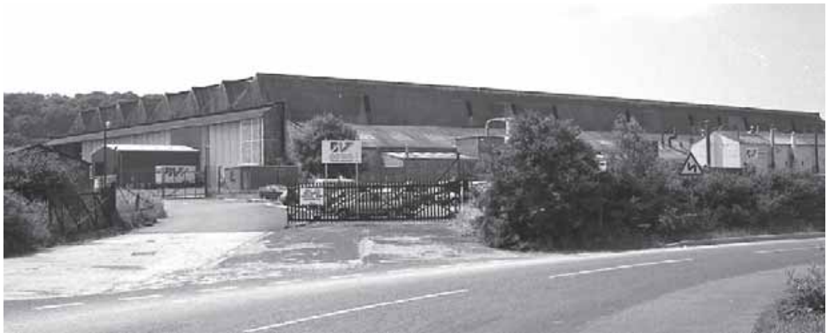
Plate 20: No.1 Erecting Hall at Banwell – wide angle view, 1990
