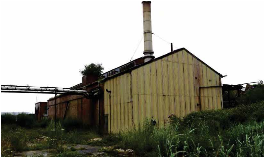
Plate 45: Boiler house extension
