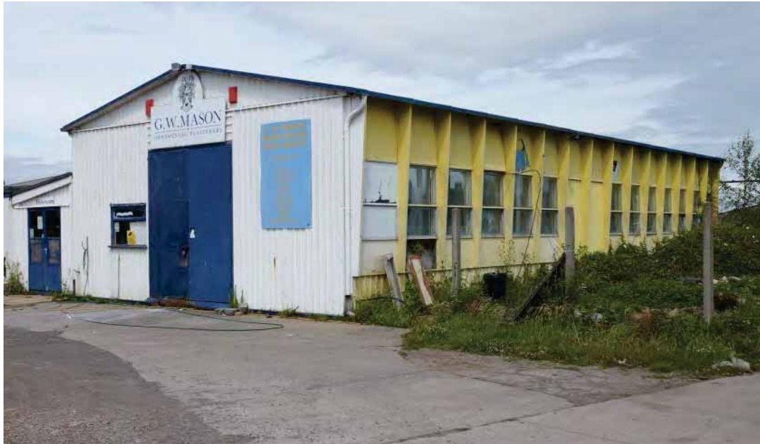
Plate 78: The 15-bay aluminium Mark I school building with triangular fins
