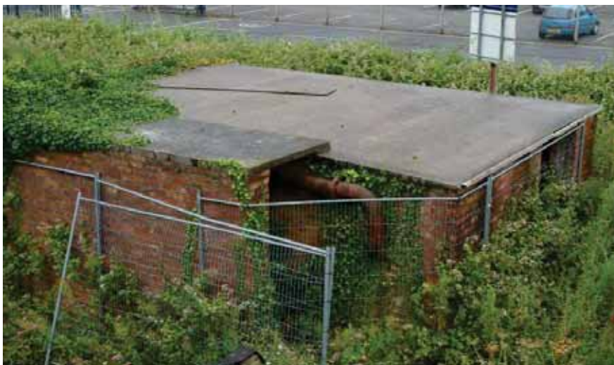
Plate 83: The air raid shelter viewed from the first floor of the admin building
