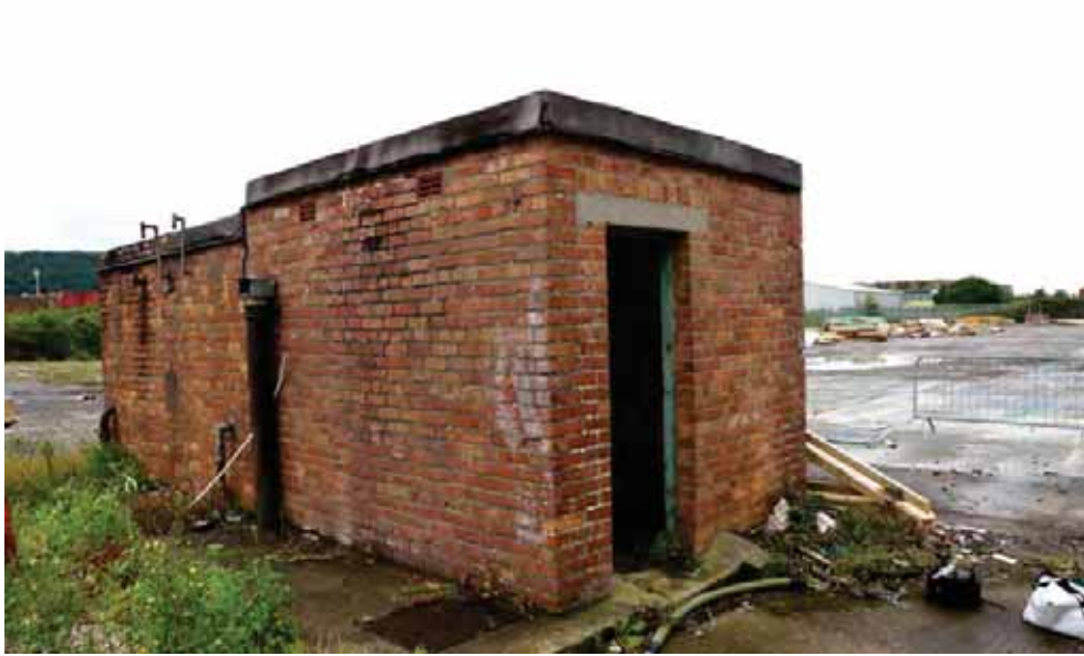
Plate 28: Plate 1: Pump House, building 102, July 2015
