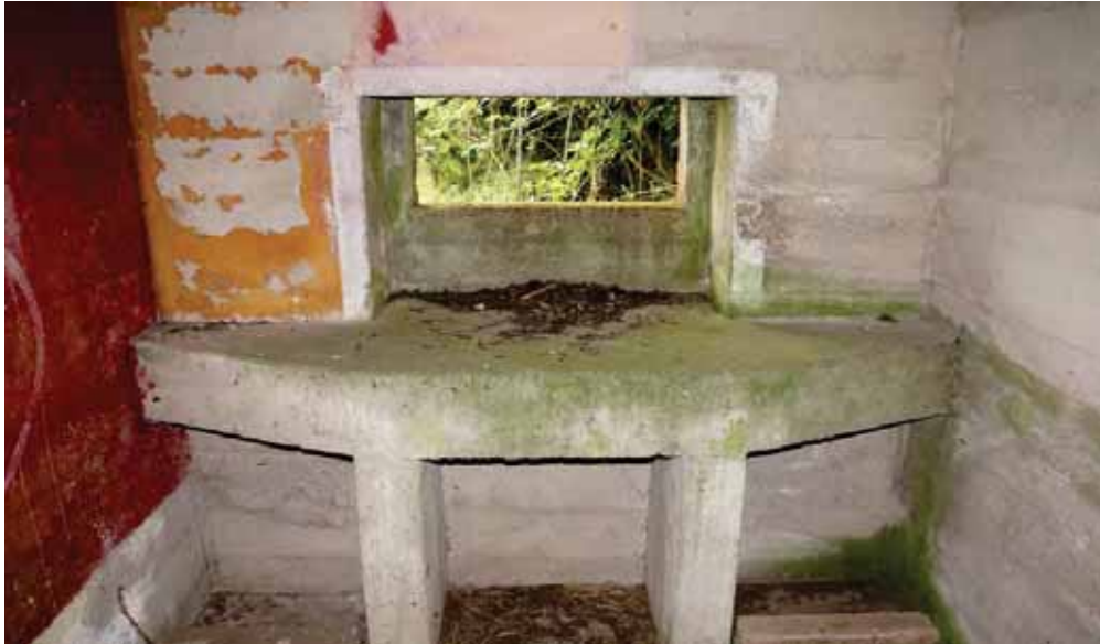
Plate 14: Pillbox, (Bldg.104) – interior view looking towards the airfield (July 2015)
