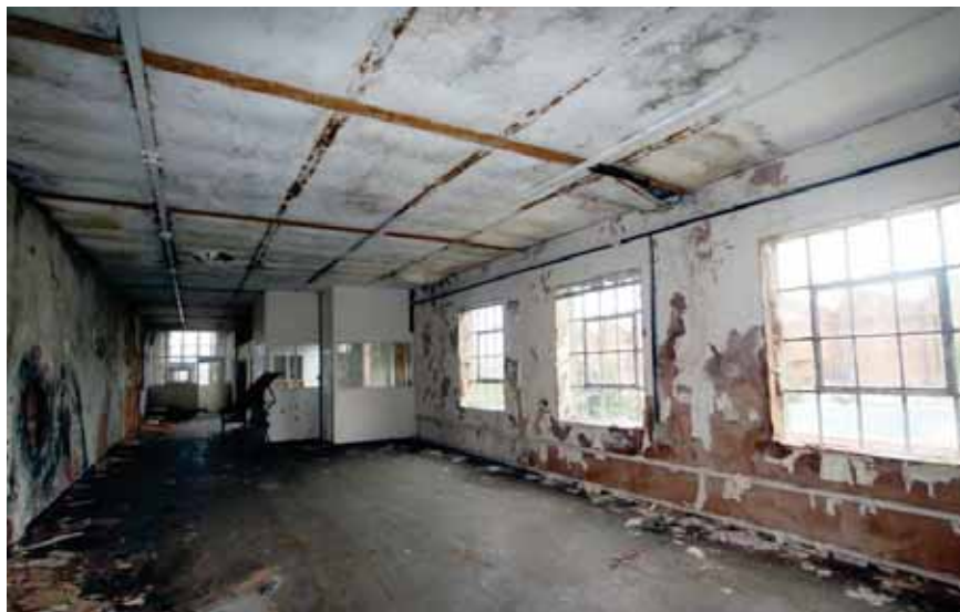
Plate 50: Interior of the first floor, July 2015
