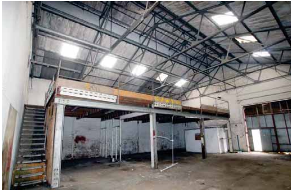
Plate 47: Interior of boiler house, July 2015
