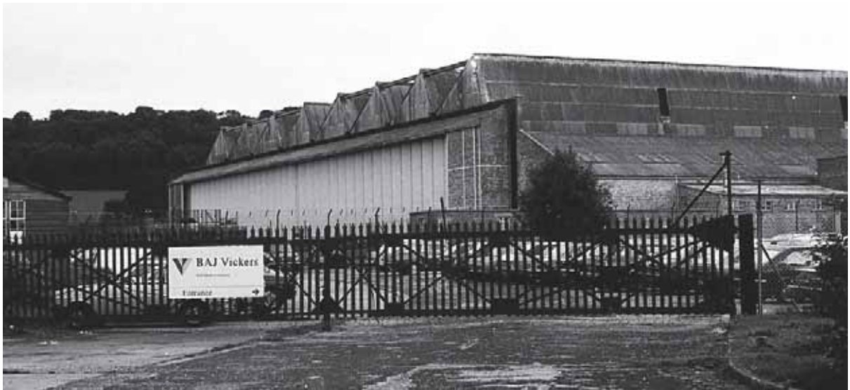
Plate 20: No.1 Erecting Hall at Banwell, September 1982
