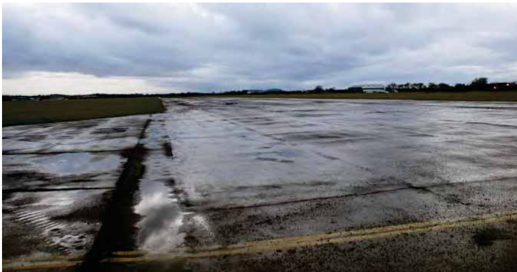
Plate 17: A rather wet concrete runway as seen in 2009
