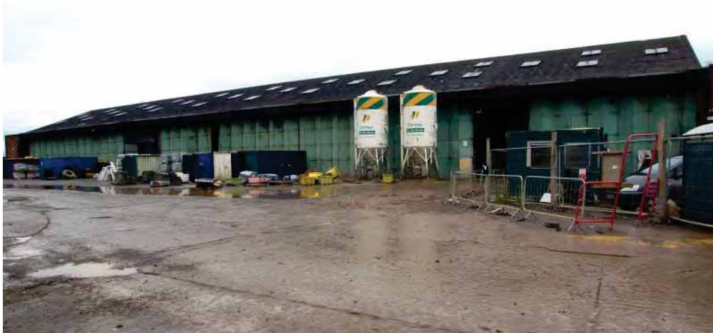
Plate 68: Front elevation of No.3 flight shed
