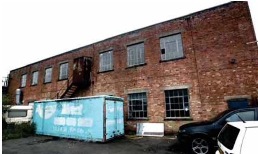
Plate 49: The front elevation of the boiler house offices / workshop, July 2015
