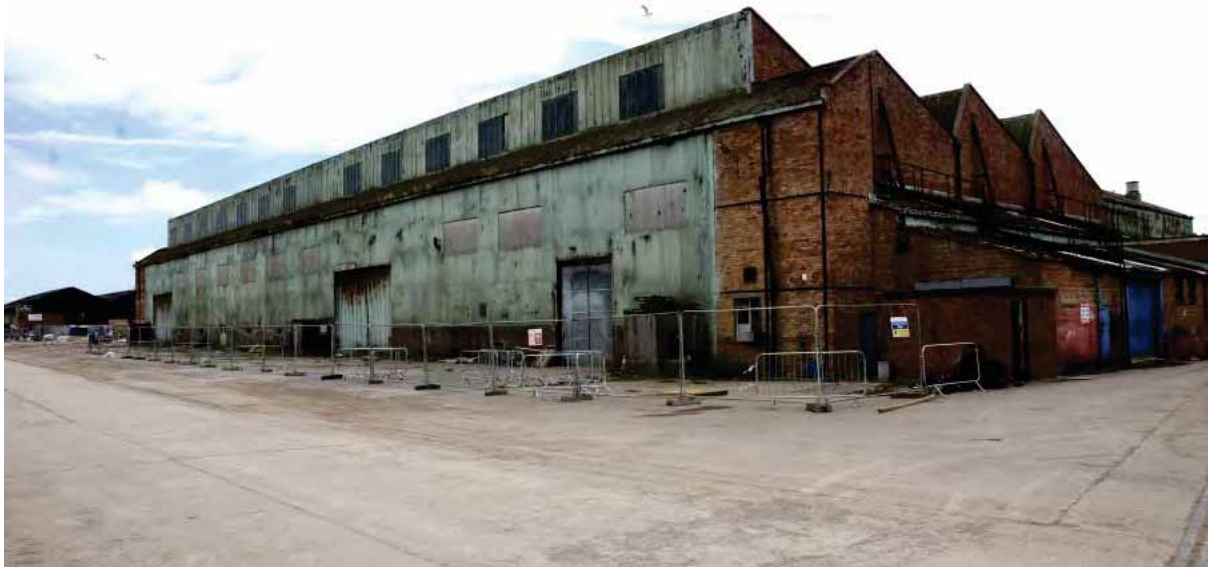
Plate 31: Flight Shed No.1 looking east
