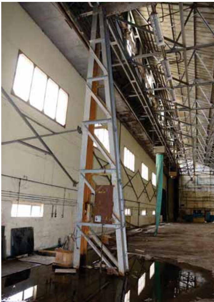
Plate35: Flight Shed No.1 – one of two internal central 'A' frames
