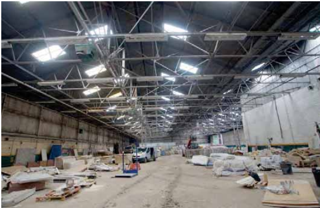
Plate 69: No.3 Flight Shed – interior view
