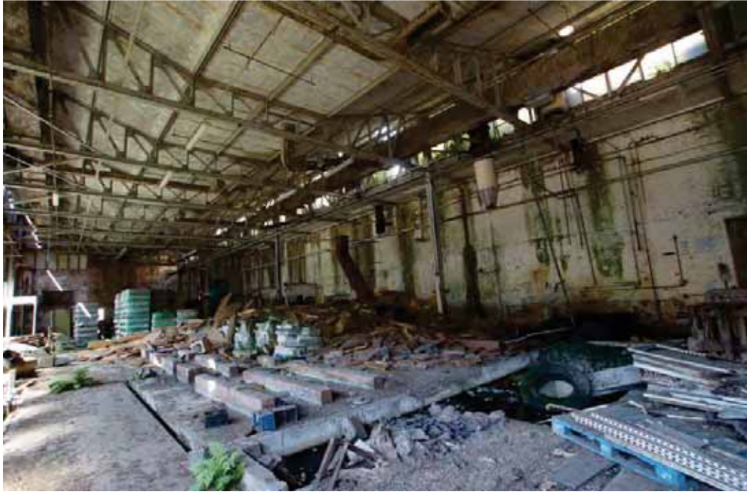
Plate 58: Shop 7 – treatment room annexe
