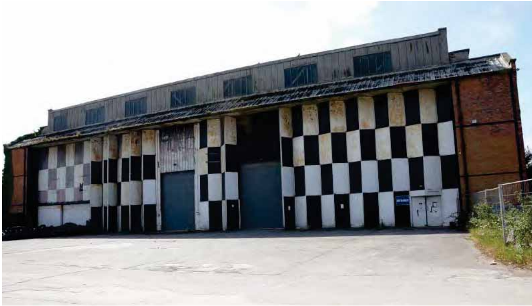
Plate 36: Dope Shop – north elevation
