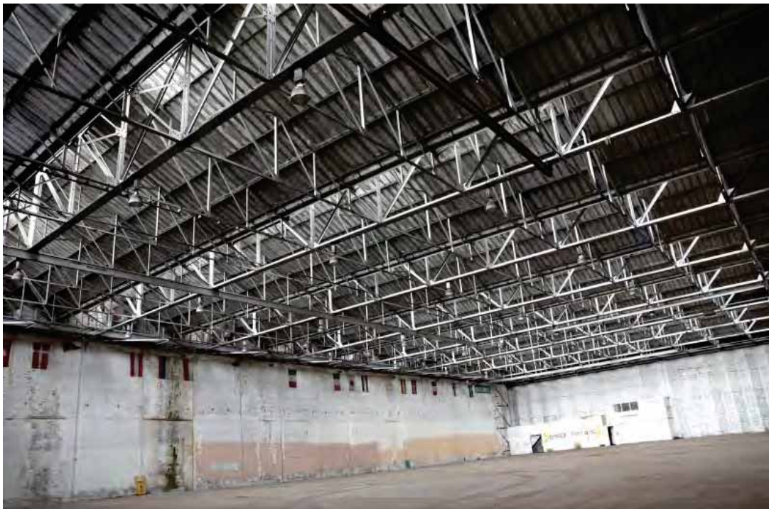
Plate 39: Dope Shop – interior view showing lattice roof girders and north-light trusses
