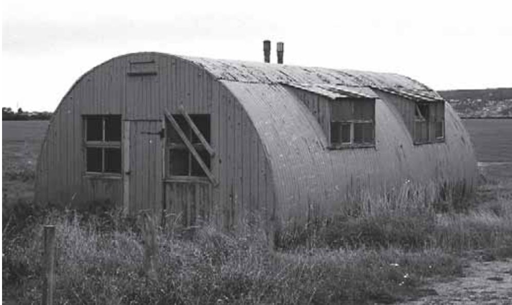
Plate 15: 16-ft-span Nissen hut on Defence Site No.3, (Bldg.76), September 1982
