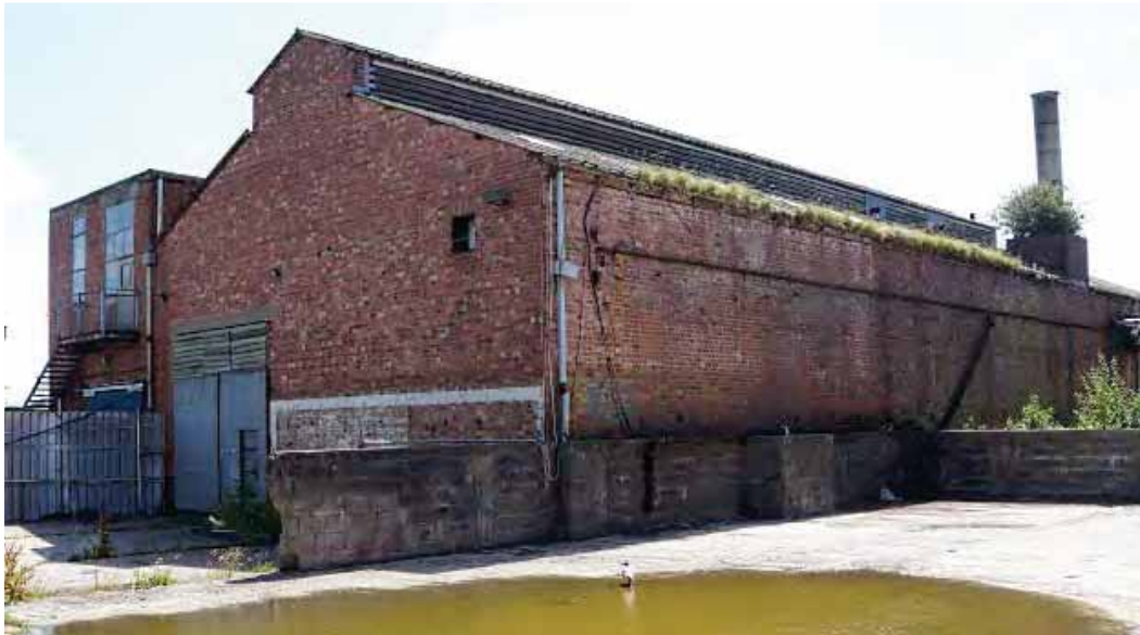
Plate 44: Boiler house looking south-east
