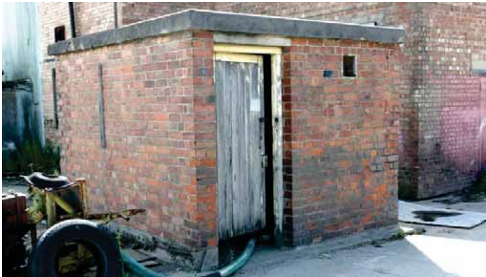
Plate 29: Sewage pump house, building 148, July 2015
