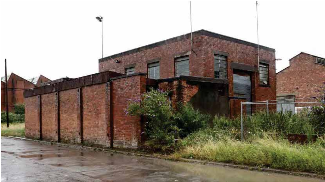
Plate 41: Power house – view looking at the blast wall of the transformer enclosure in front. The switch room is behind.
