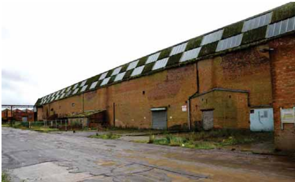
Plate 61: Shop7 a view looking south-east – note the camouflage paint
