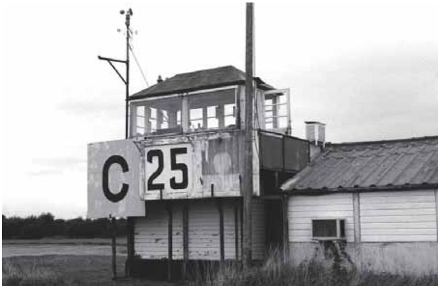
Plate 4: The wooden control tower still operational in September 1982
