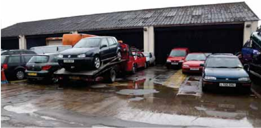
Plate 51: Garage – front elevation partly hidden by vehicles
