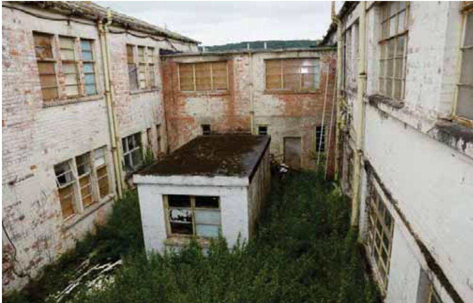
Plate 66: Administration Block – the original connecting corridor and an ancillary building
