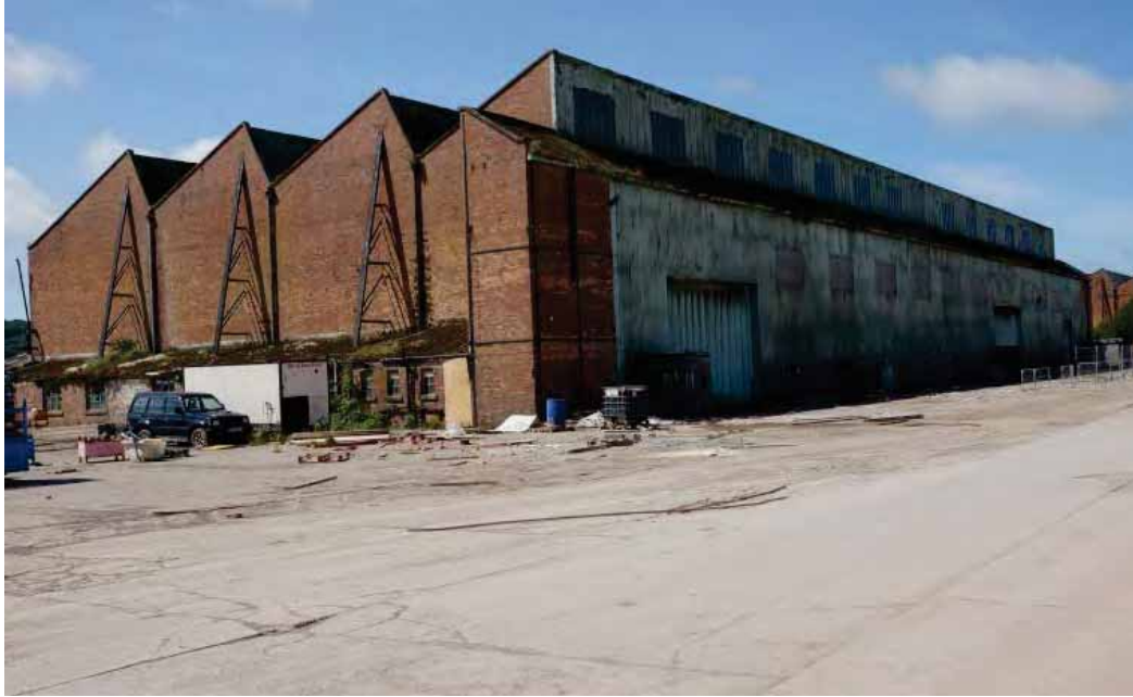
Plate 32: Flight Shed No.1 looking west
