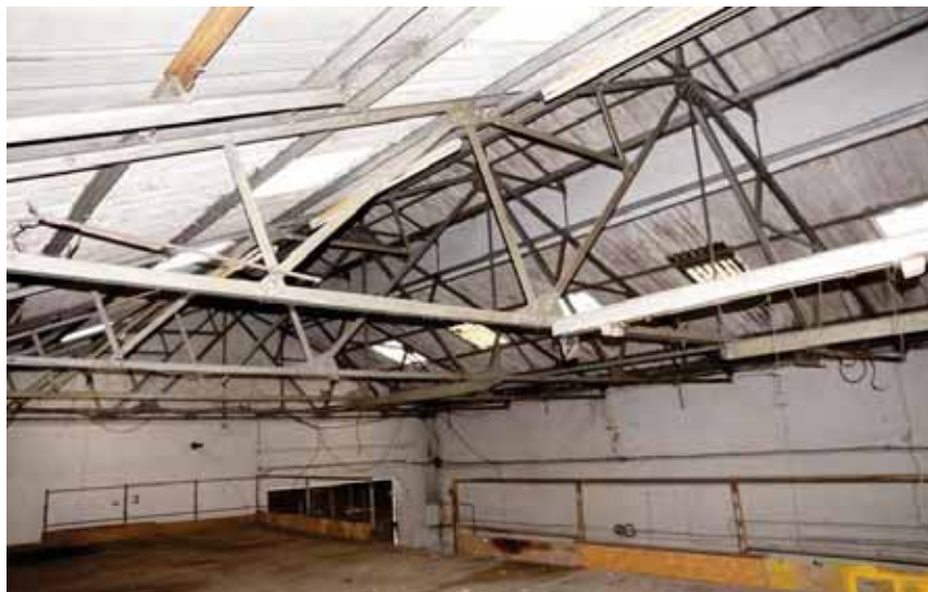
Plate 48: Boiler house Cargo Fleet roof trusses, July 2015
