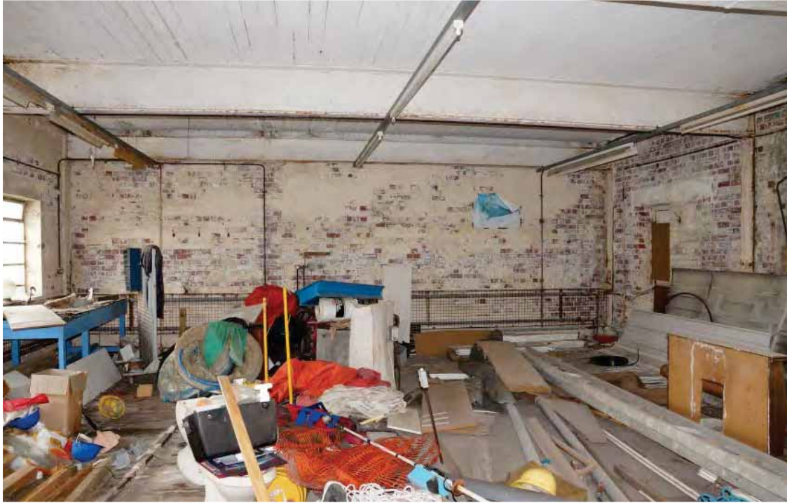
Plate 43: Power house – the first floor
