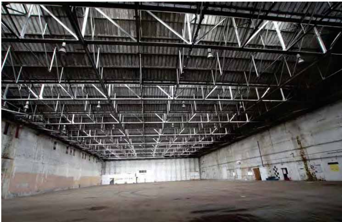
Plate 37: Dope Shop – interior view looking south
