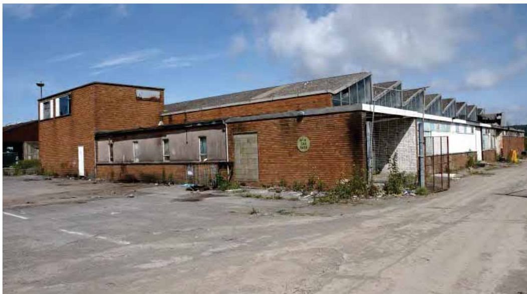
Plate 75: Design Office – view looking north-west
