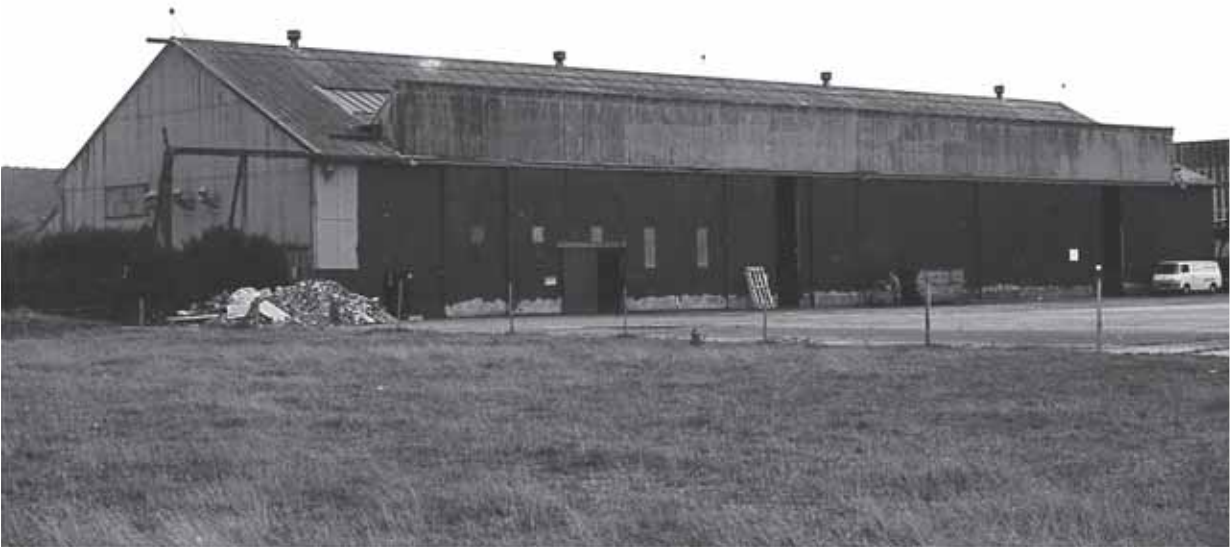
Plate 9: The original hangar, (Bldg.2), September 1982
