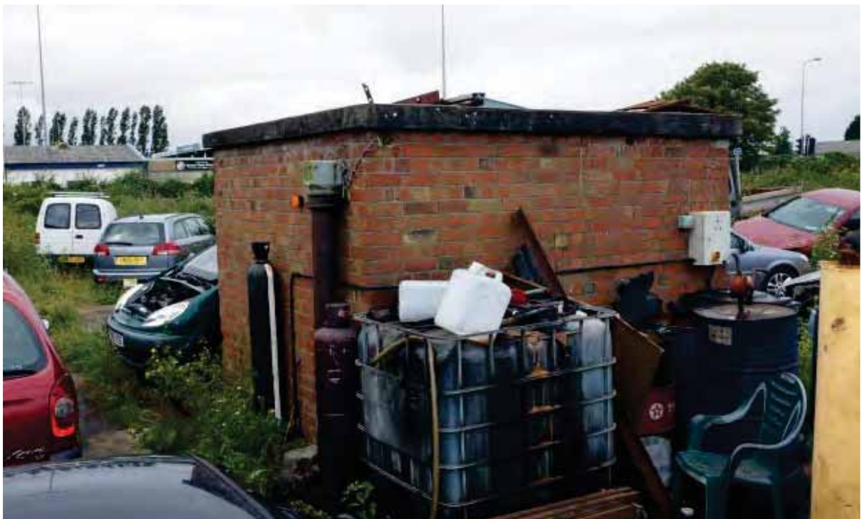
Plate 27: Building 46 – view looking west
