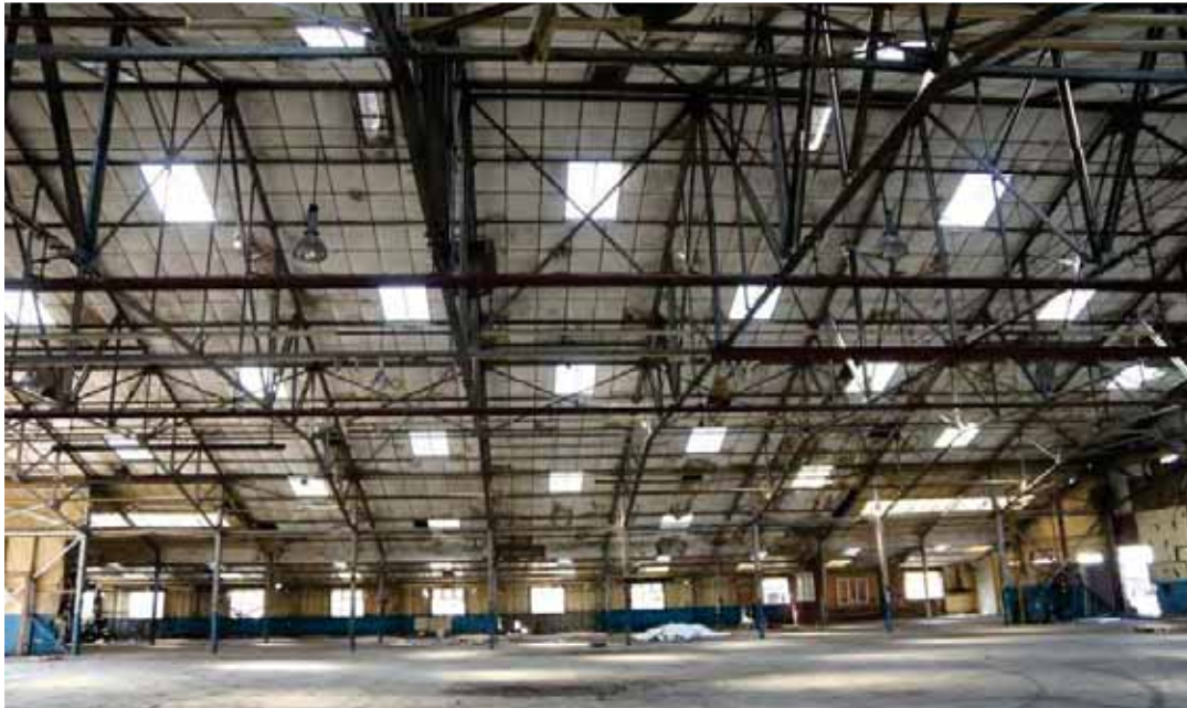
Plate 73: Shop 10 – interior view looking towards the standard annexe
