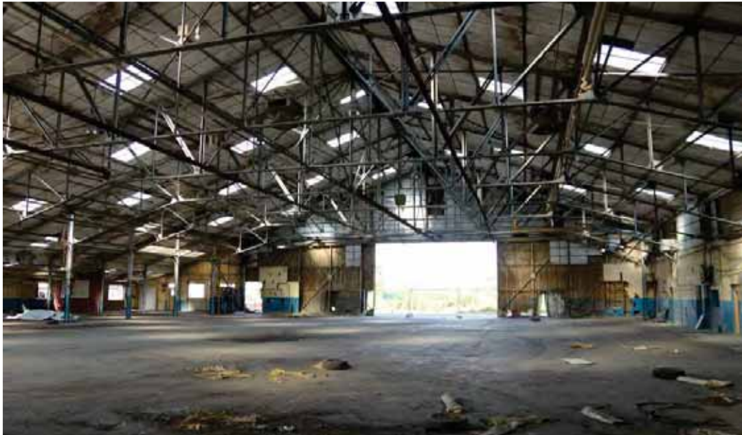
Plate 72: Shop 10 – interior view looking west
