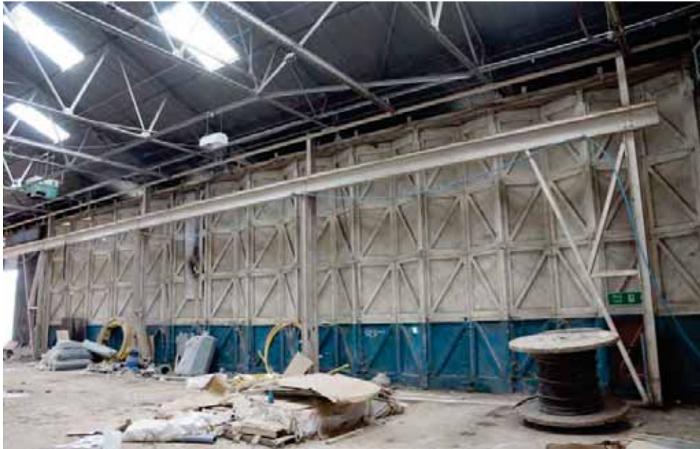
Plate 70: No.3 Flight Shed – interior view of small shop within showing the Esavian doors
