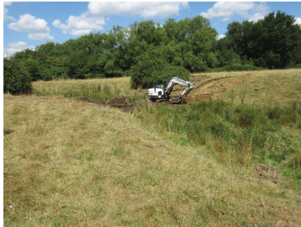
View of trench 1 during backfilling, looking north-west
