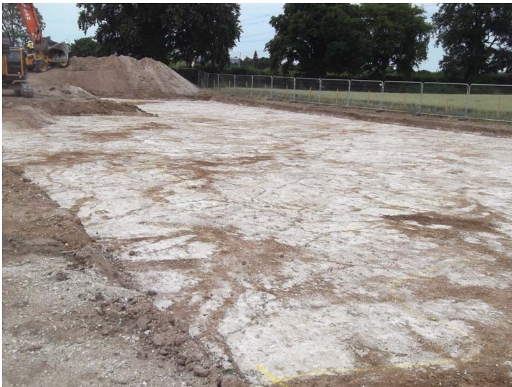
Figure 6: Site, looking north-east
