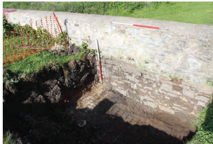
Trench H5, looking south-west (scales 1m)
