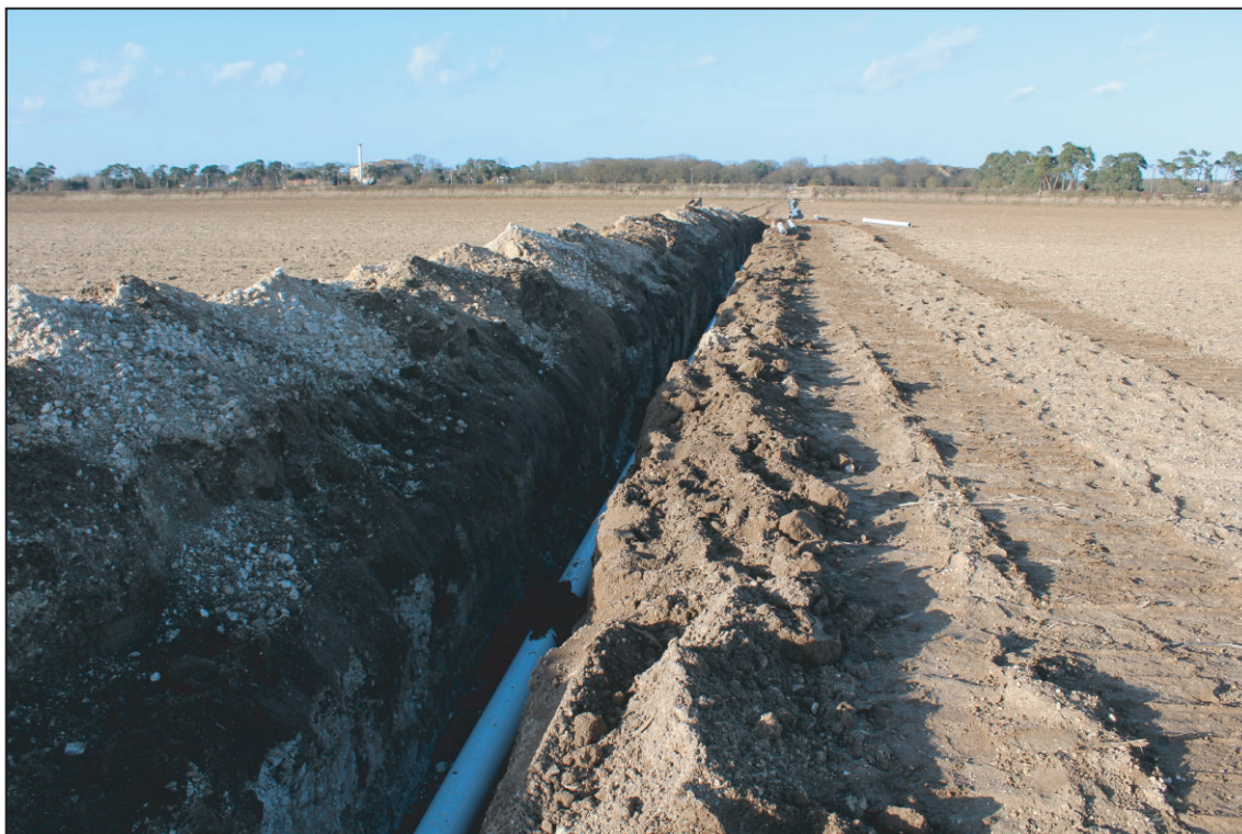
Trench for the pipeline, looking north-west
