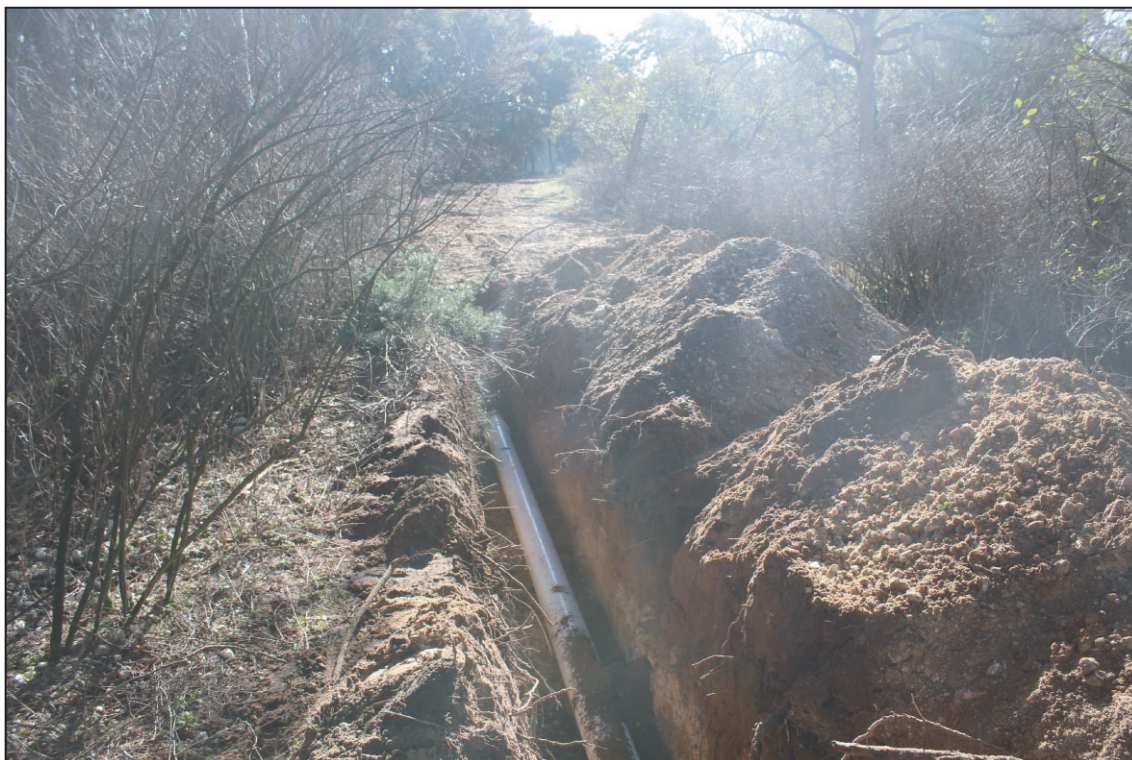
View of pipe and backfill, looking south
