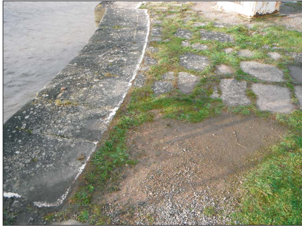
Northern side of Harbour, looking west, before excavation
