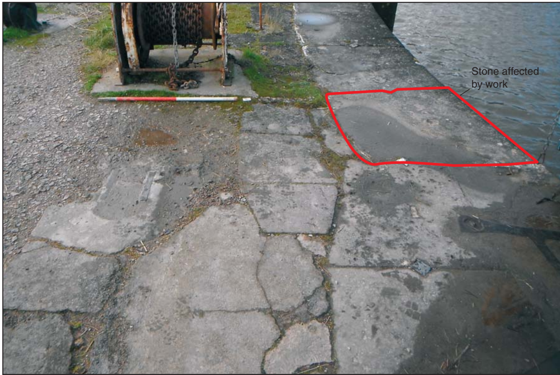
Southern area prior to excavation, looking west (1m scale)
