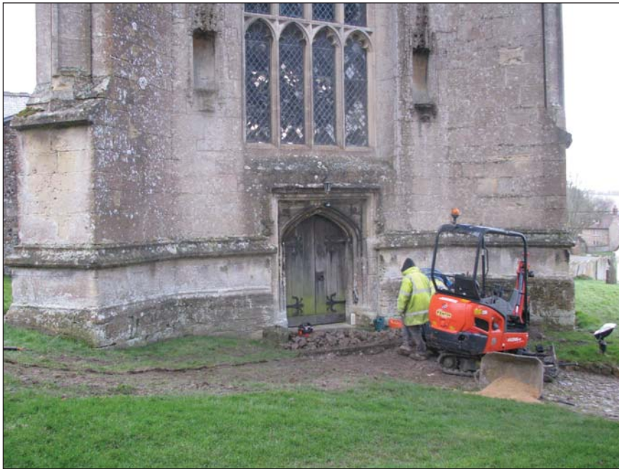
General view south-east of Trench 3
