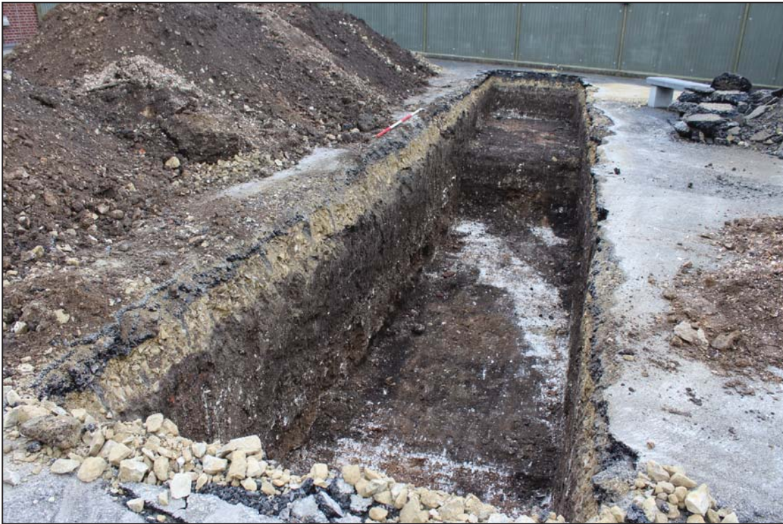
Oblique view of trench 3, looking north (2m scale)
