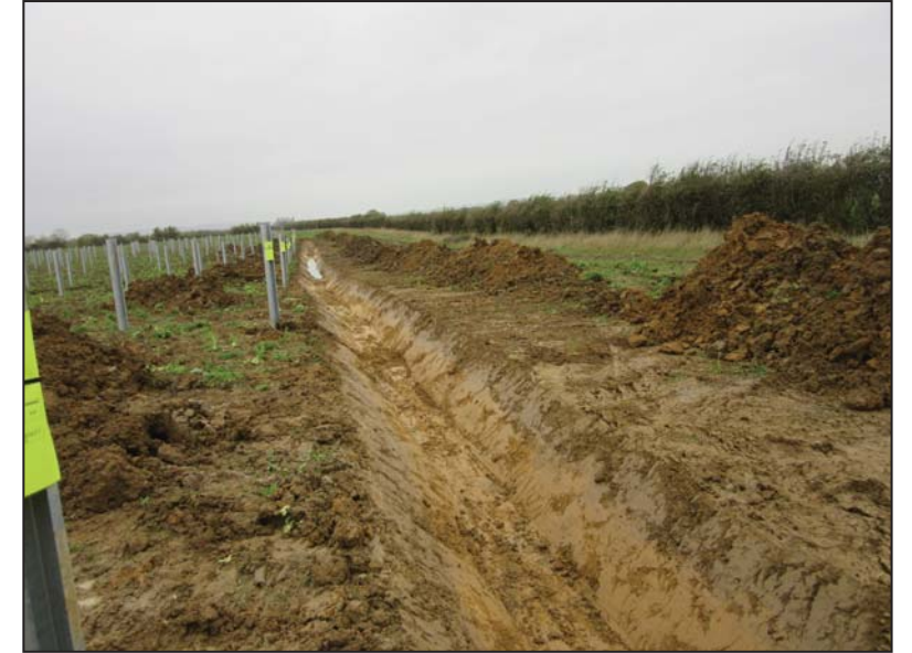
Post-excavation view of Trench 2
