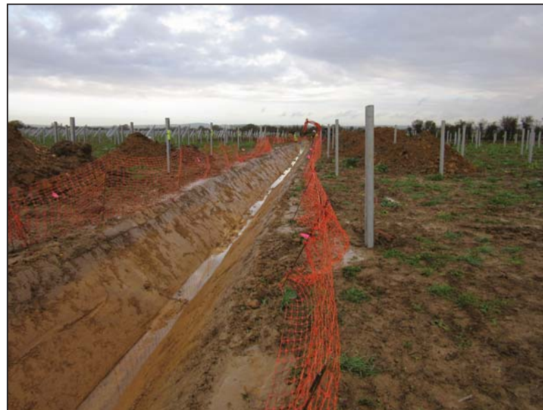
Post-excavation view of Trench 2
