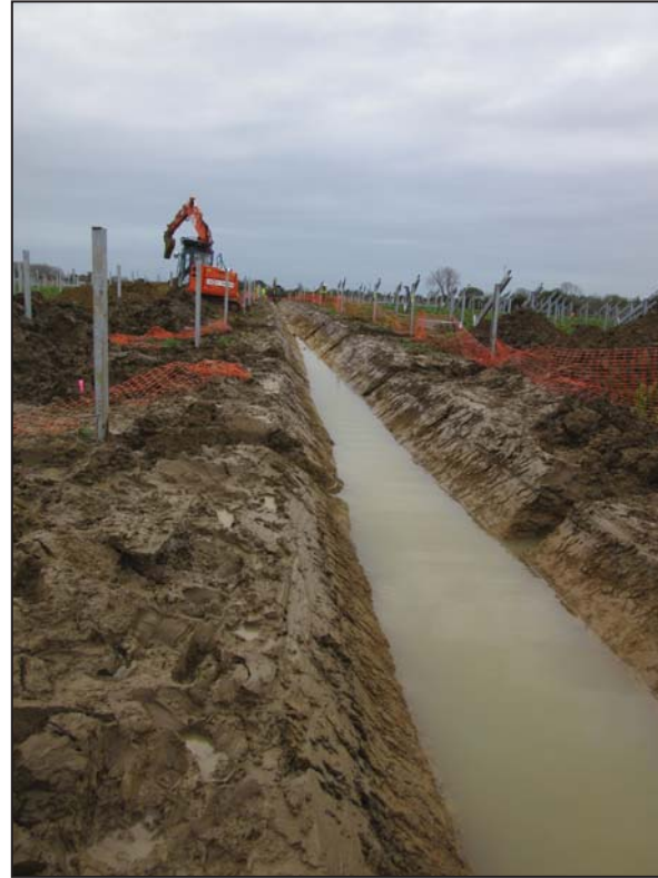
Post-excavation view of Trench 2
