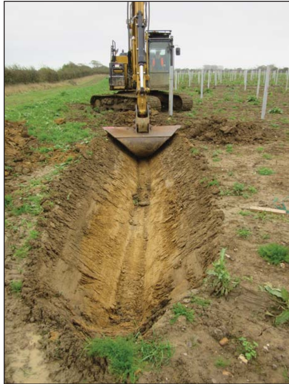
Opening up Trench 2
