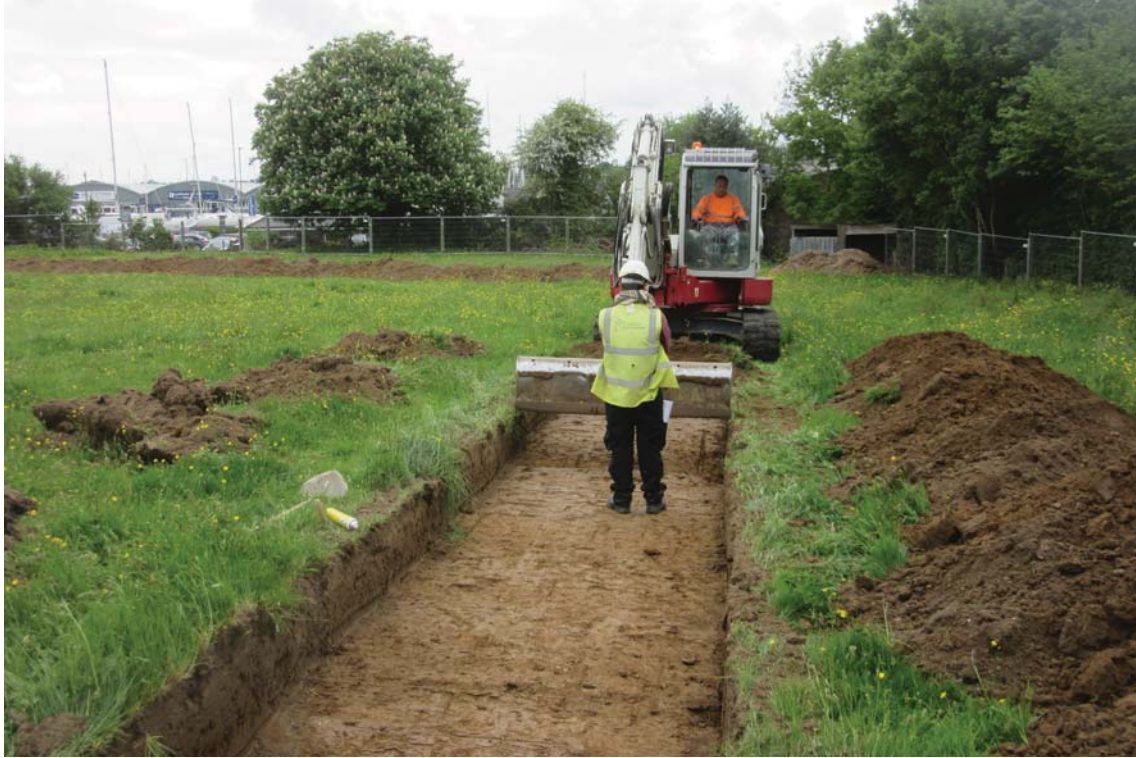
Photograph during work on site
