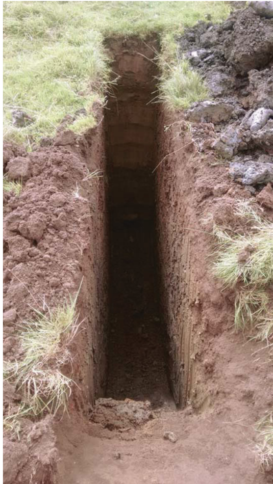
Trial pit 1, looking west
