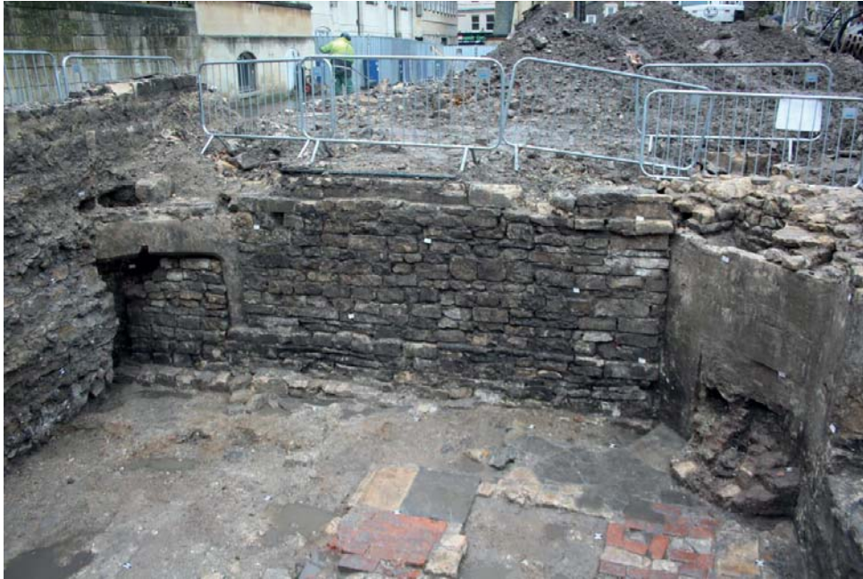
No. 9 Bridewell Lane, showing the two altered fireplaces and the later inserted walls (unrendered), looking south.
