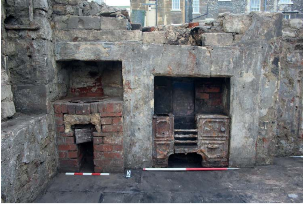
Detail of fireplace and later oven with 'copper' to the southern wall of the front room of 4 Bridewell Lane, looking south (scales 1m and 0.5m).
