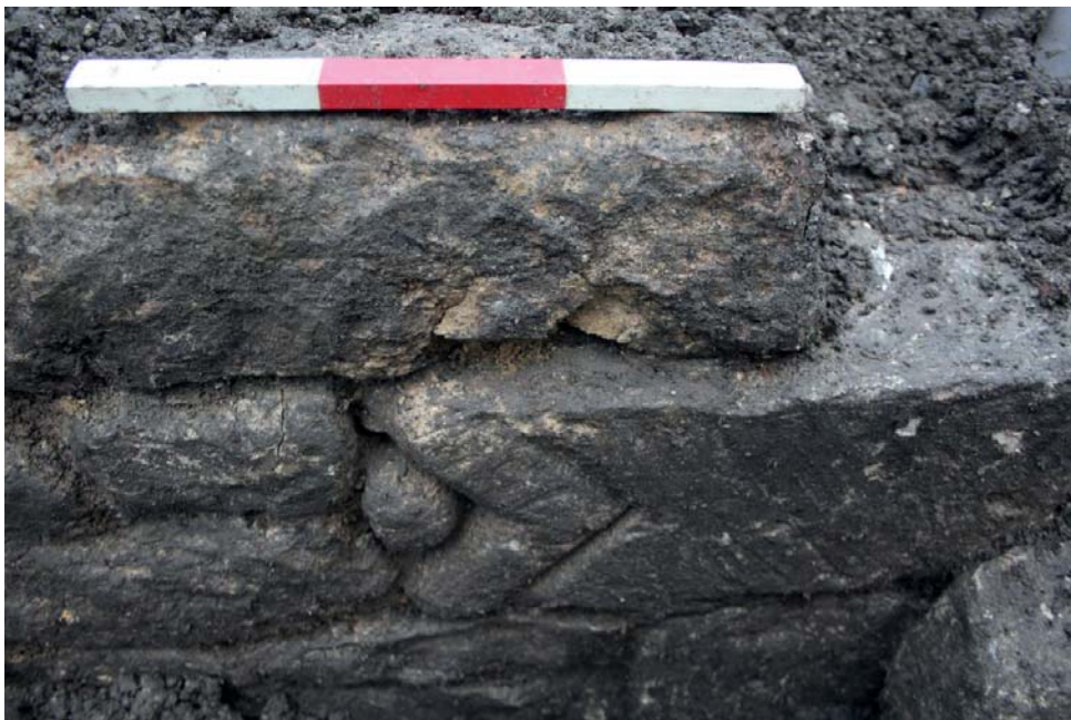
A re-used piece of moulded 16th or 17th century stone set into the rear wall of 9 Bridewell Lane, looking east (scale 0.3m).
