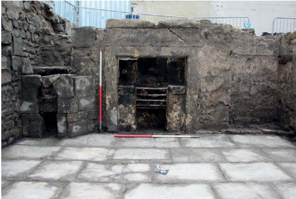
Detail of fireplace and associated later oven structure to the right within the front room of 2 Bridewell Lane, looking south (scales 1m).
