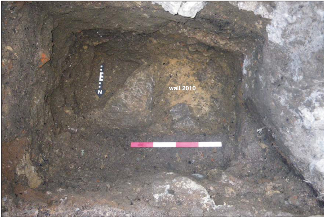
Figure 3: Wall 2010 in base of test-pit for borehole B, looking south (0.4m scale)
