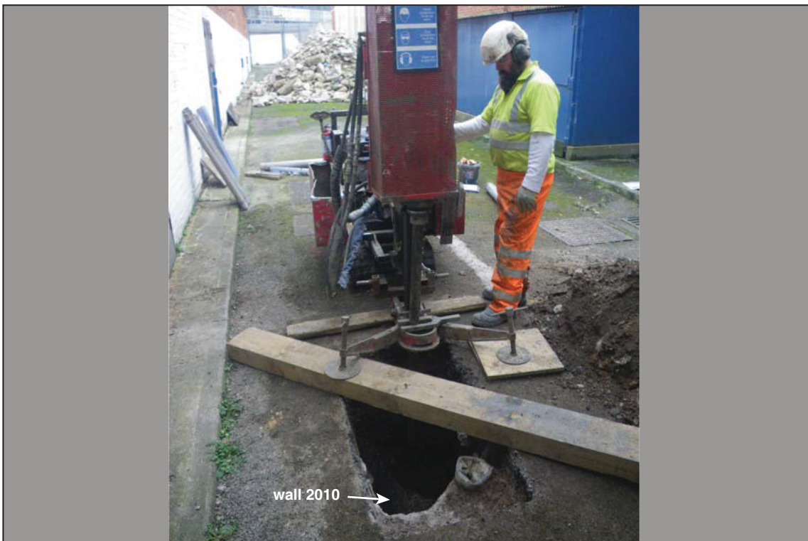
Figure 4: Drilling borehole B adjacent to wall 2010, looking east
