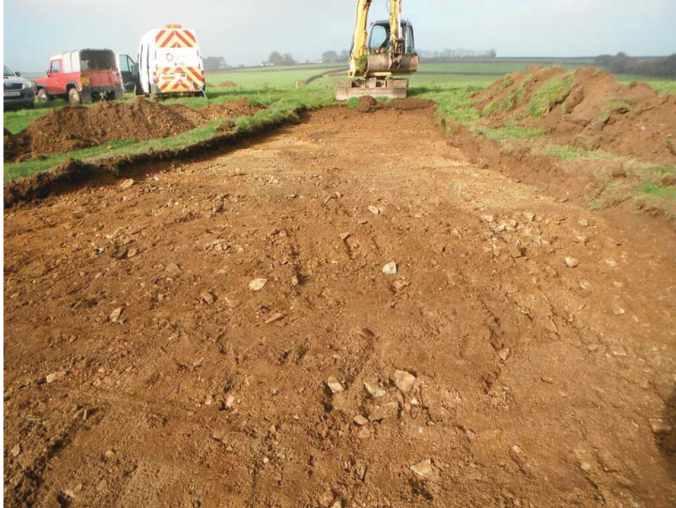
Stripping of Trench 1, looking north-west
