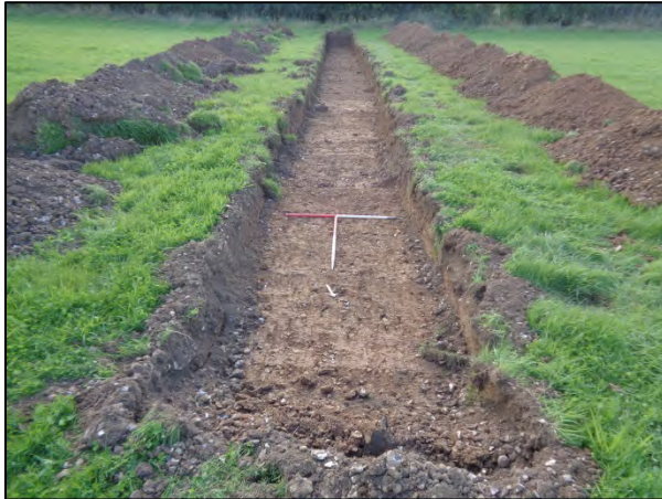
Plate 13: Trench 14 looking south-west (99.08m aOD)
