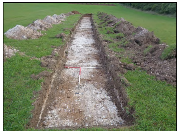
Plate 12: Trench 13 looking east (103.78m aOD)
