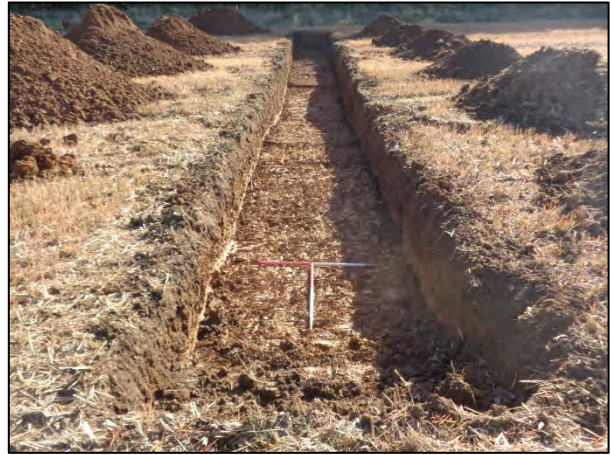
Plate 100: Trench 101 looking east (140.05m aOD)
