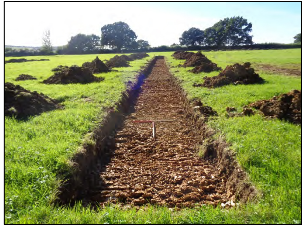
Plate 64: Trench 65 looking south-west (149.98m aOD)
