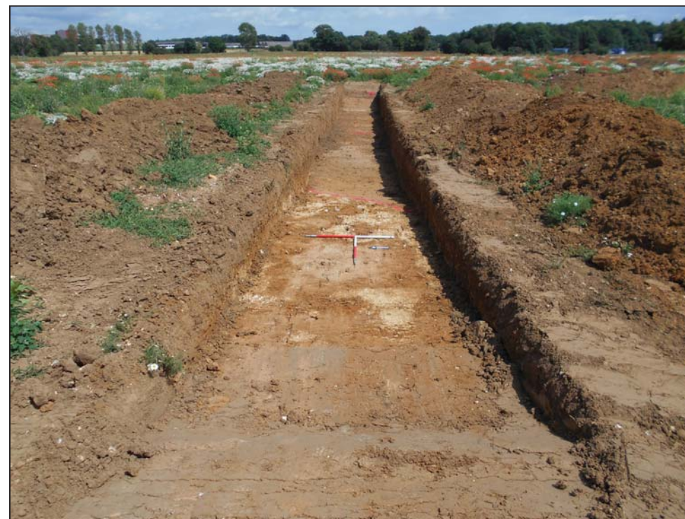
Trench 34, looking east (scales 1m)
