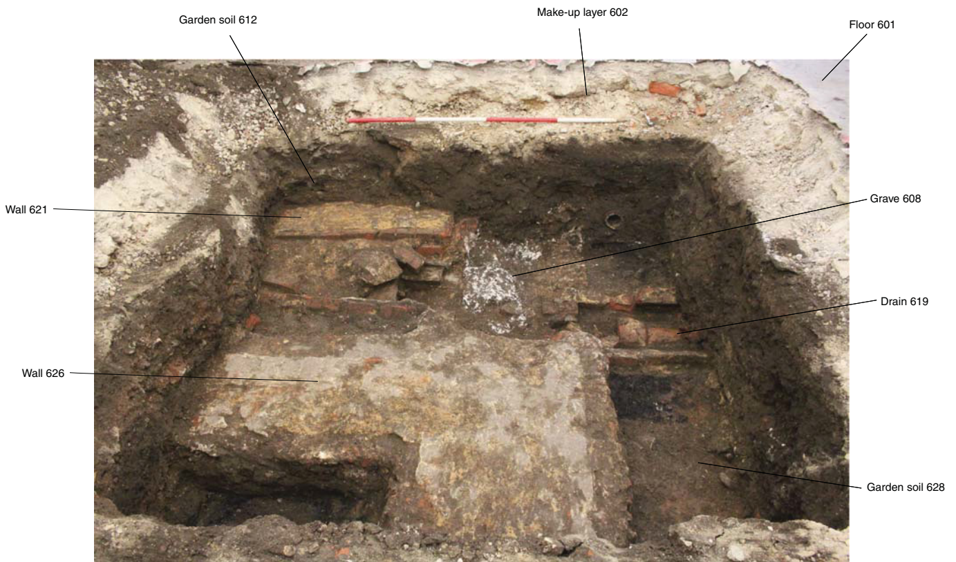
Trench 6, looking south, showing 19th-century walls, culvert and 20th-century grave (2m scale)
