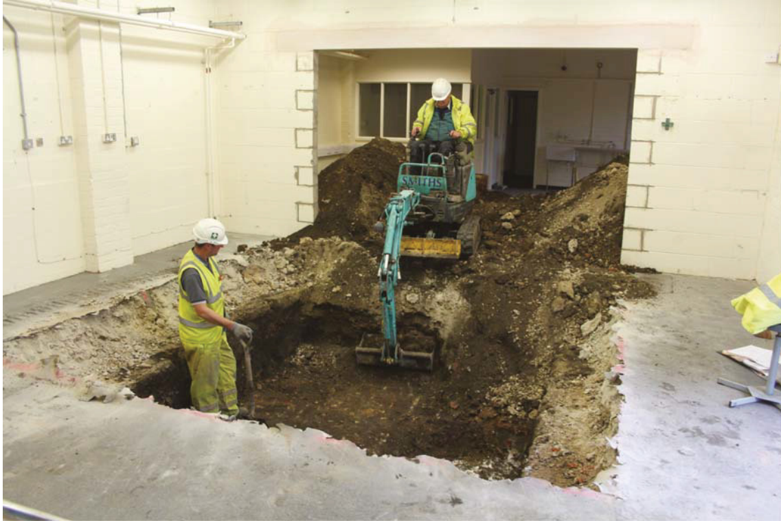
Mechanical excavation of Trench 6, looking east
