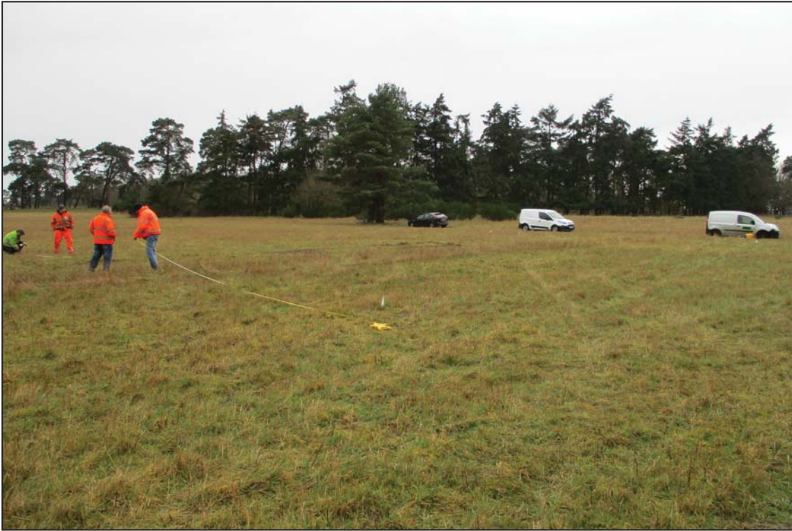
Laying out the site of the infiltration basin, looking north-west
