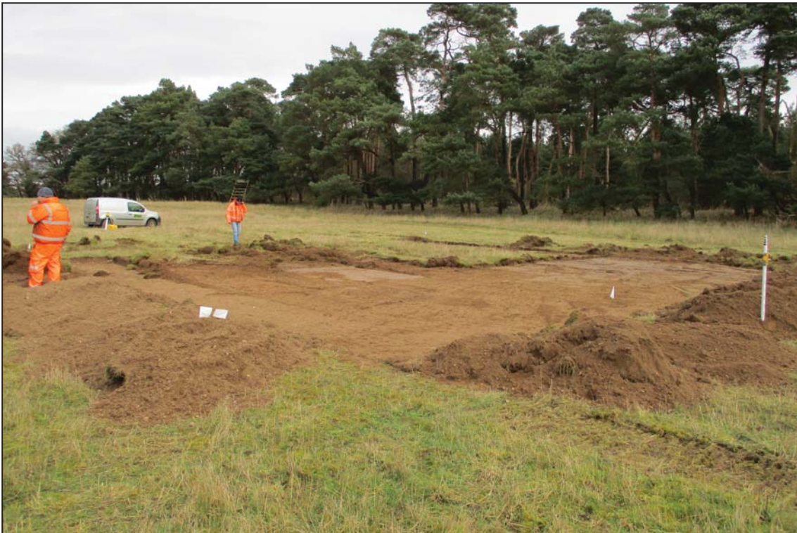
Ground reduction for the infiltration basin, looking north-east
