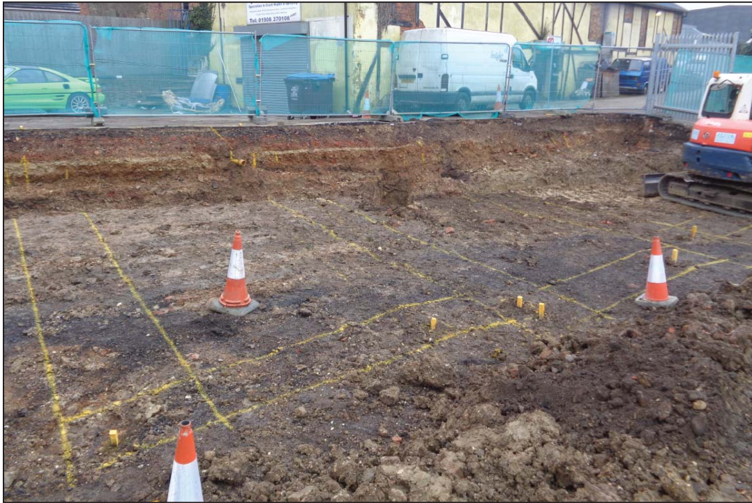
Photograph 1 : working shot looking north-west to modern section
