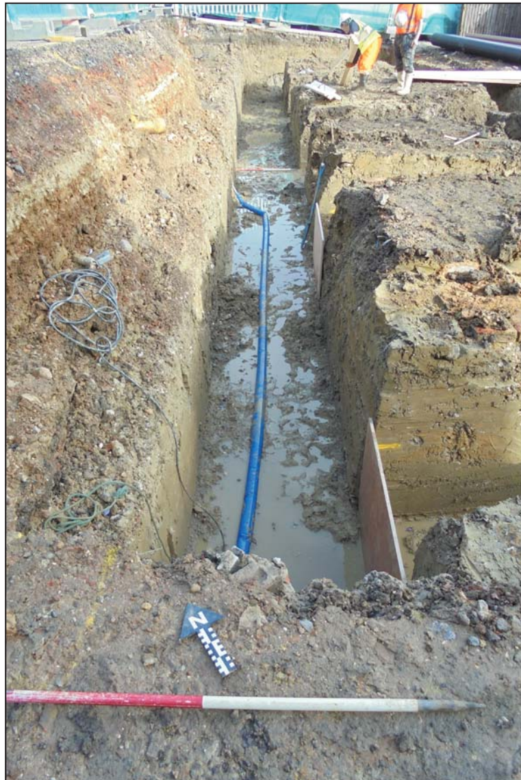
Photograph 3: Western foundation trench, looking north-east (scale 1m)
