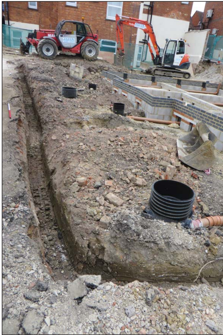
Photograph 5: Service trench excavation, looking south-east (scale 1m)
