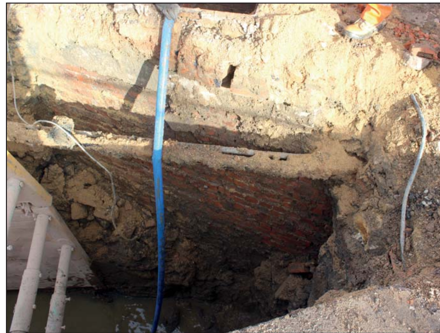
Manhole 3 at southern extent of drainage trench
