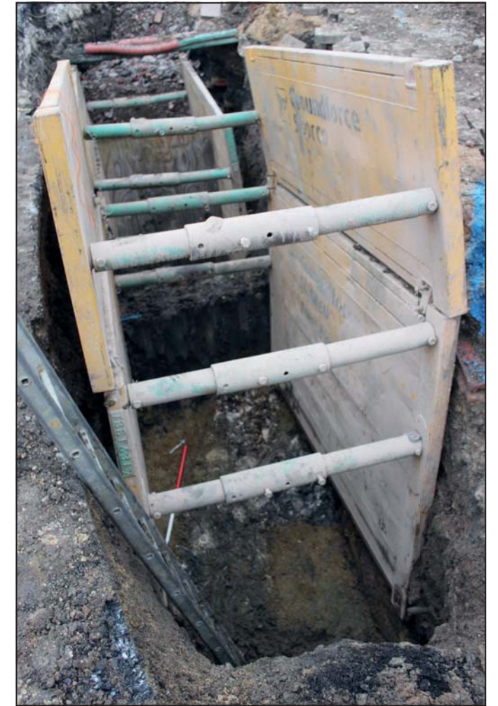
General site photo
