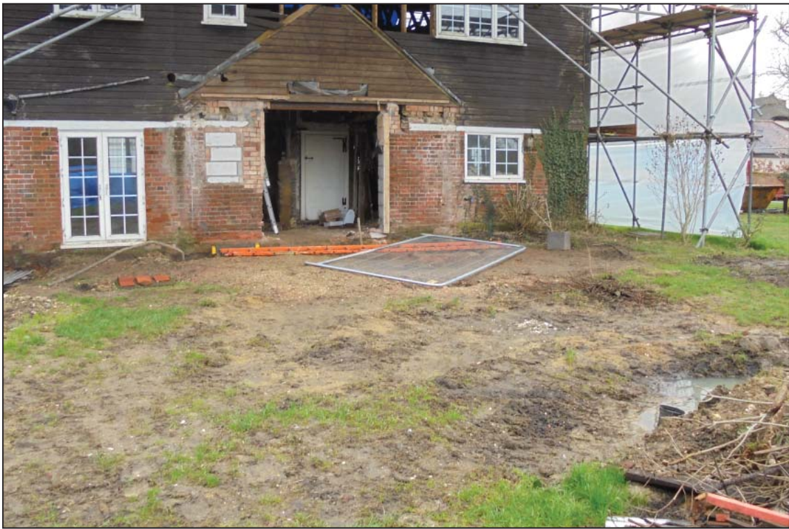
Trench 2 area pre-excitation, looking south-east
