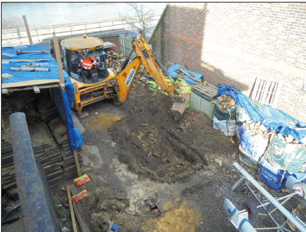
Working shot showing limitations for excavation
