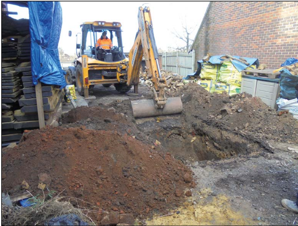
Working shot showing limitations for excavation
