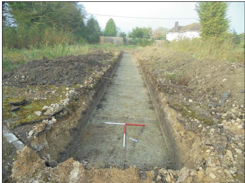
Pre-excavation view south-west across trench 5 (1m scale)
