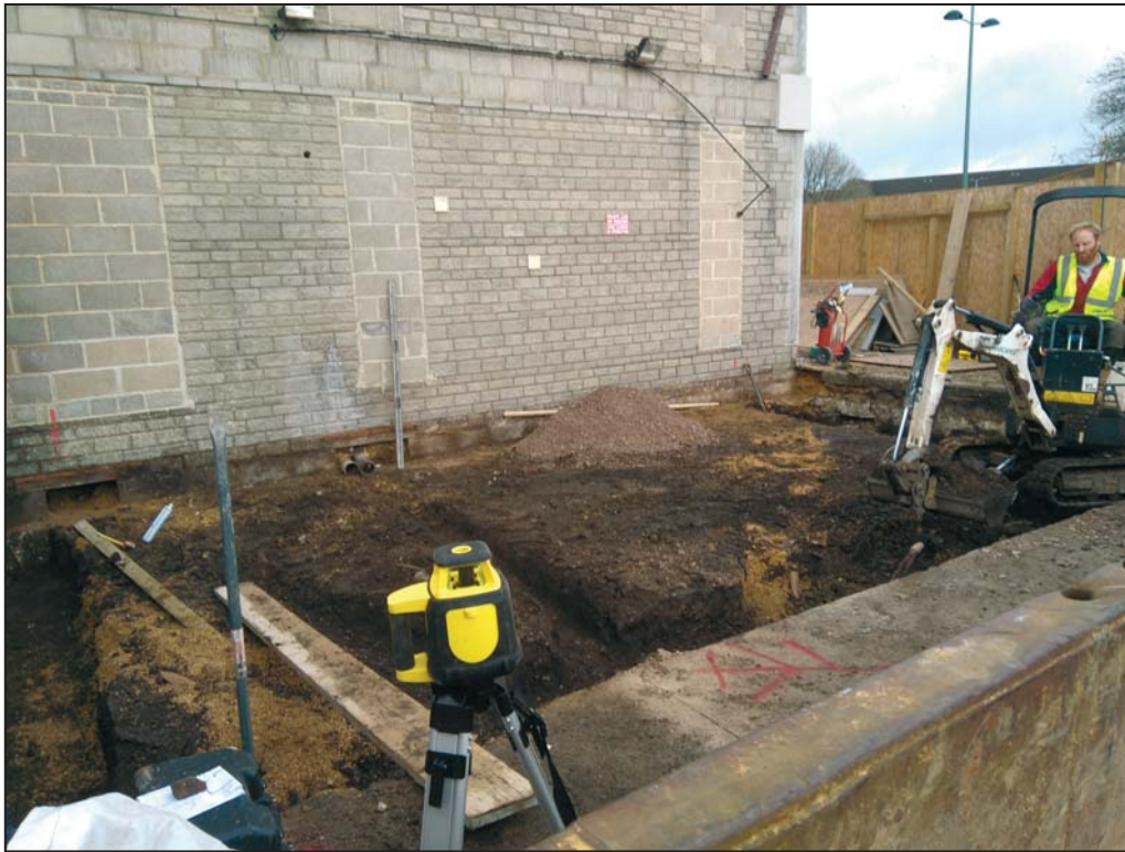
Working shot showing the extent of Trench 3, looking north-east
